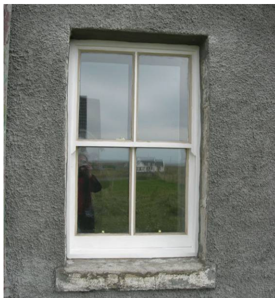
Fig. 5. The new timber double glazed window
