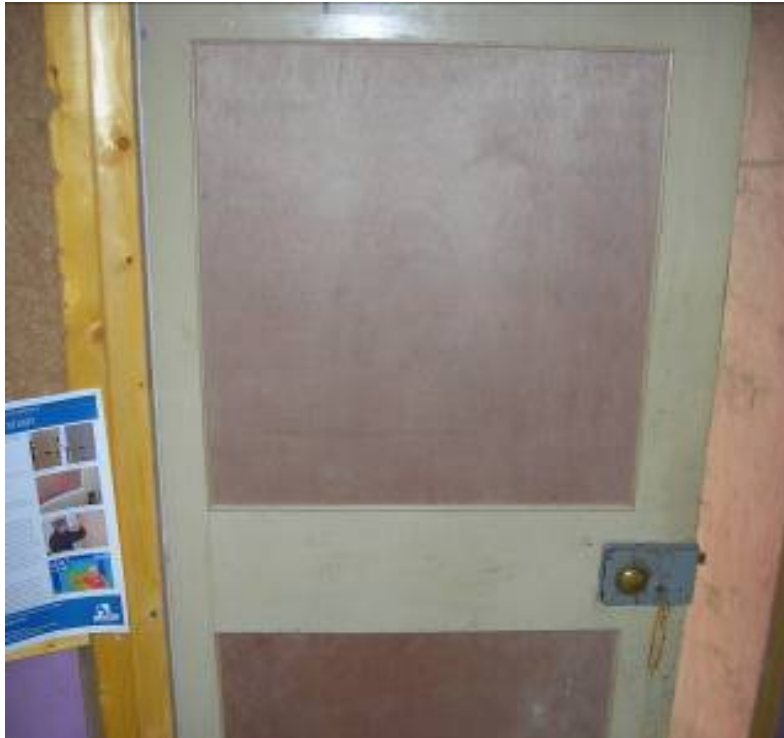
Fig. 7. The insulated door prior to painting
