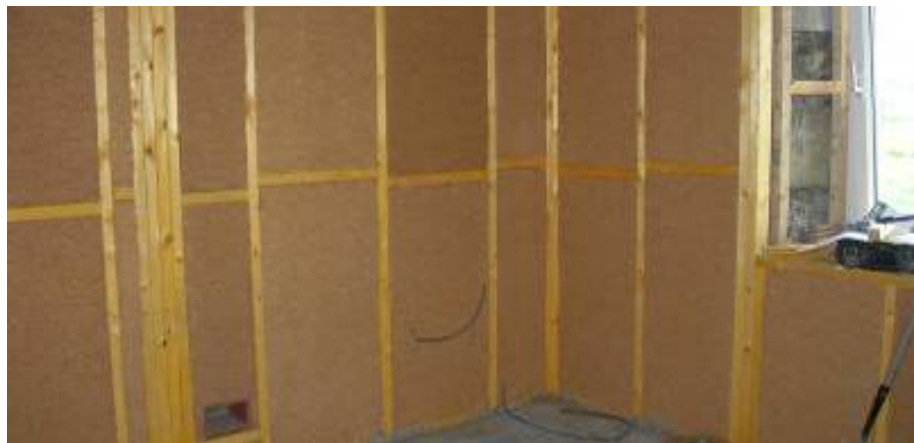
Fig. 2. Wood fibreboard between timber straps prior to application of plasterboard
