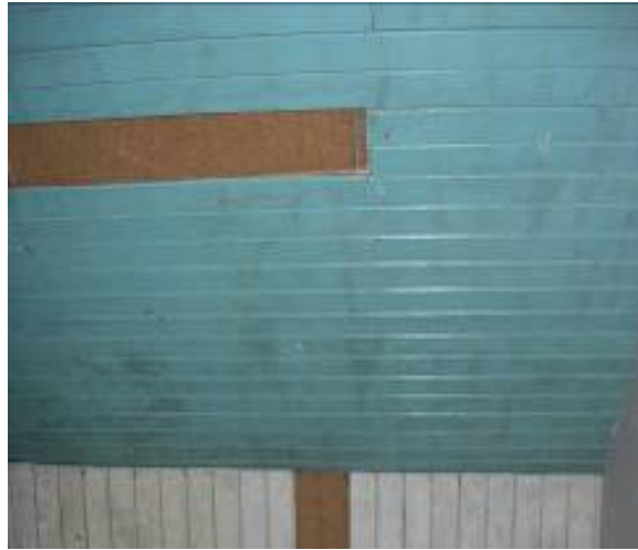
Fig. 4. Wood fibre insulation to the coom, showing re-fixed timber linings
