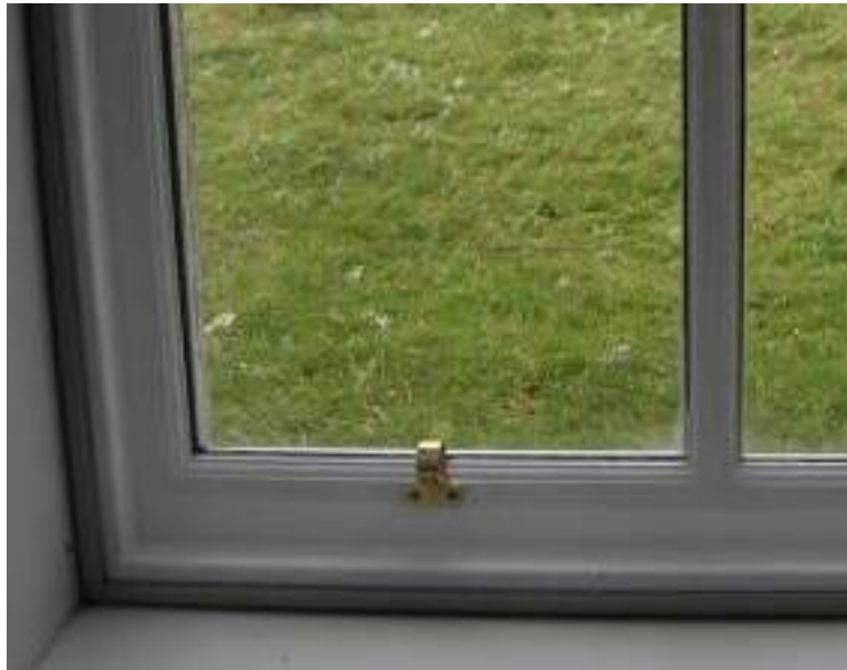
Fig. 6. New double glazed window with polycarbonate secondary glazing in place
