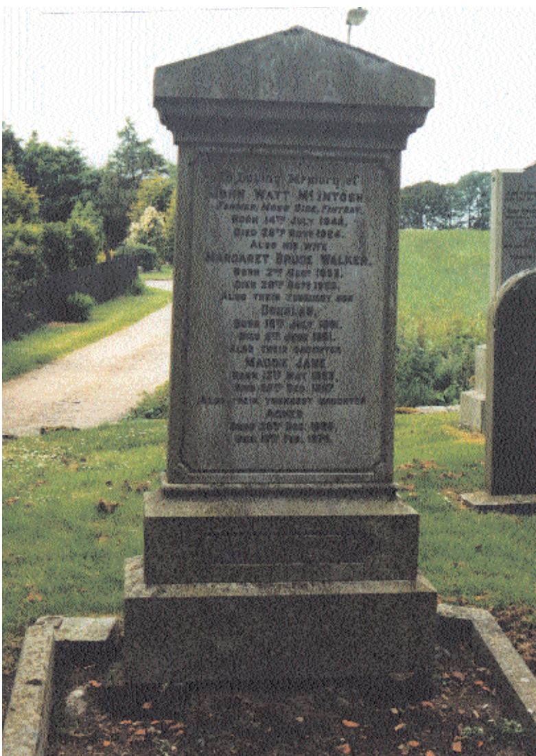
A typical early 20th-century four-piece granite memorial. This memorial is highly unstable and could be toppled easily. The base is balanced on a few loose bricks and the joints between the granite elements are unlikely to be pinned.
