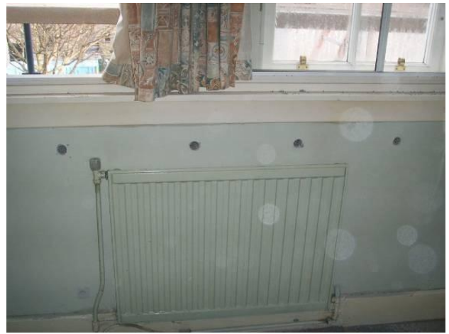
Fig. 19. Drill holes. Image by Adam Dudley Architects
