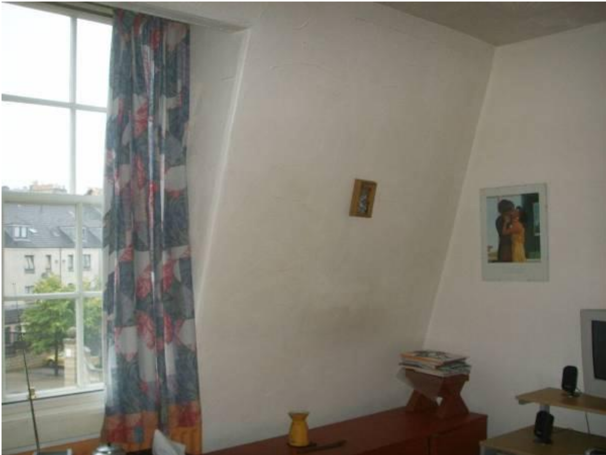
Fig. 4. Mansard roof in the kitchen with finish to walls
