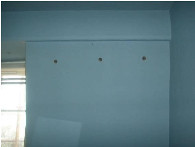
Fig. 18. Drill holes in the bedroom. Image by Adam Dudley Architects
