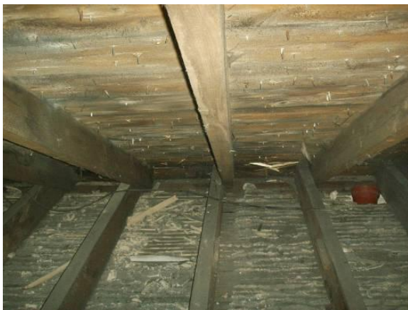
Fig. 12. Existing roof insulation was removed. Image by Adam Dudley Architects
