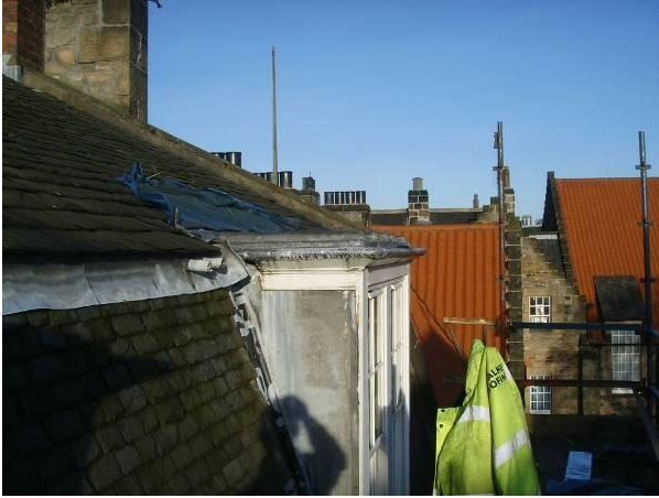
Fig. 5. Lead flat roofed dormer. Image by Adam Dudley Architects
