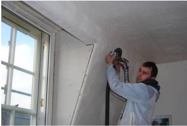
Fig. 16. Bonded polystyrene bead being pumped into the void
