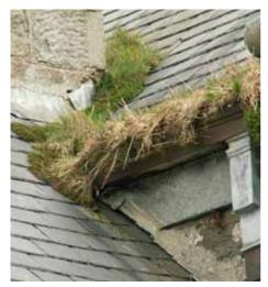
Fig. 5 Guttering clogged by plant growth.
