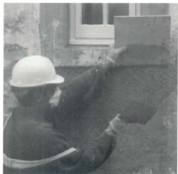
Figure 18 Application of the final (thrown) coat of harl.
