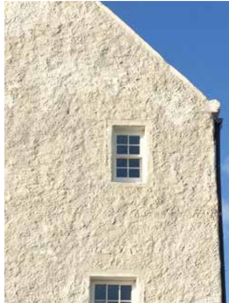
Far left: Resilience of this gable end has been improved by adding additional lead work to skew copes and a hood mould over the window to shed water more effectively from the walls
