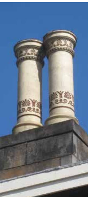
Below: Terracotta chimney pots at Moray Place, Glasgow, conserved by Glasgow City Heritage Trust
