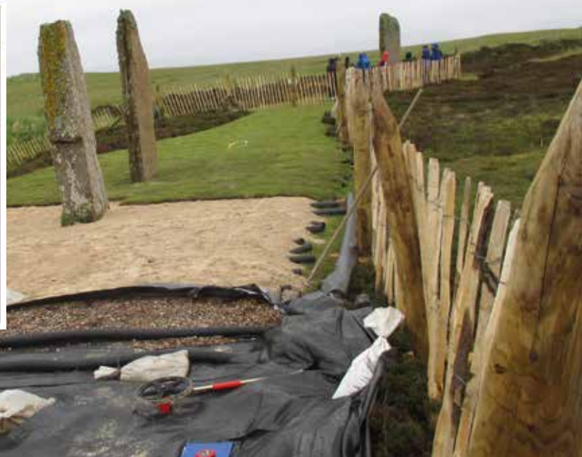
Above: Installing a drainage layer to the path
