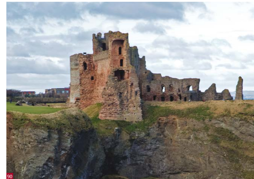
Fig. 90 Coastal erosion at Tantallon Castle, North Berwick.
