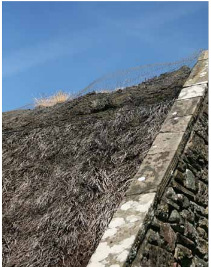
The Ale House – South Ayrshire
