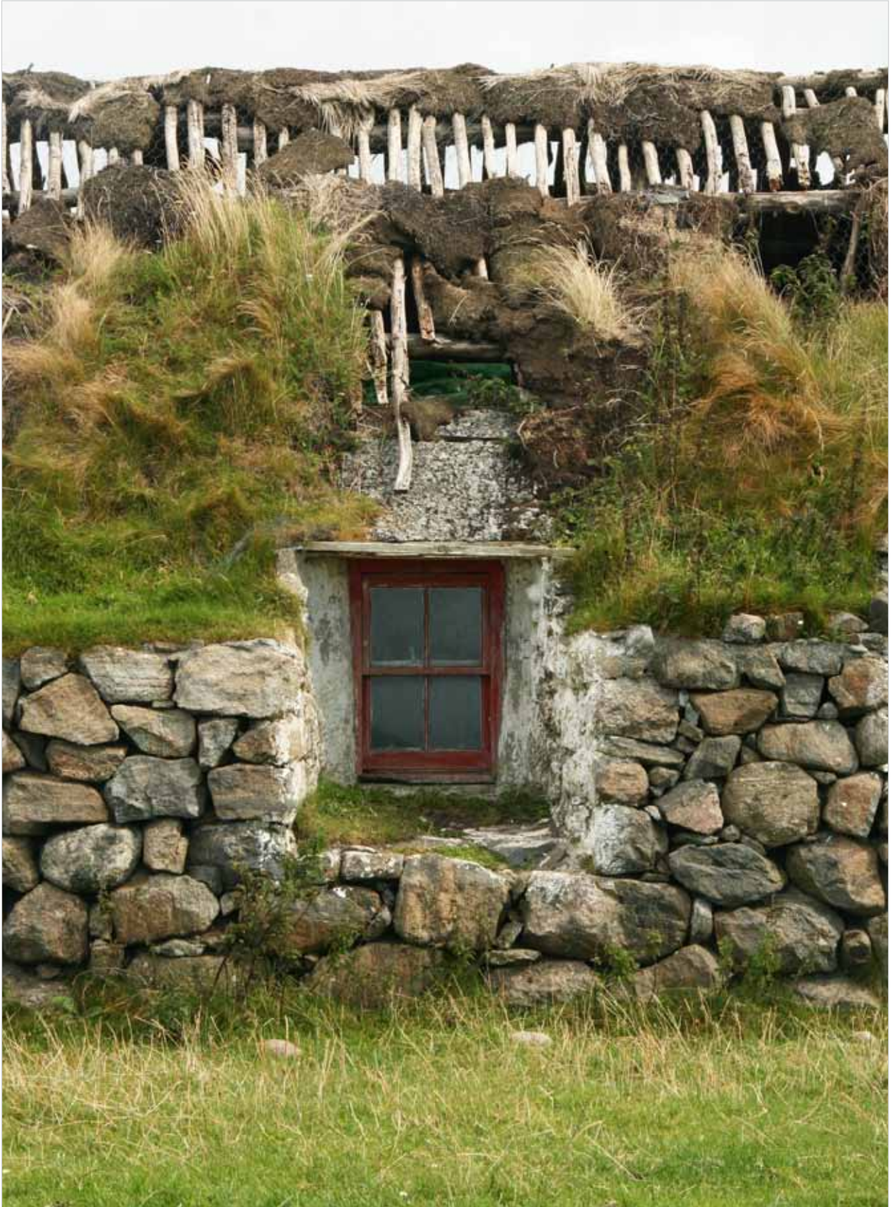
The Terrace (North Cottage) – Argyll & Bute
