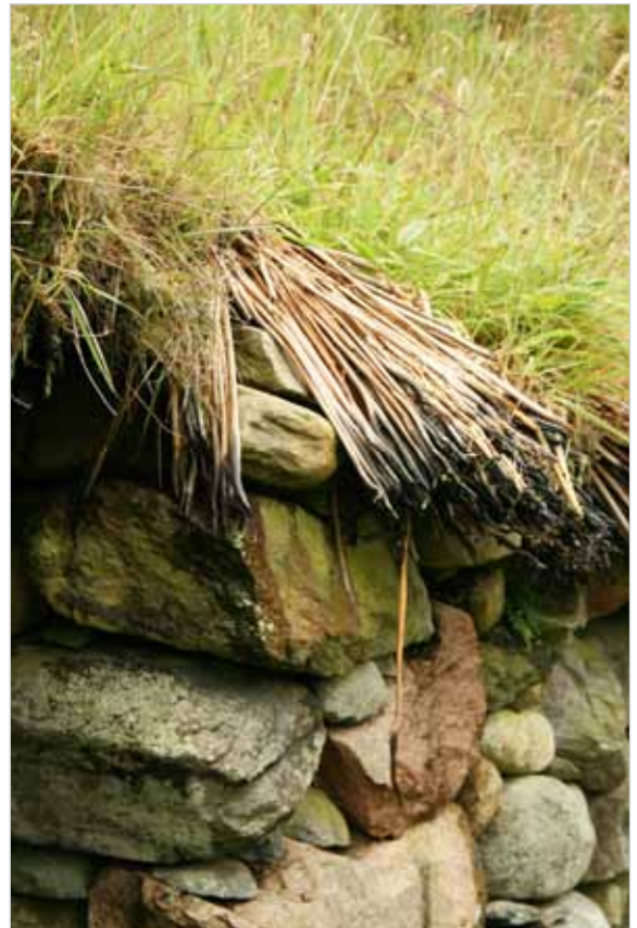
Building G – Argyll & Bute
