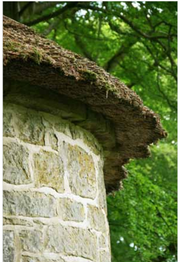
Rustick Hut – Midlothian
