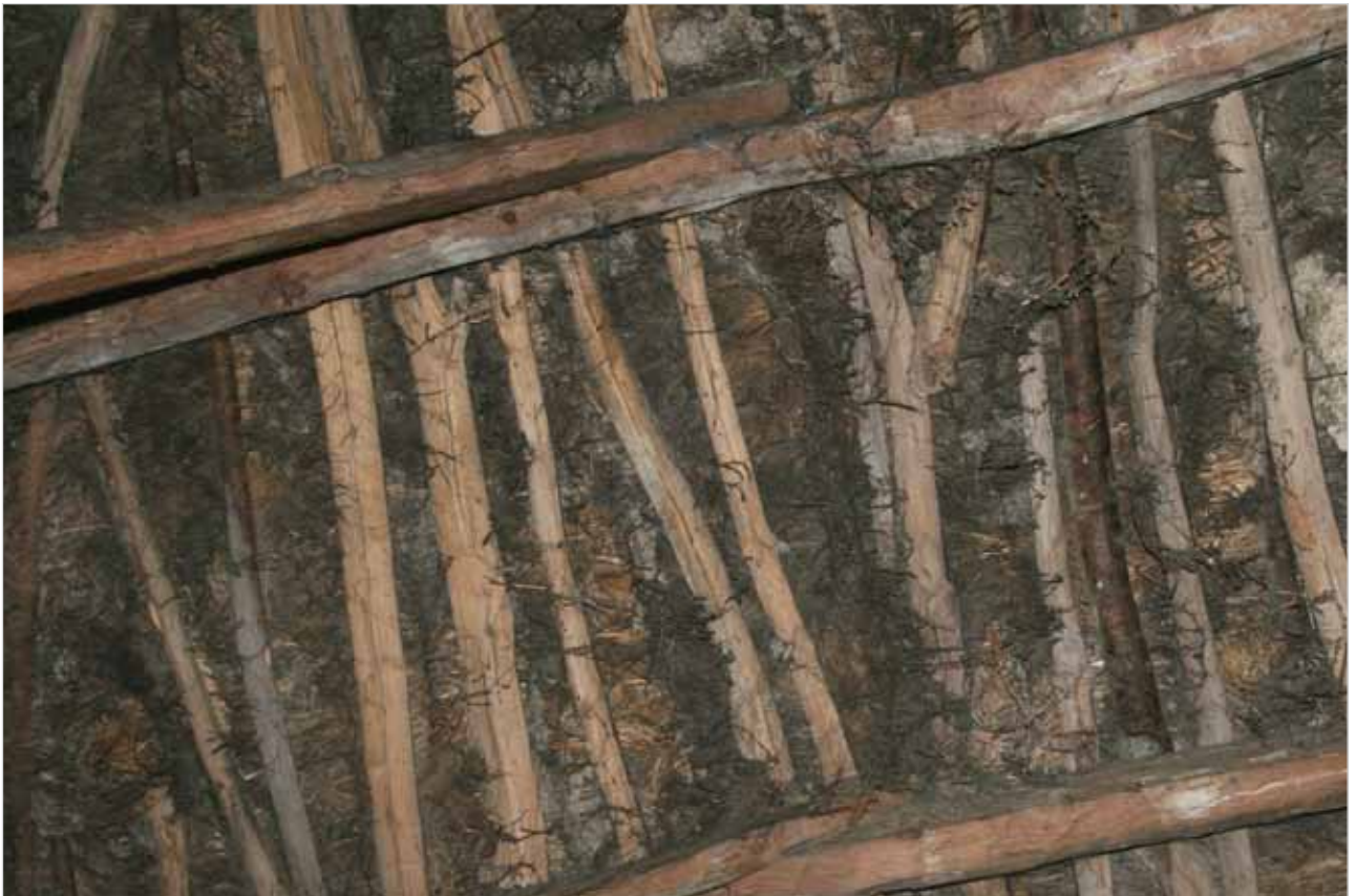
Birkfield Cottage – South Lanarkshire
