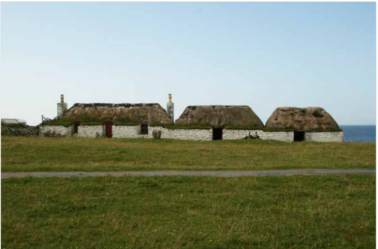
The Terrace (North Cottage) – Argyll & Bute
