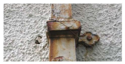
Misalignment of components – The misalignment of components, such as broken sections of drainpipes or gutters, eliminates their effectiveness. This can be caused where fixings or holder-batts (collars that are fixed to the wall on either side of the drainpipe to secure it in place) have not been maintained and have become loose. Where supporting gutter brackets or rhone hooks have been lost, they should be replaced before the gutter sections become dislodged and damaged.
