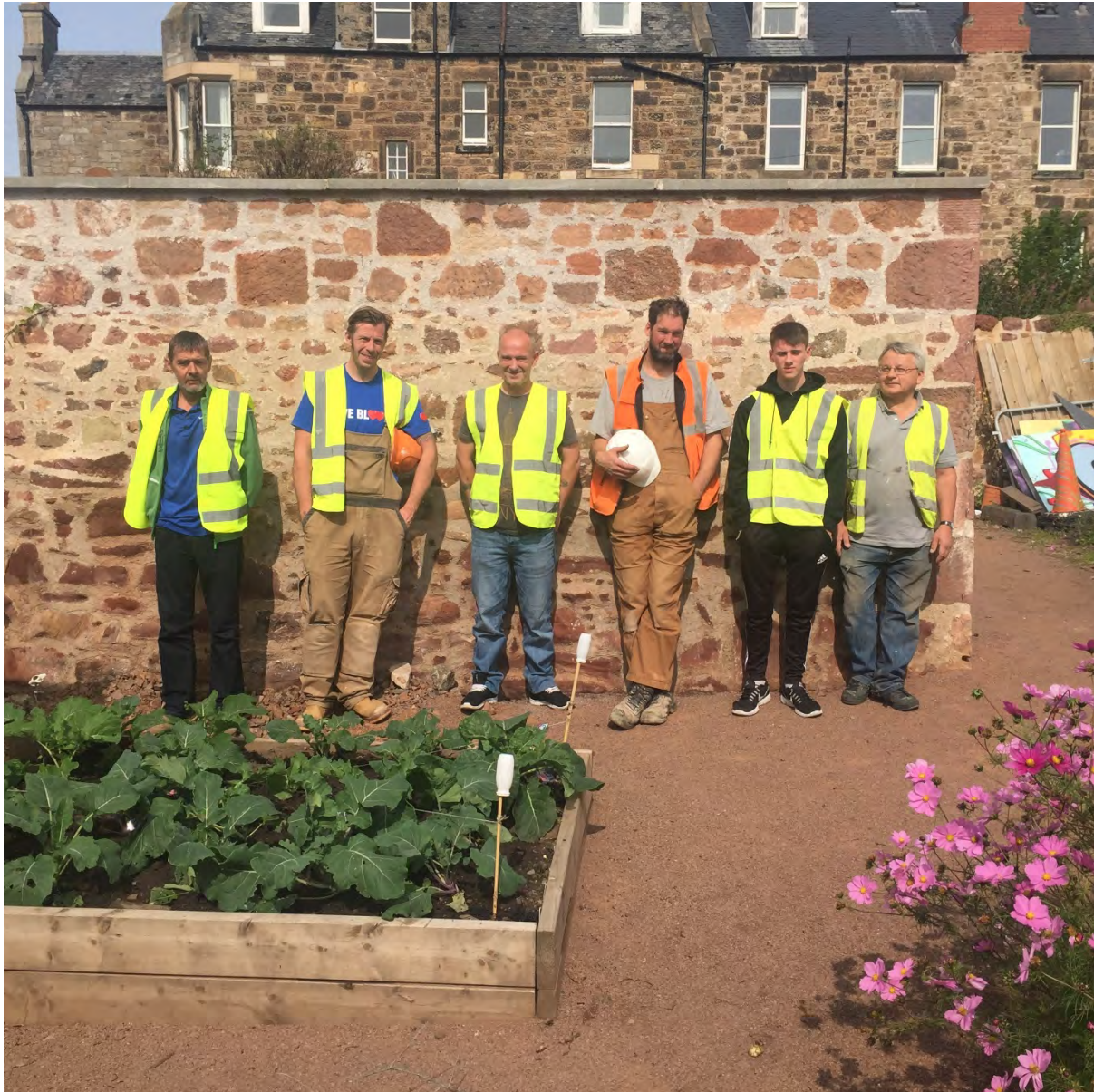
Figure 10. The contractors and volunteers by the Phase 2 finished wall on 9 August 2017.
