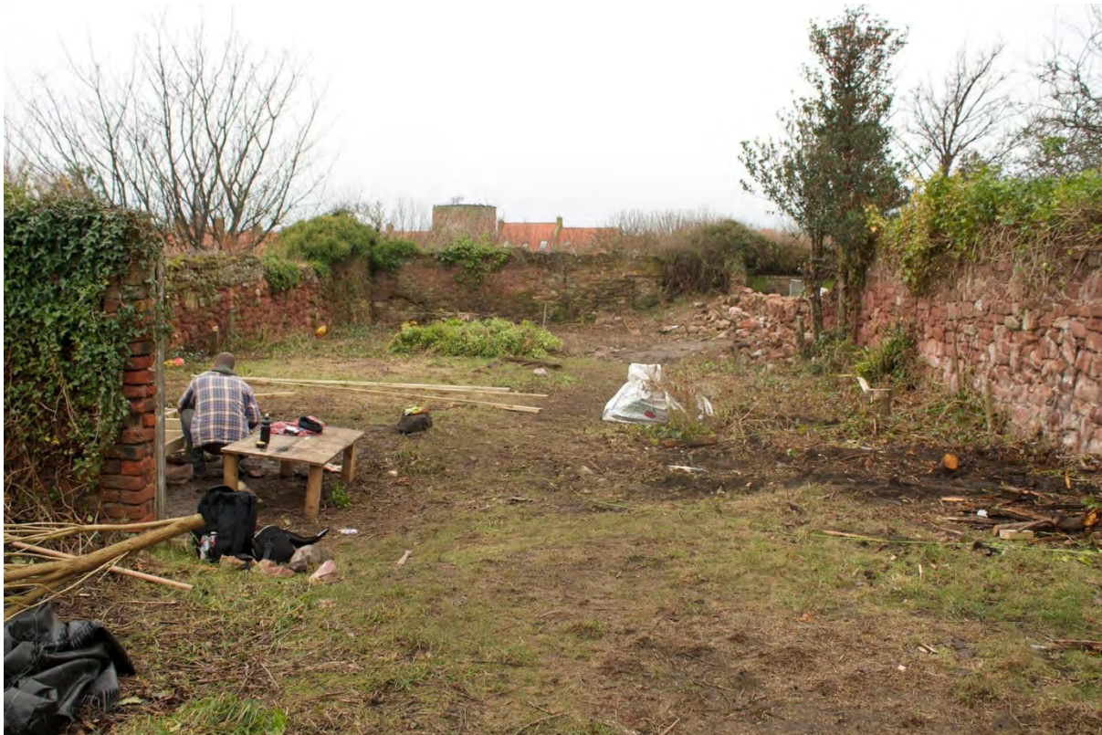
Figure 3. View of the garden plot and the boundary wall before the works. Phase 1 started with rebuilding the collapsed section on the far right.
