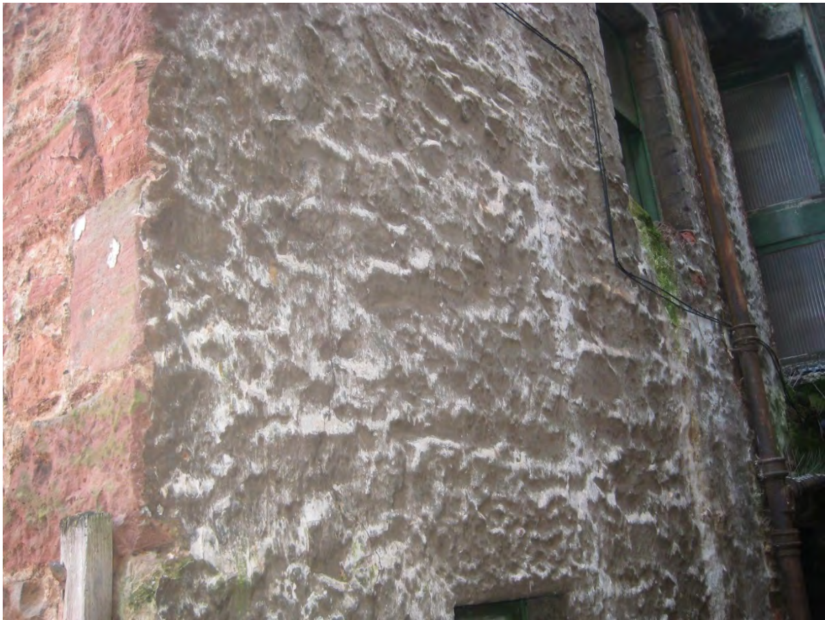
Figure 2. Surviving historic harling finished with limewash in Black Bull Close, Dunbar.
