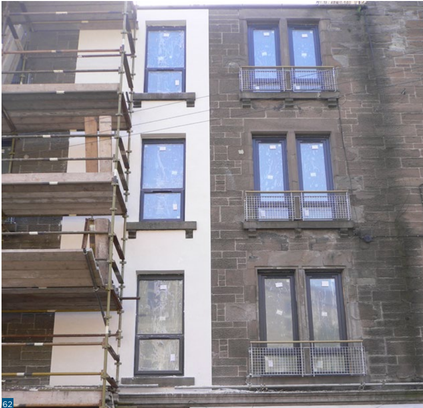
Figure 62: The visual impact of external insulation.
