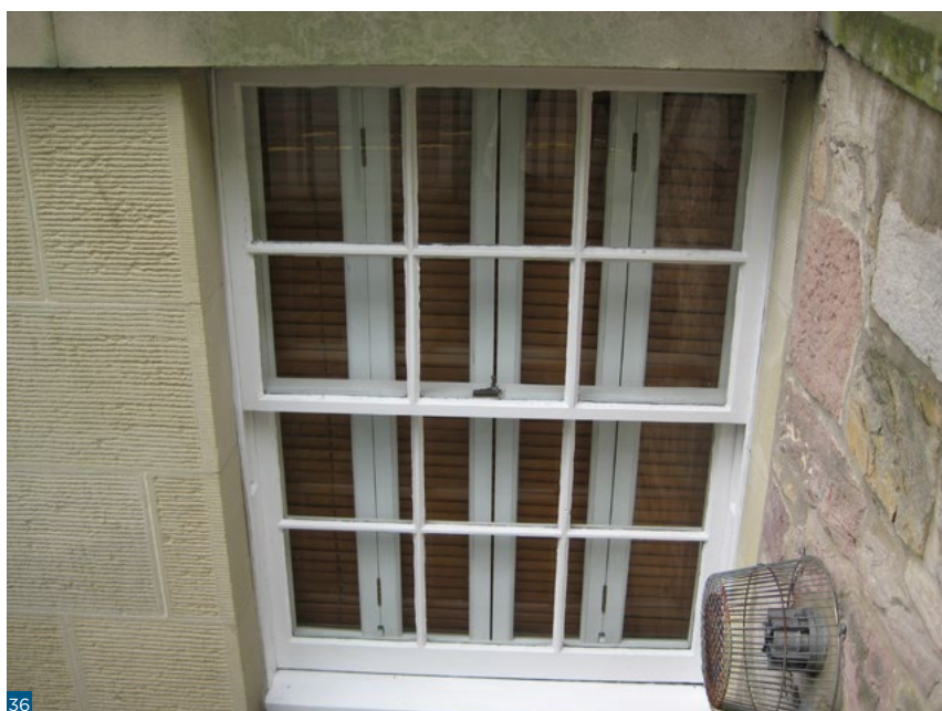
Figure 36: Glazed shutters in use.
