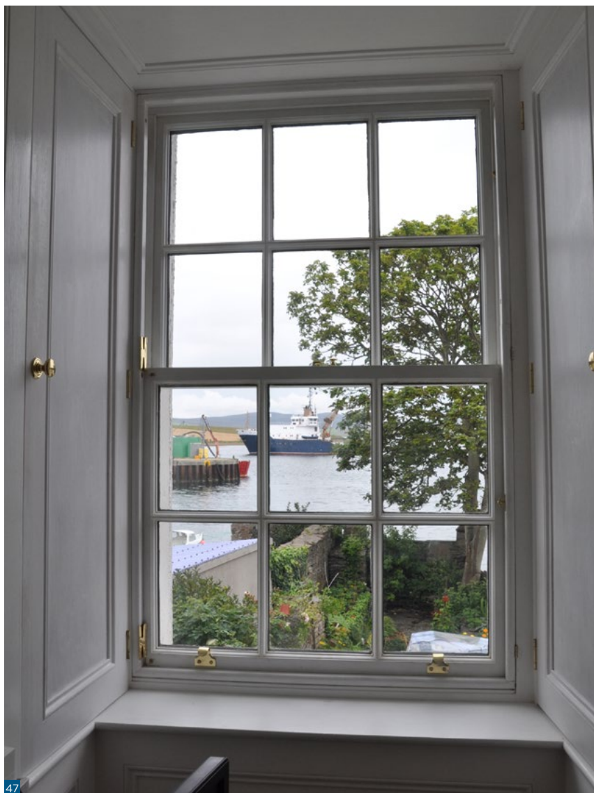
Figure 47: A new sash and case window in a Category B-listed window in Stromness. Note the new working shutters.
