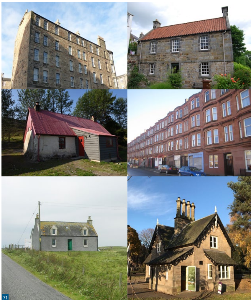
Figure 71: A range of buildings which have been retrofitted as part of Historic Environment Scotland's technical research work. Several are listed and they have all had significant work carried out. Here, they are shown in their post-retrofit state.
