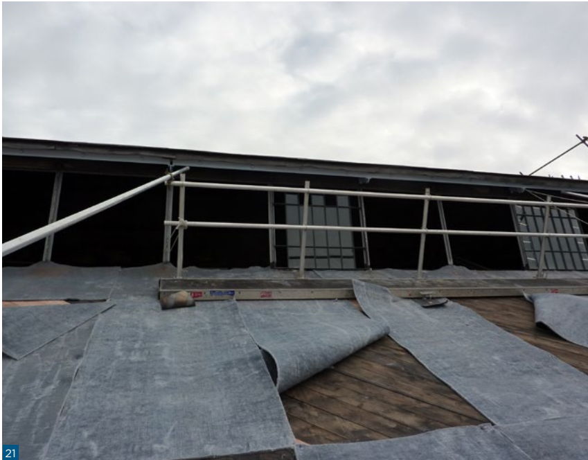
Figure 21: An aerogel insulation blanket laid on top of the sarking.
