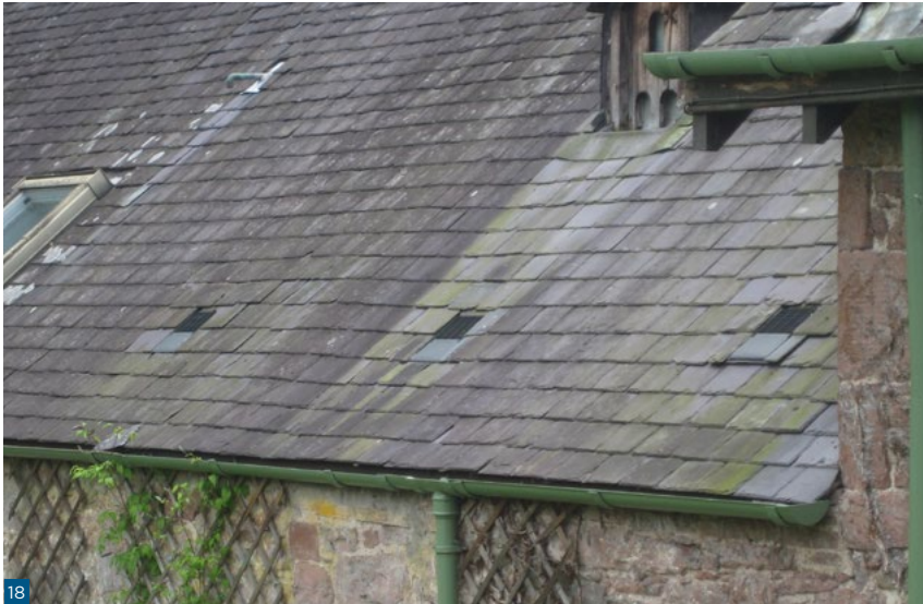
Figure 18: Low-profile roof vents on a slate roof following an upgrade to the roof space.
