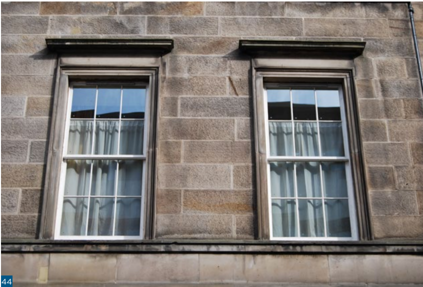
Figure 44: Vacuum panes were trialled at Archibald Place, Edinburgh, in 2009.
