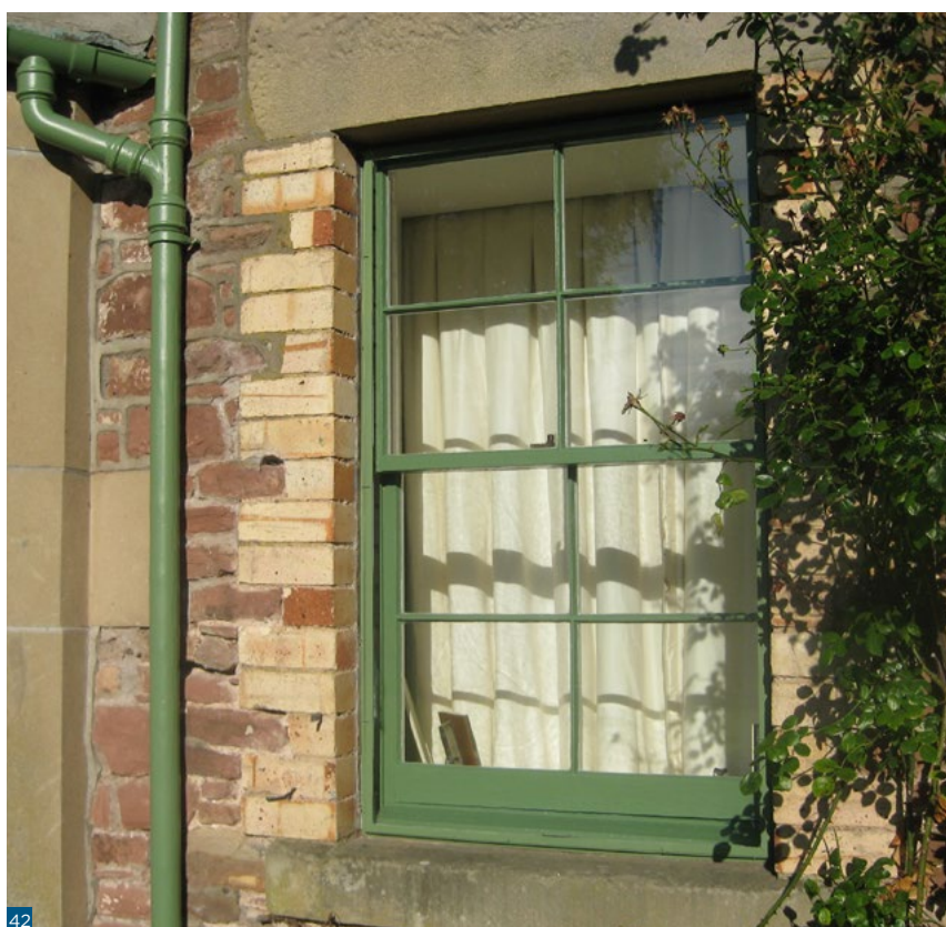
Figure 42: External secondary glazing which gives weathering protection, as well as a degree of thermal improvement.
