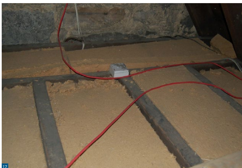
Figure 17: Wood fibreboard laid between ceiling joists.
