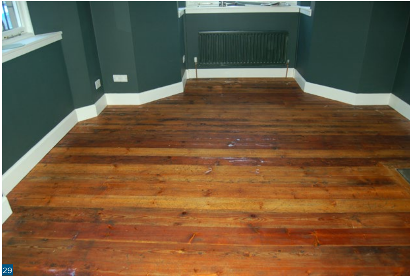
Figure 29: A relaid floor can be finished to a high standard.
