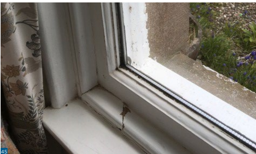
Figure 45: A standard dimension double glazed unit fitted into an existing sash.
