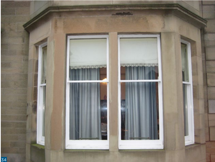
Figure 34: Traditional pattern roller blinds can help reduce heat loss through a window.
