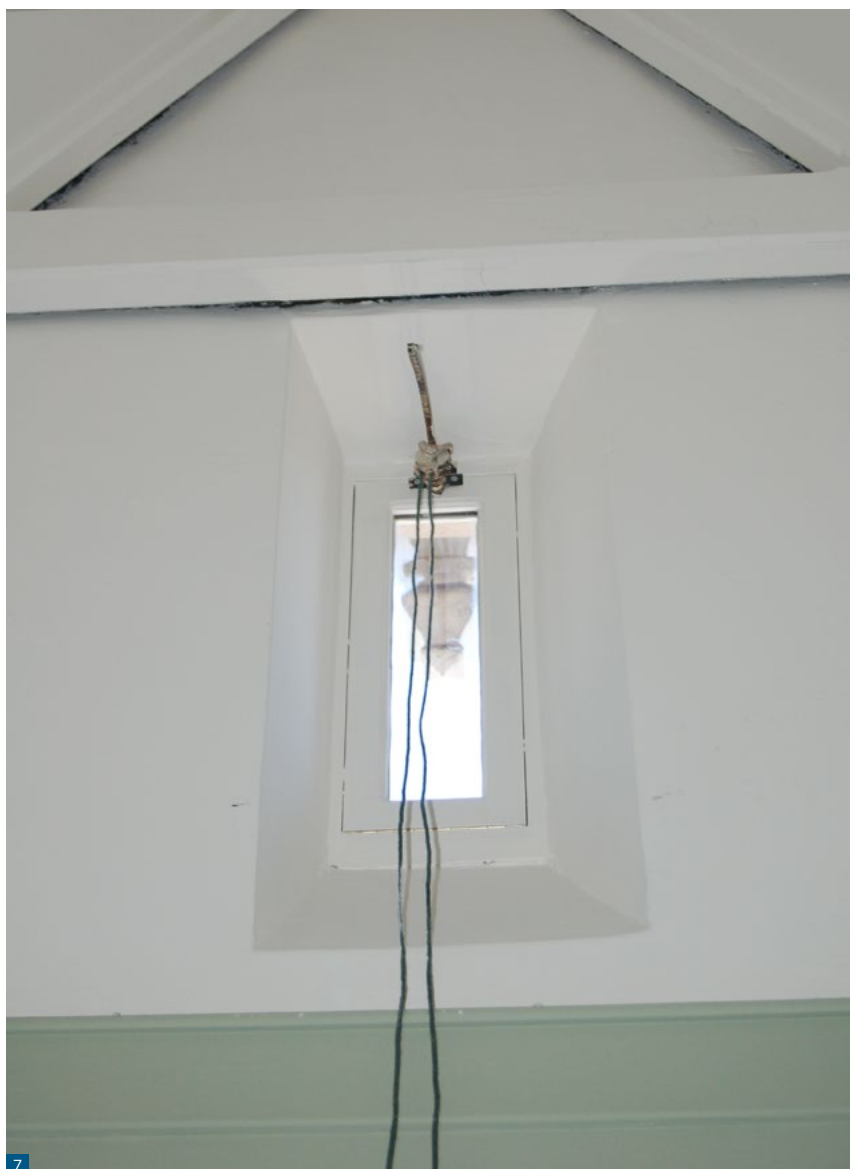
Figure 7: This quarter light has been made to open to allow managed ventilation.
