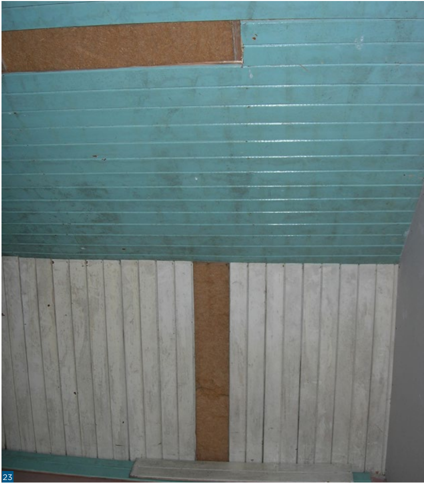
Figure 23: Wood fibreboard used behind an existing timber lining on a coom.
