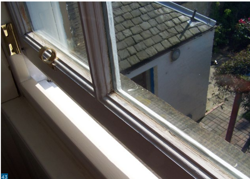
Figure 43: Narrow profile double glazed panes set into an existing window sash. Image © Gordon Barclay
