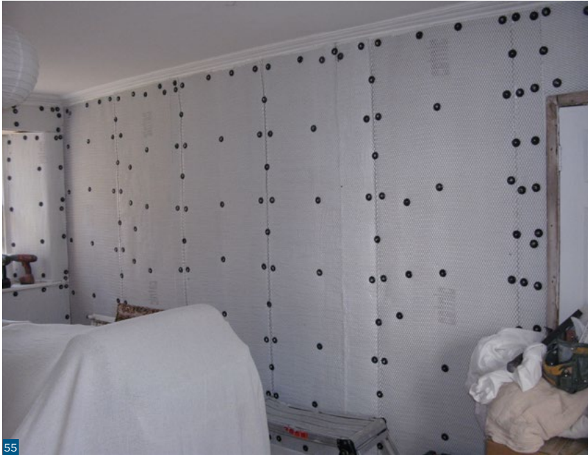
Figure 55: Aerogel blanket applied directly to masonry using thermally decoupled expansion fasteners ( Refurbishment Case Study 3 ).
