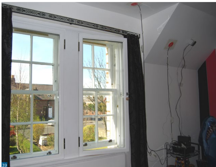
Figure 39: Timber framed secondary glazing in a dormer window.
