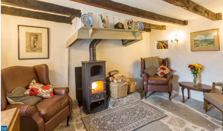
Figure 58: The finished room at Downie's Cottage showing the insulated lime plaster and the relaid stone flagstones. Image © Callum Innes
