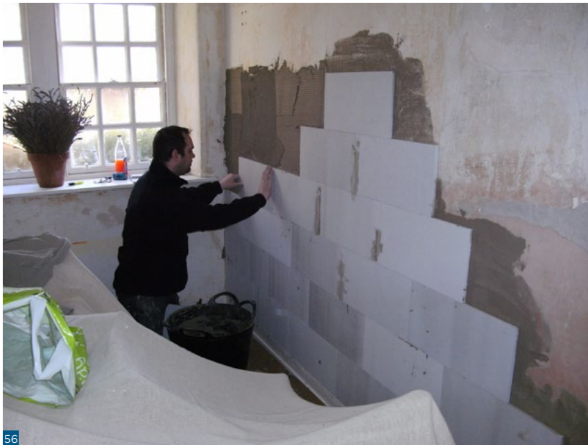
Figure 56: Application of calcium silicate insulating boards.
