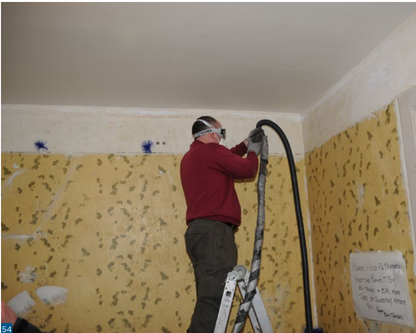
Figure 54: Cellulose fibre being blown behind lath and plaster.
