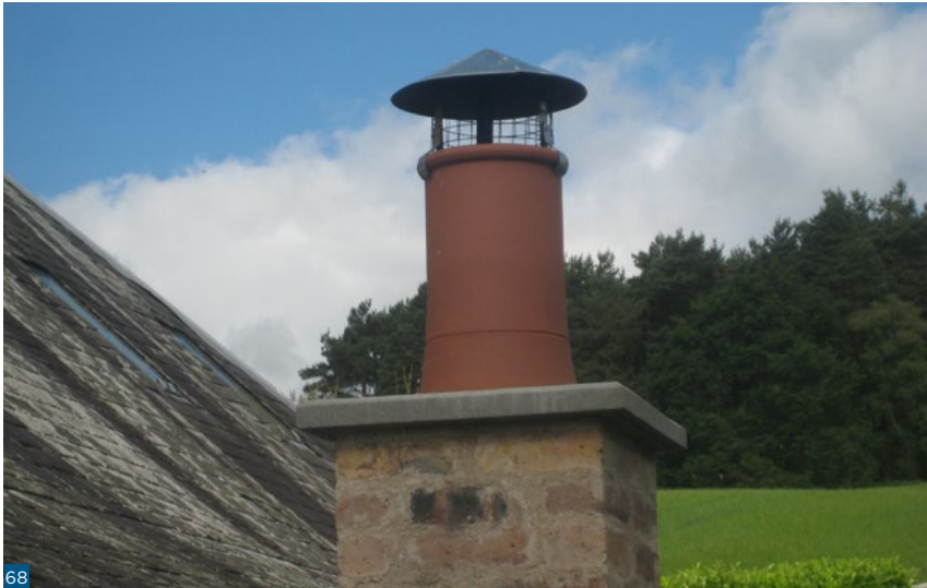
Figure 68: A cowl with mesh keeps a chimney dry but ventilated and free of birds.
