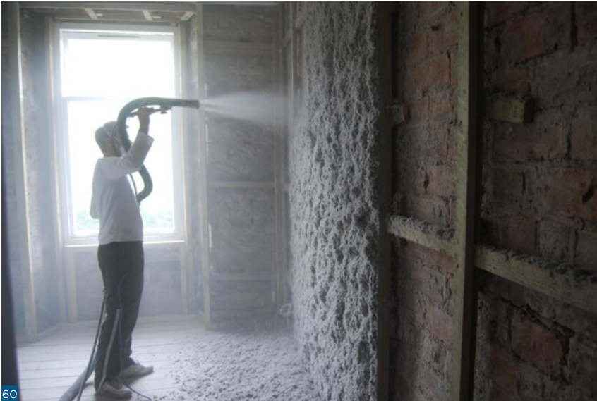
Figure 60: Cellulose insulation being applied damp.
