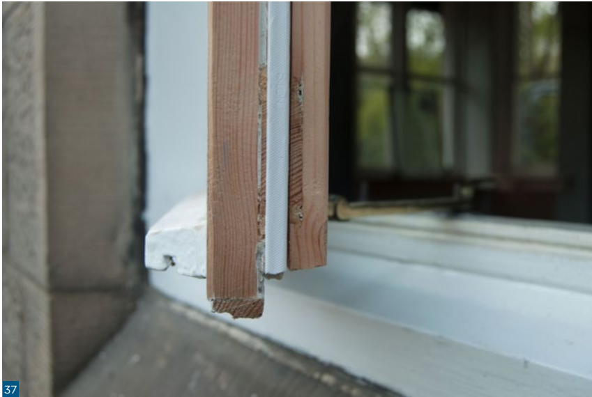
Figure 37: A newly fitted brush strip (white) on a casement window at Holyrood Park Lodge.
