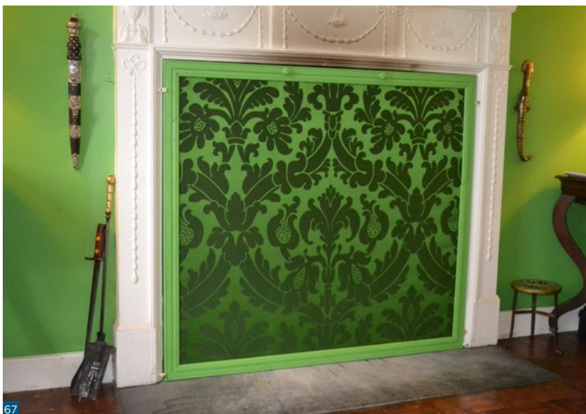
Figure 67: A hearth board used to temporarily close off a fireplace.
