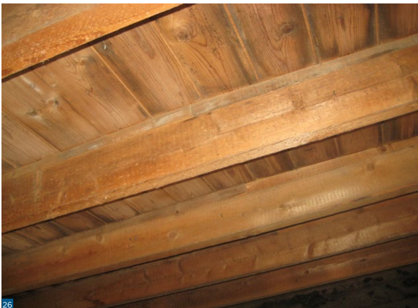
Figure 26: A typical underside of a flat roof.
