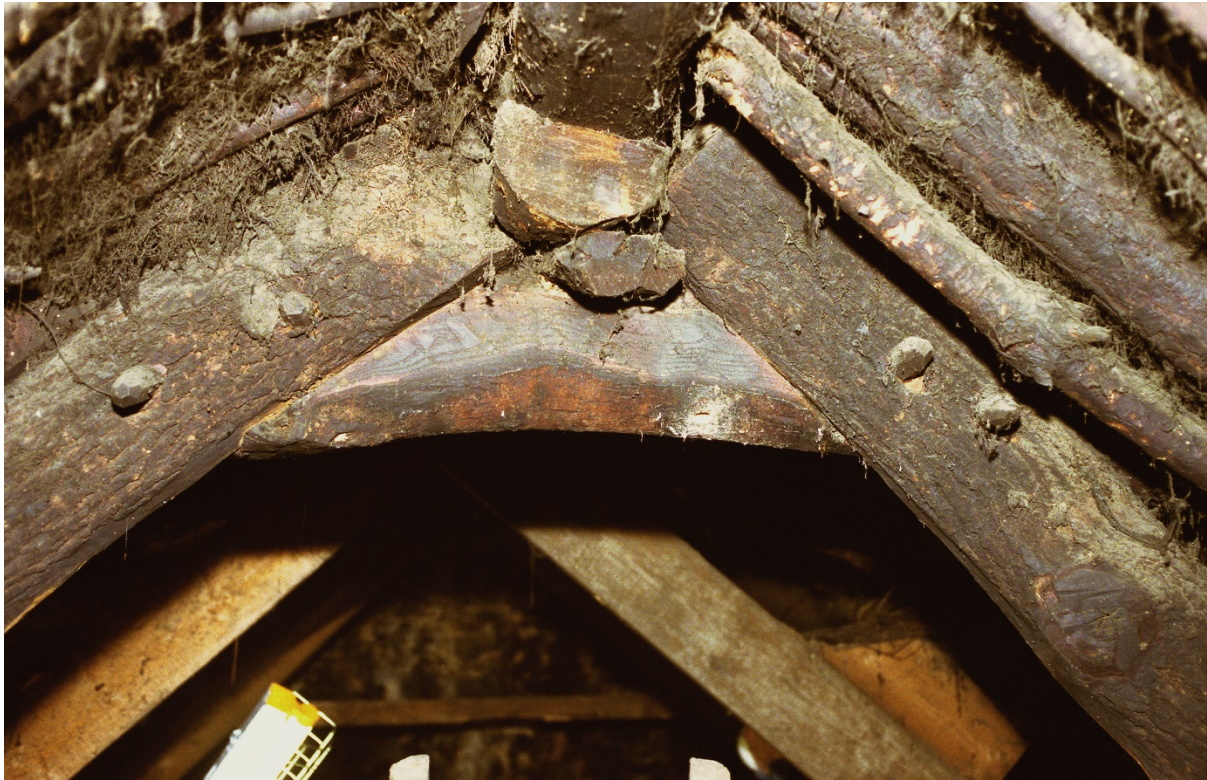
Figure 5: Detail of apex of east couple, with visible pegging © Crown Copyright HES
