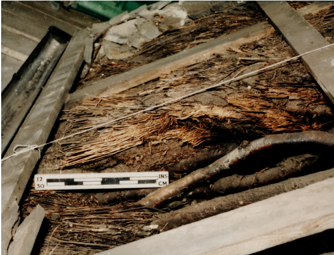
Figure 6: Detail of thatch, preserved beneath the corrugated iron roof © Crown Copyright: HES.
