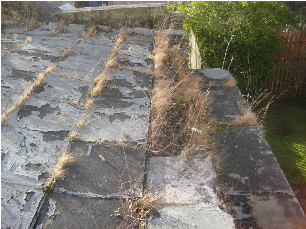
Fig. 2. The condition of the roof covering prior to the 2014 works
