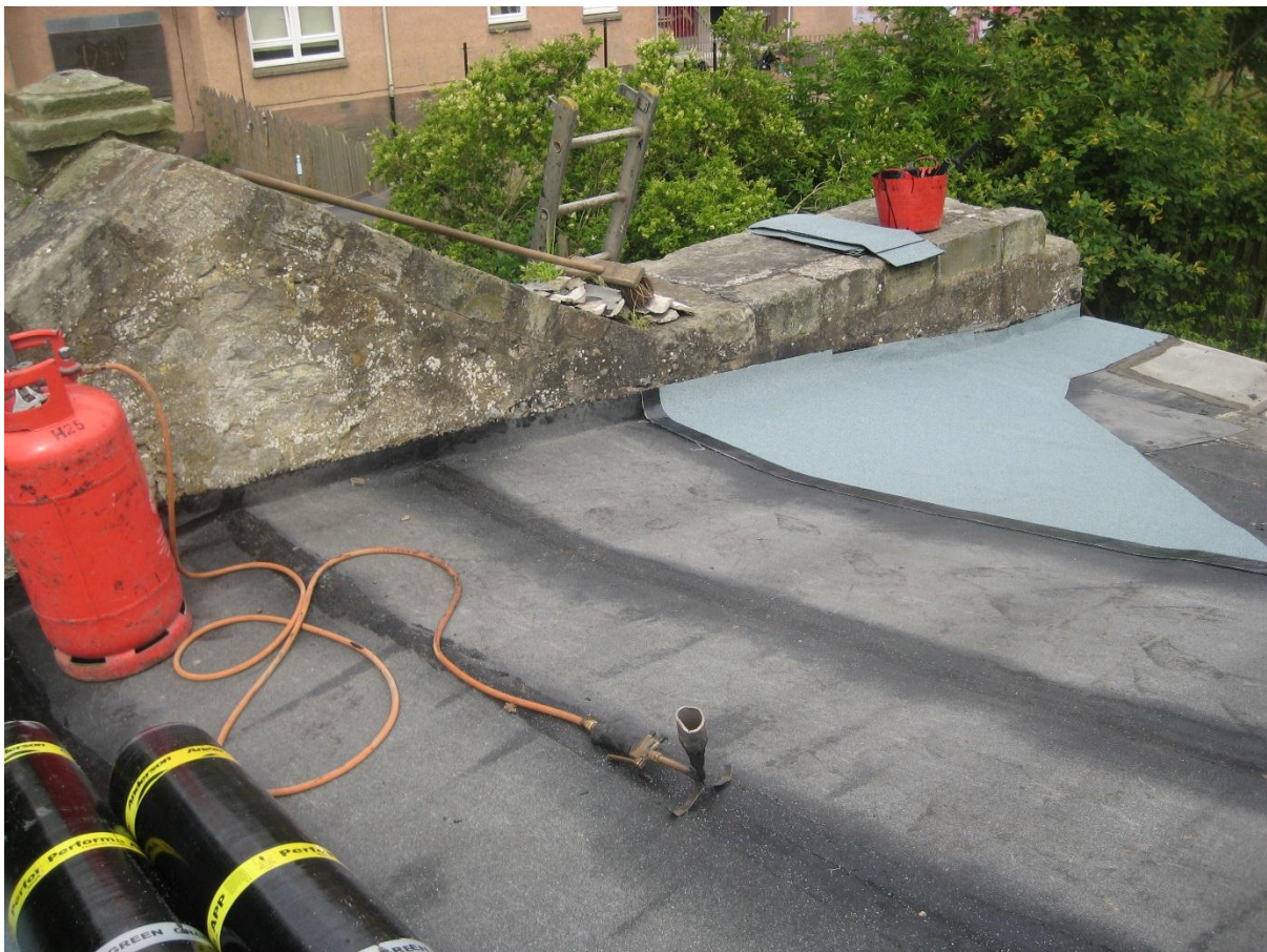
Fig. 3. The application of the bitumen felt covering
