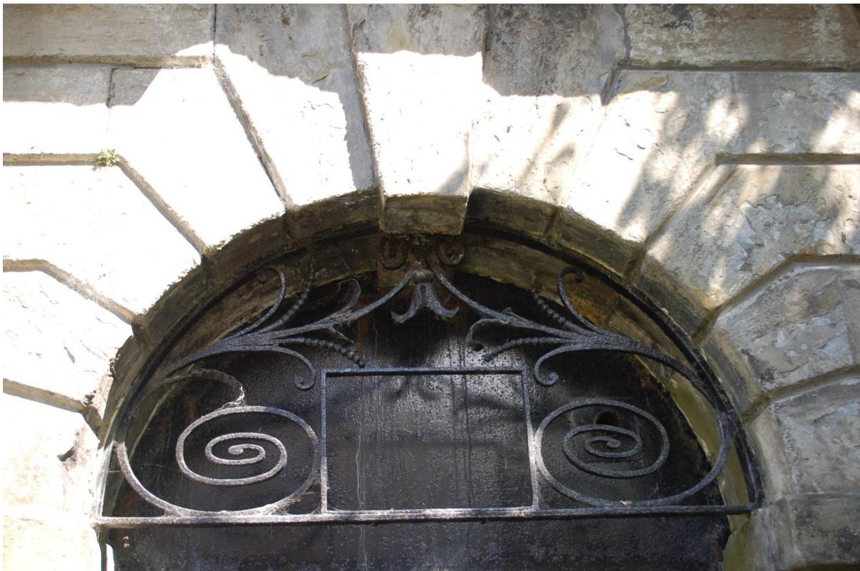
Fig. 6. Original wrought iron screen in front of the modern steel door
