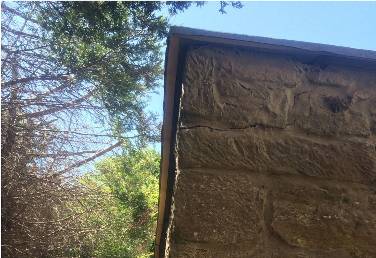
Fig. 4. The finished edge detailing
