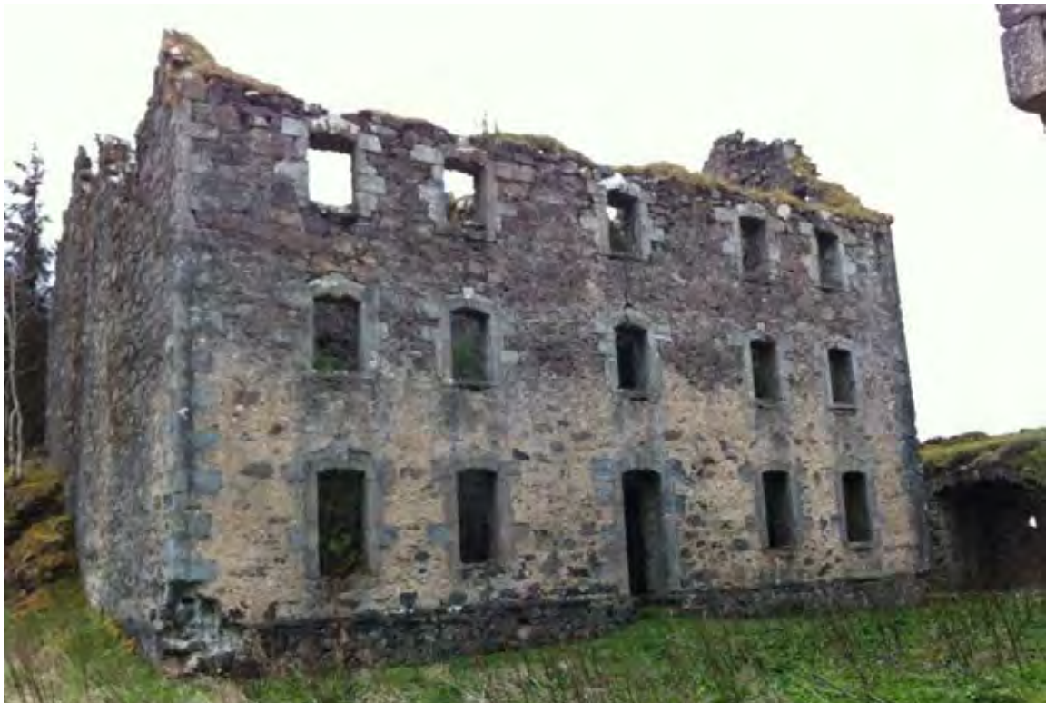
Figure 30.1. Principal elevation of the barracks.
