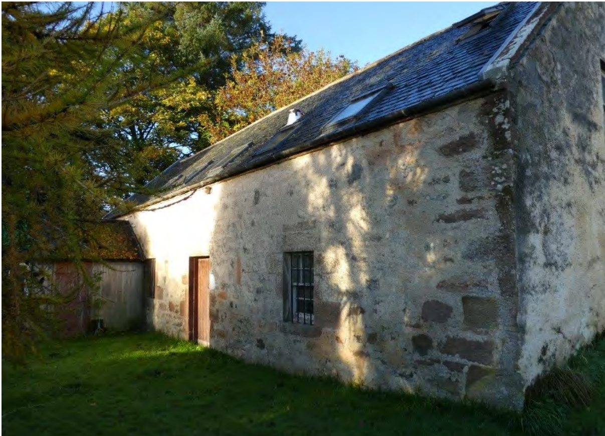
Figure 47.1. Rear elevation of the cottage.
