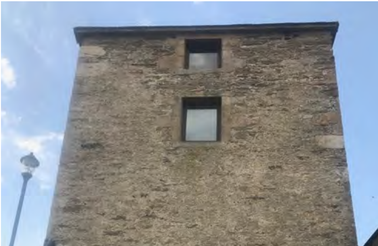
Figure 41.1. View of the east gable.
