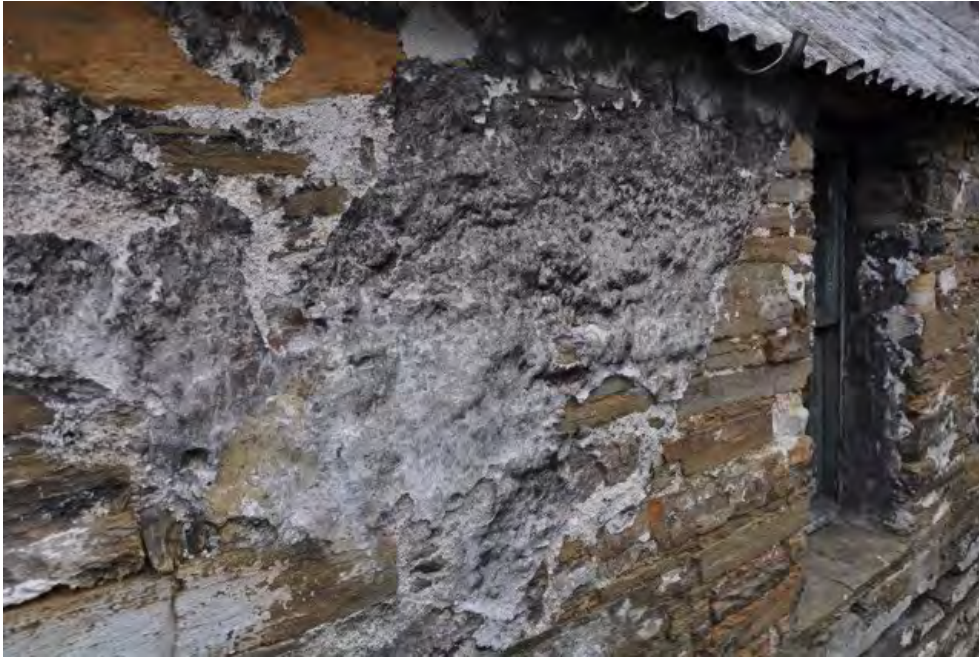
Figure 20.2. Well-preserved areas of harl displaying multiple limewash coats.
