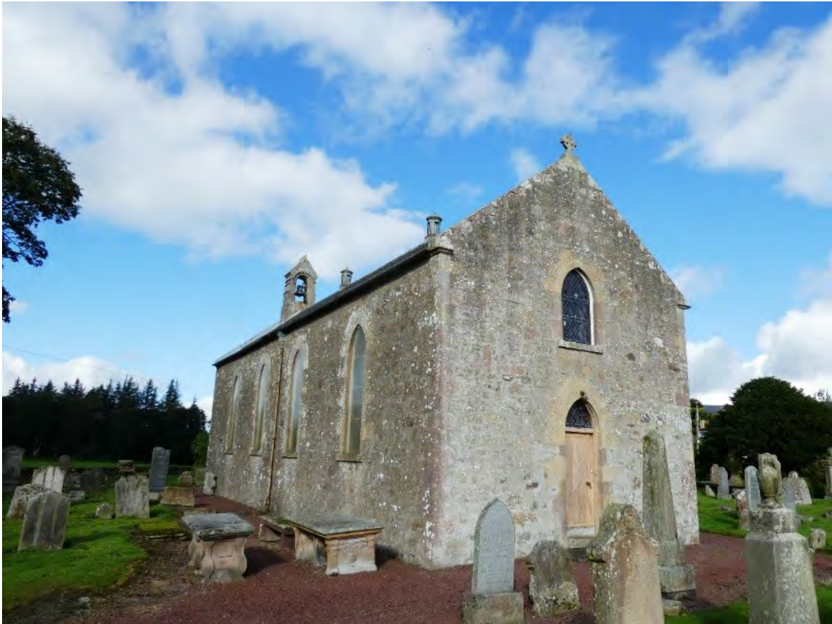
Figure 27.1. General view of the church.
