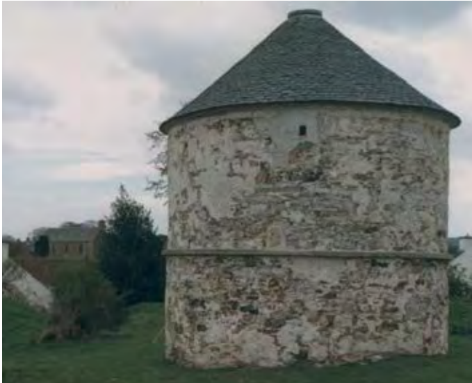
Figure 24.1. The doocot following removal of the cement harl.
