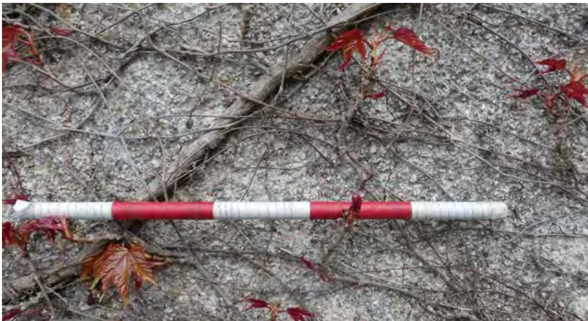
Figure 70.2. Detail of harl underneath the ivy.
