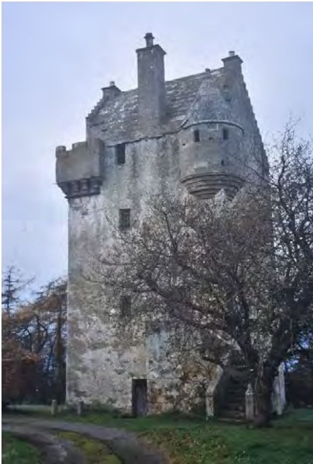
Figure 16.1. Side elevation of the tower in 1993, prior to re-harling.
