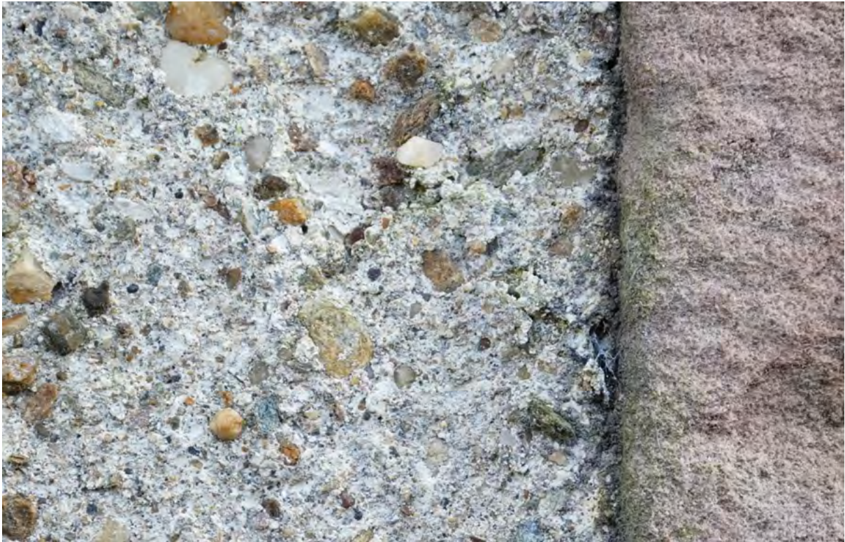
Figure 55.3. The harl coat coming up against a window band.
