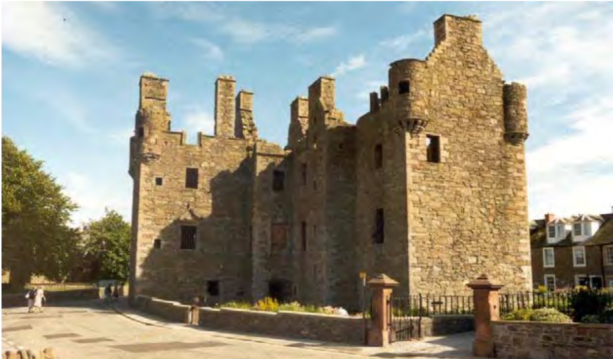
Figure 11.1. View of the castle from the north elevation.
