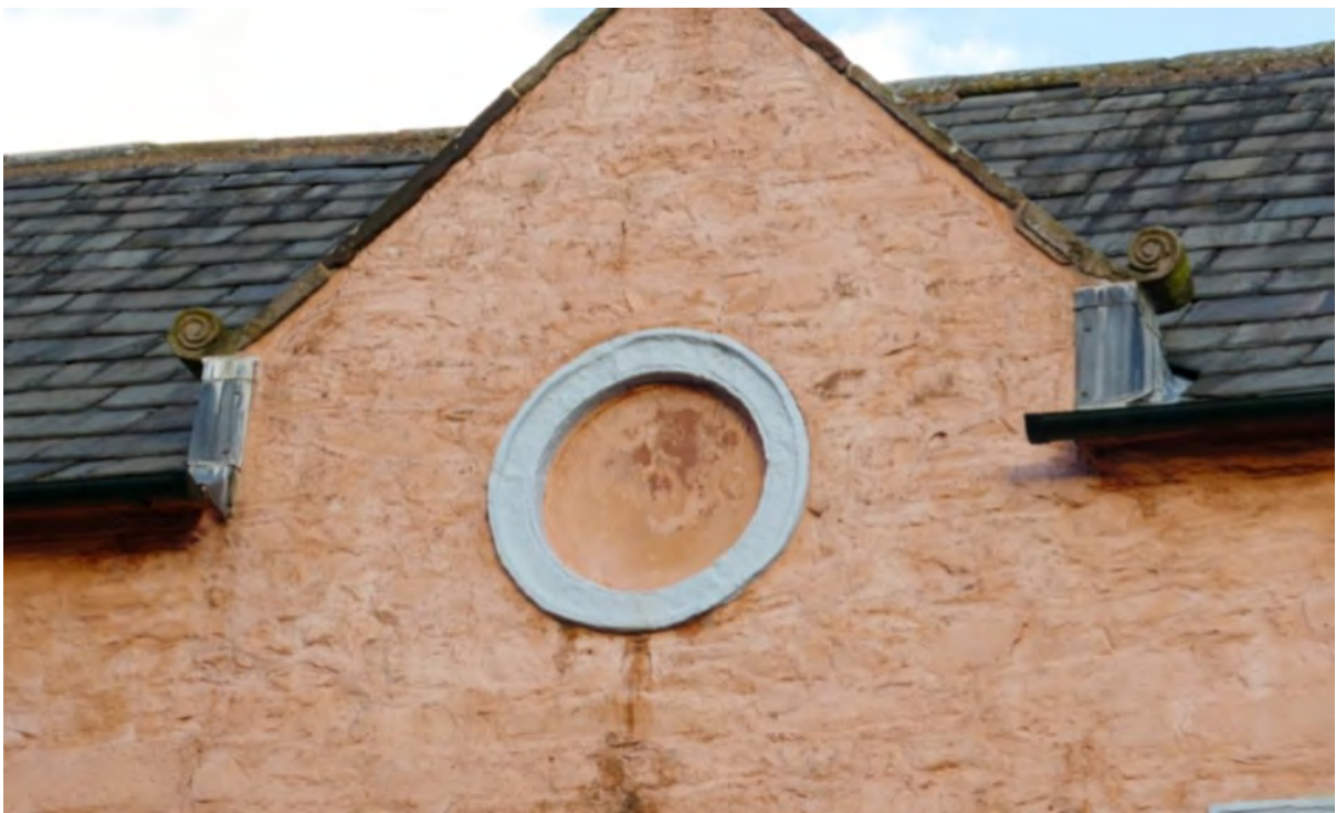
Figure 22. Broughton House, Kirkcudbright. Limewashed masonry elevation with no harl.
