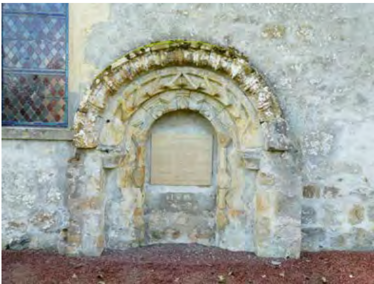
Figure 27.3. The 13th century arch with remains of limewash or fine plaster.
