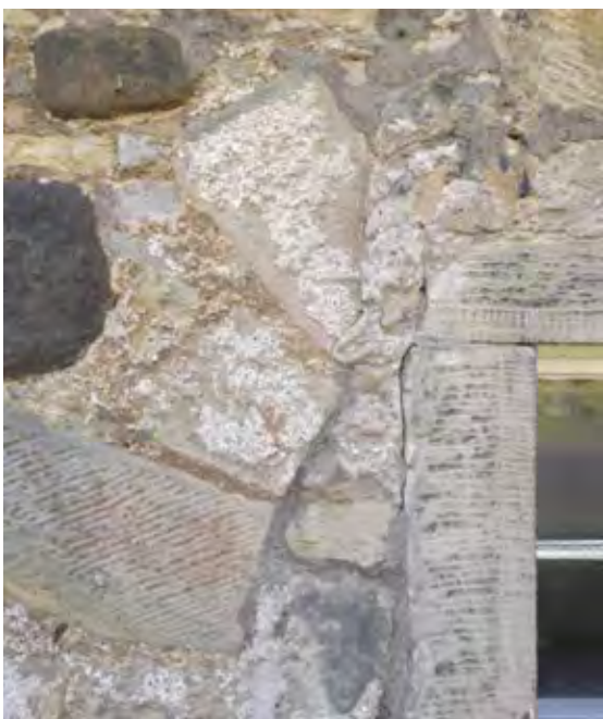
Figure 66.4. A thin harl taken over the dressed stones.
