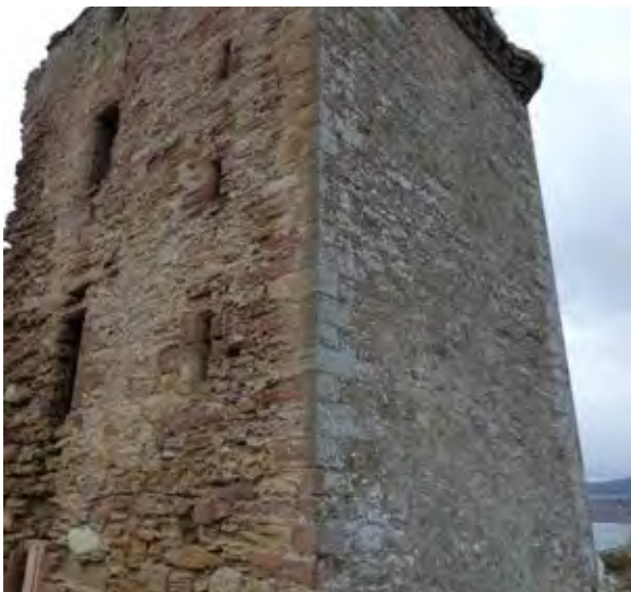
Figure 03.2. View of the north-east corner of the building.
