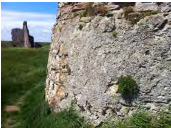
Figure 10.2. Large area of harl; the remains of Newark Castle are visible in the distance.
