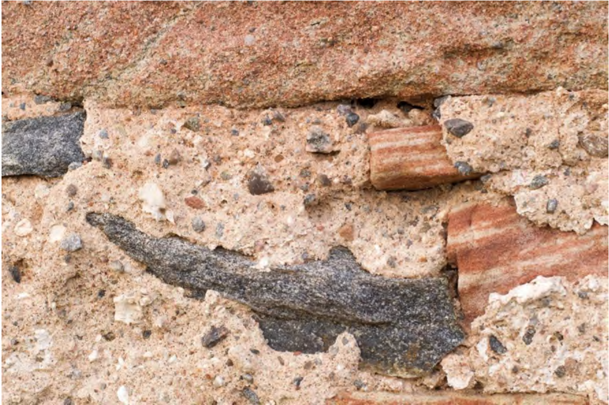
Figure 65.2. Detail of integrated harl finish.
