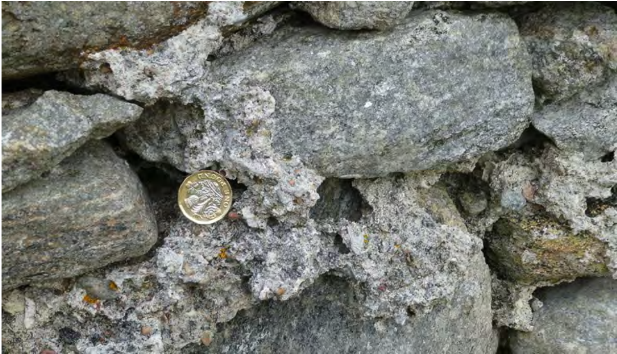
Figure 02.2. Integral bedding mortar and harl on the east gable.
