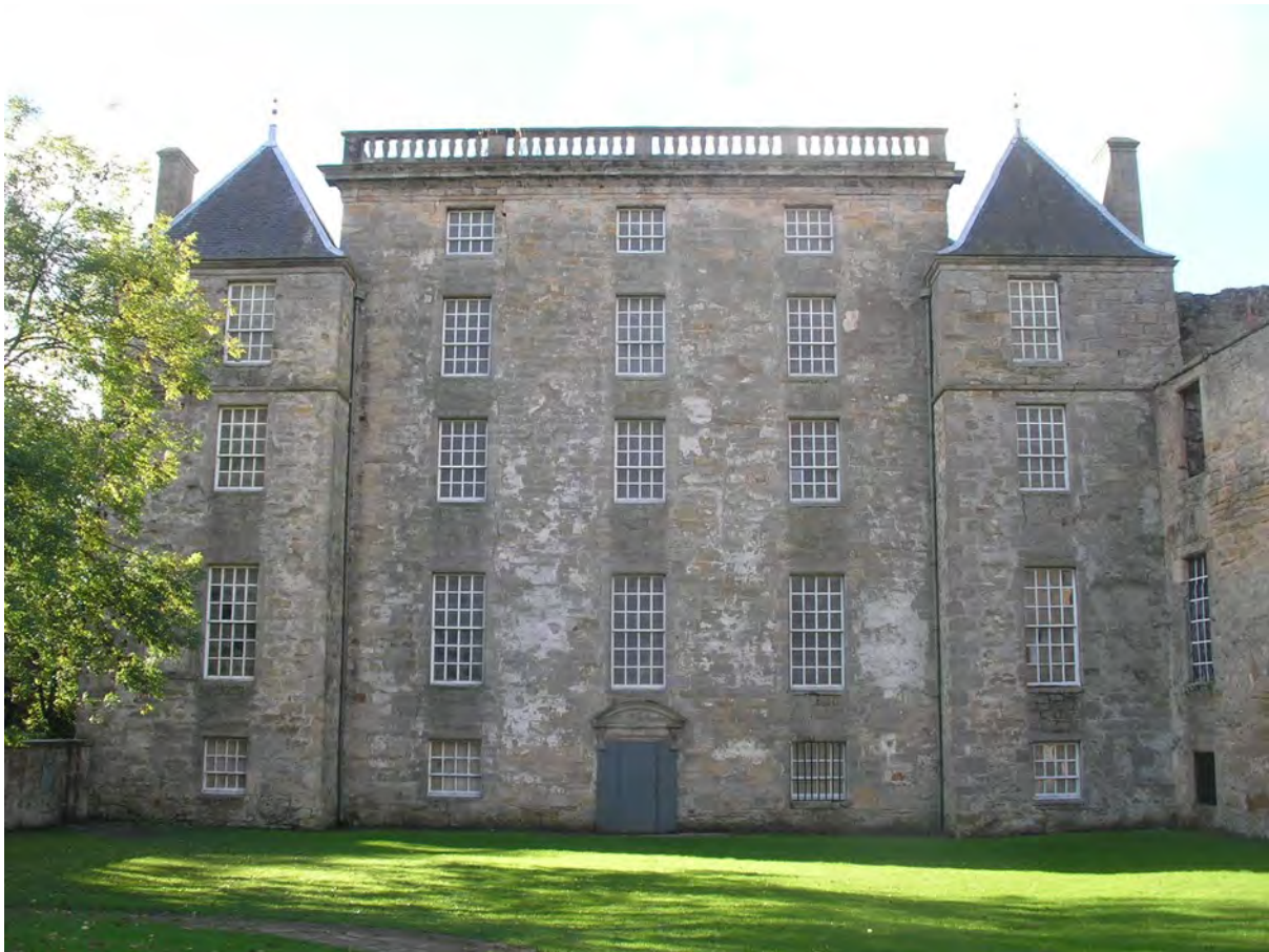
Figure 17.1. Kinneil House in 2013. Some vestiges of lime finishes remain.
