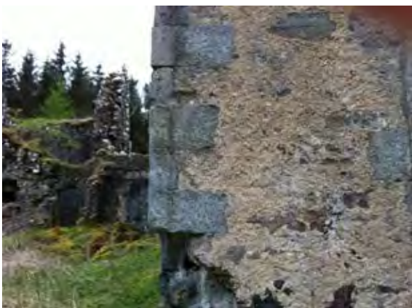
Figure 30.5. Surviving fragments of harl near the quoins.
