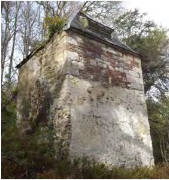
Figure 42.1. The south side of the structure showing the 19th century rebuild of its upper parts.
