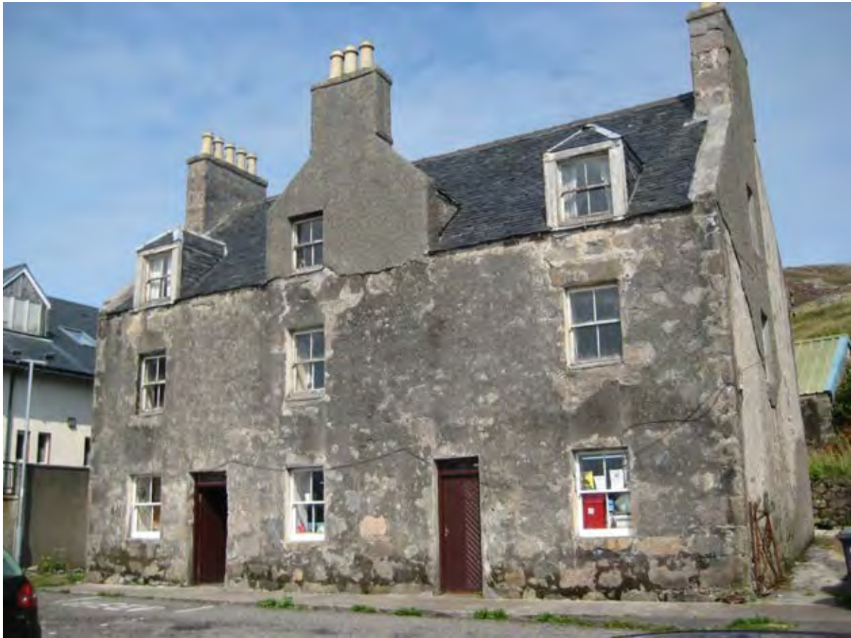
Figure 53.1. The front elevation of the shop
