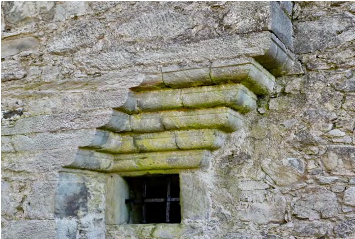
Figure 14.3. Harl running up to the corbelled feature on all sides
