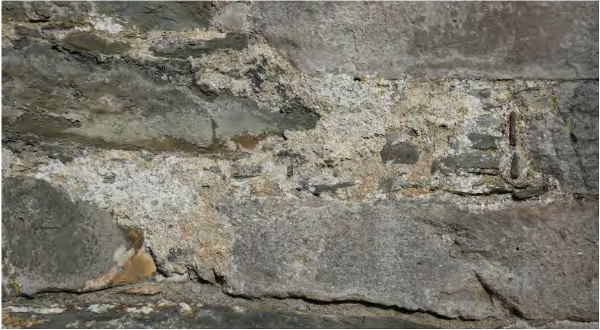
Figure 11.2. Remaining harl on the south west elevation.
