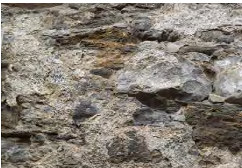
Figure 32.2. Detail of remaining harl.
