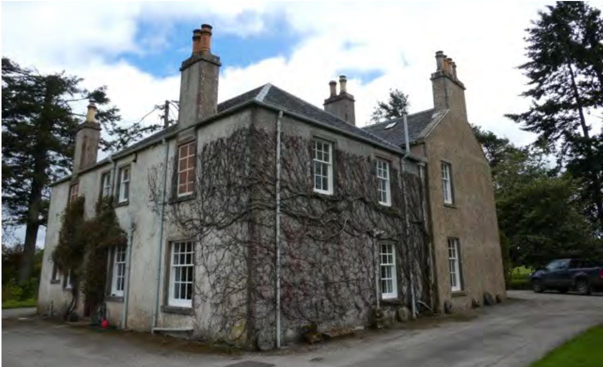
Figure 70.1. General view of the manse, with extensive ivy coverage.
