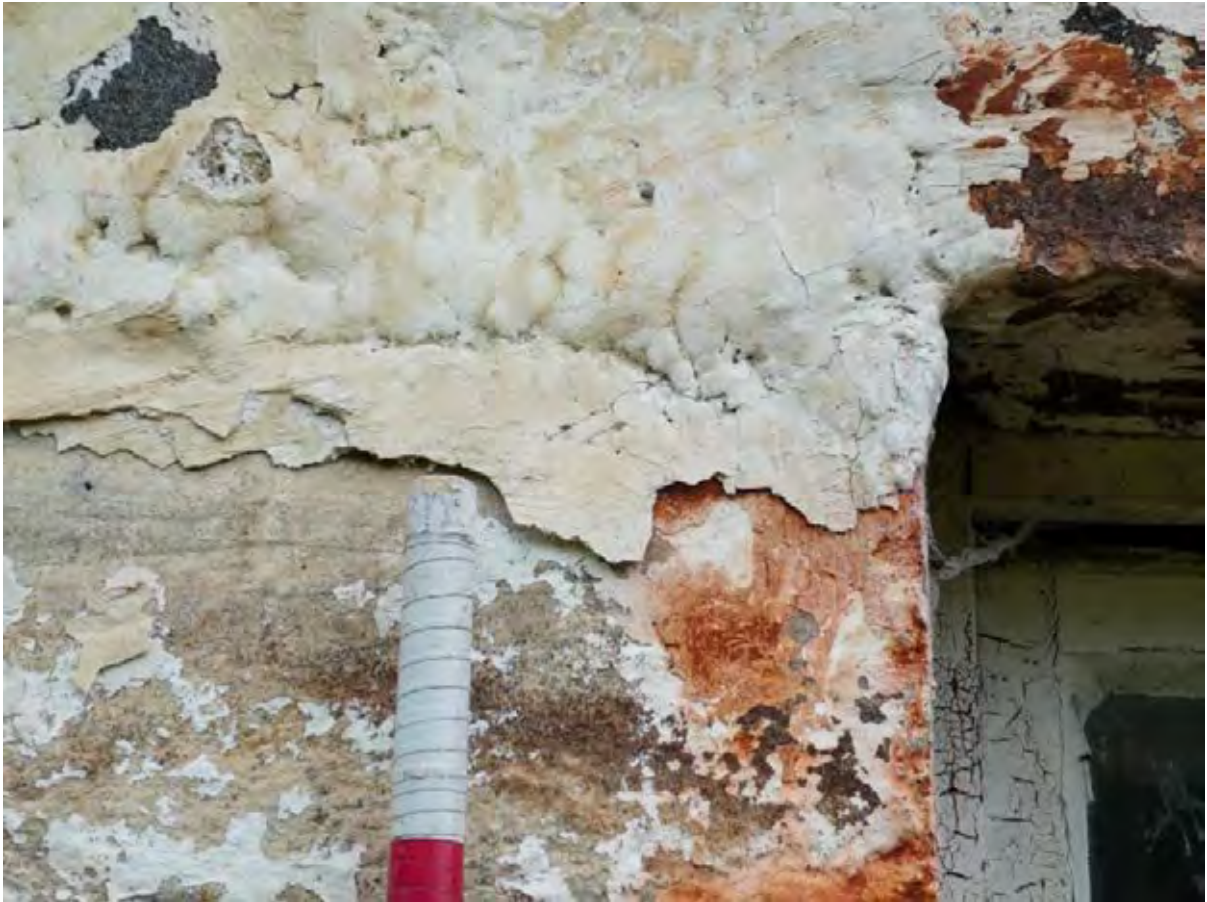
Figure 62.3. Area of remaining harl.
