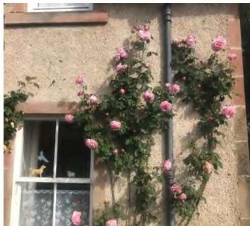
Figure 72.3. Detail of the front elevation showing the neat junction with the window jambs.
