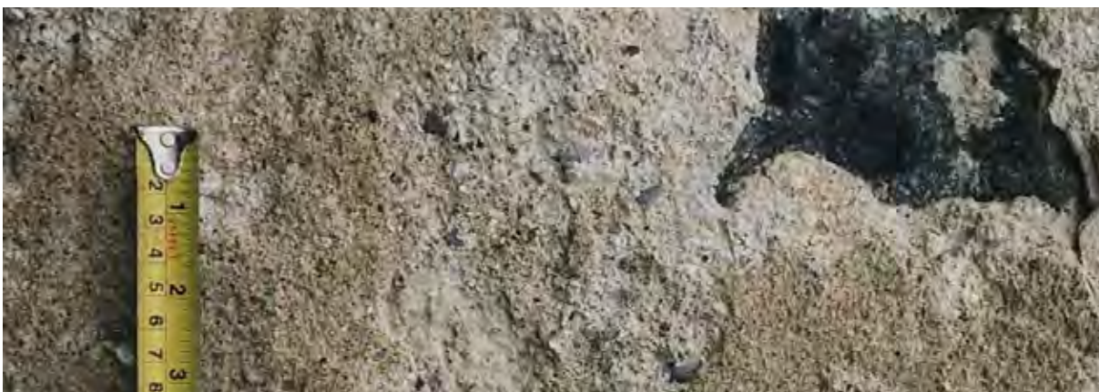
Figure 24.2. Detail of the build-up of external finishes.
