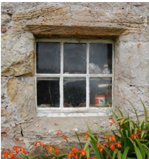
Figure 15.2. Visible traces of harl on the left side of the window.
