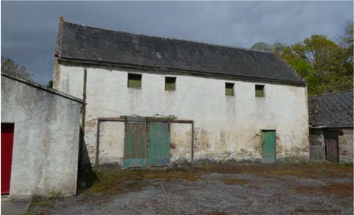
Figure 22.1. Principal elevation of the barn.
