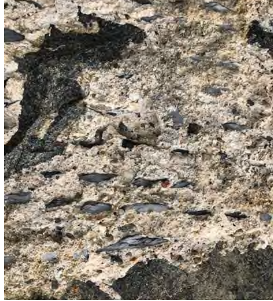
Figure 41.3. Detail of the harl.
