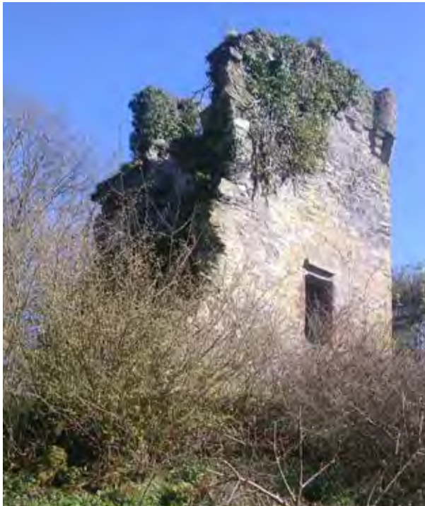
Figure 04.1. The tower looking south-east.
