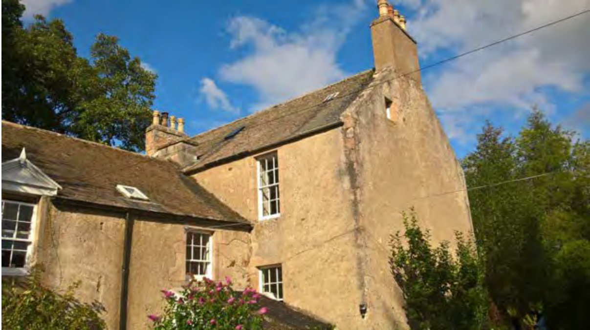
Figure 36.3. The rear elevation of the house. Some decay of the render evident from the run off from the skew cope.
