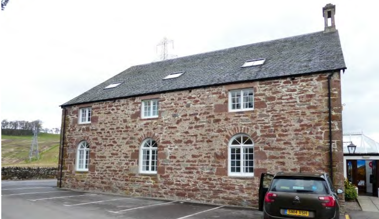
Figure 33.1. Rear elevation of the building.
