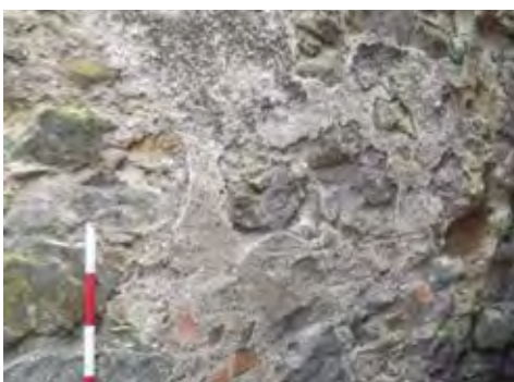
Figure 31.2. Harl application in Balmerino Place.
