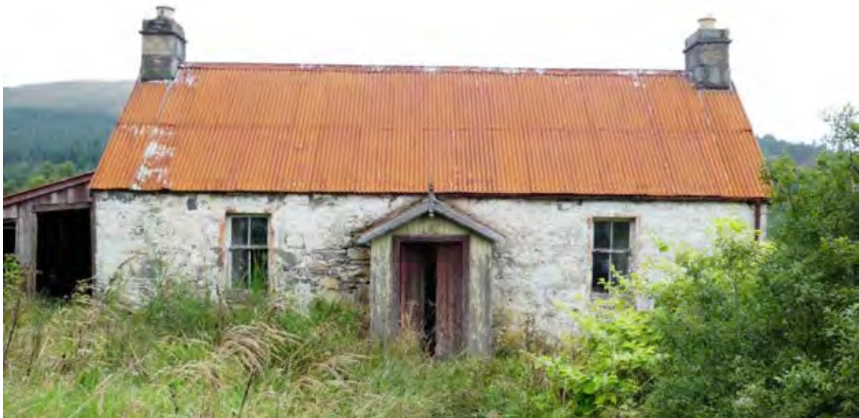
Figure 62.1. Front elevation of the cottage.
