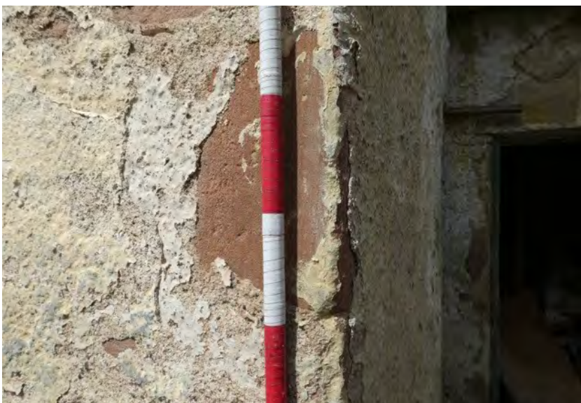
Figure 22.4. Harl taken over the door jamb.
