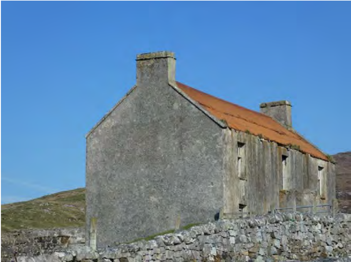
Figure 50.1. General view of the store house.
