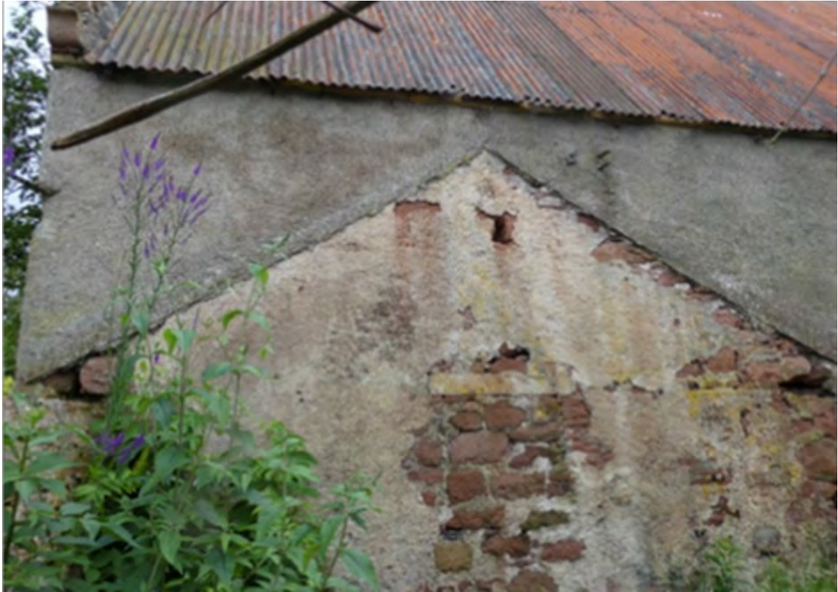
Figure 5. Townland's Barn, historic harl revealed by loss of an extension.
