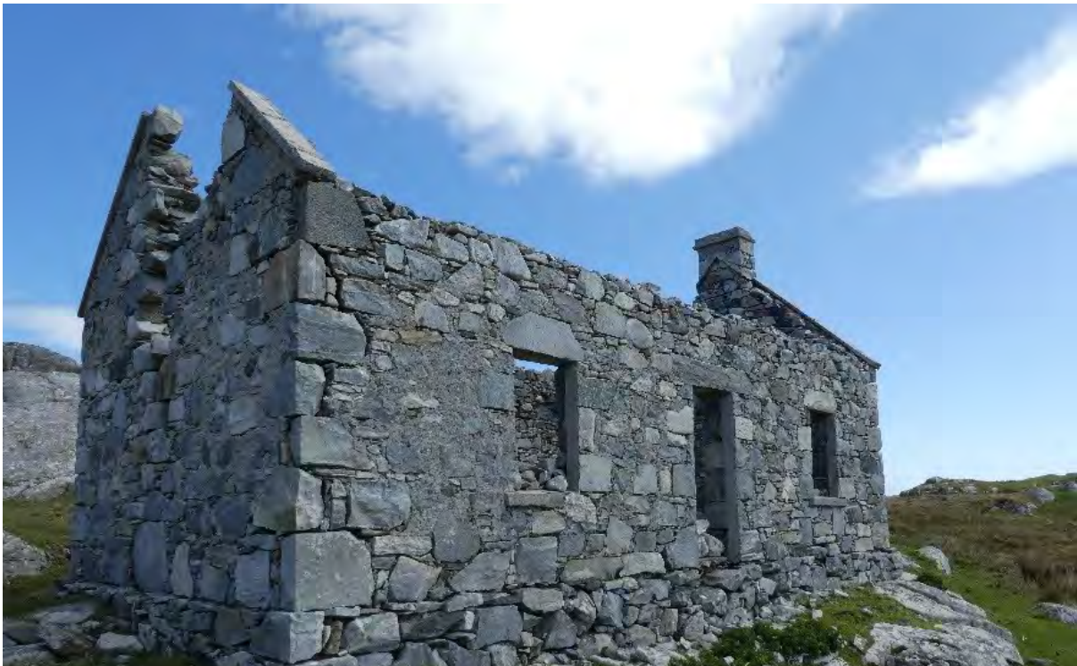
Figure 59.1. The south west elevation of the cottage at Manish.
