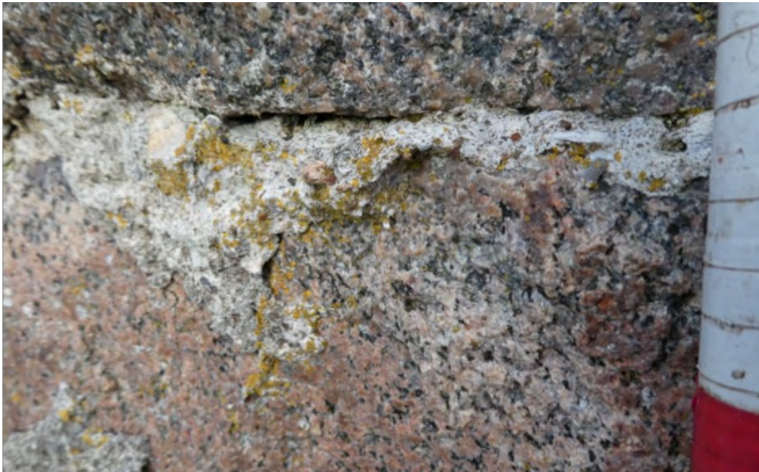
Figure 25. Orchardton Tower, Dumfries and Galloway. The bedding mortar inseparably combined.
