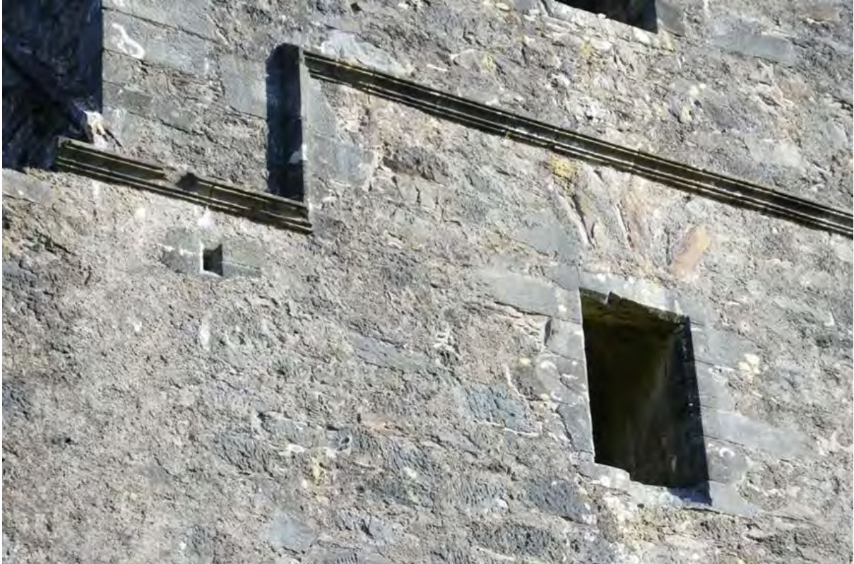
Figure 14.2. Extensive surviving areas of exterior harl finish on the South elevation.
