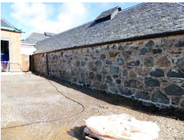
Figure 54.2. The steading after removal of the harl.
