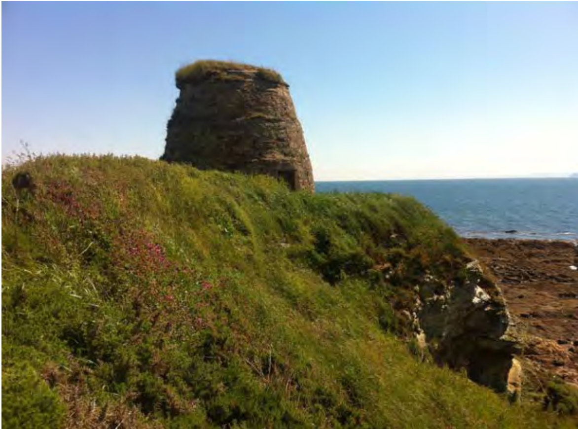
Figure 10.1. General view of the exposed cliff-top location of the doocot.
