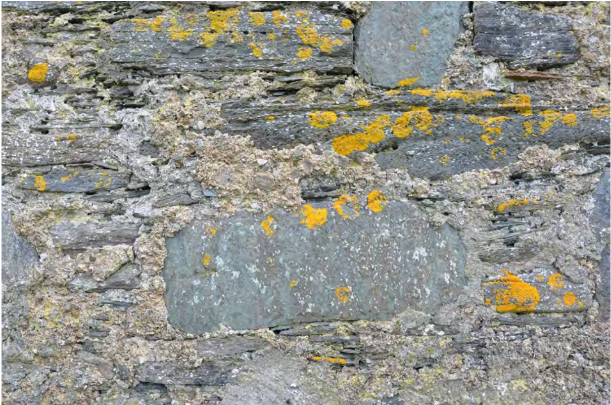
Figure 01.3. The harl appears to be lime rich, with a marine aggregate occasionally showing quite large fragments of shell in the mix.
