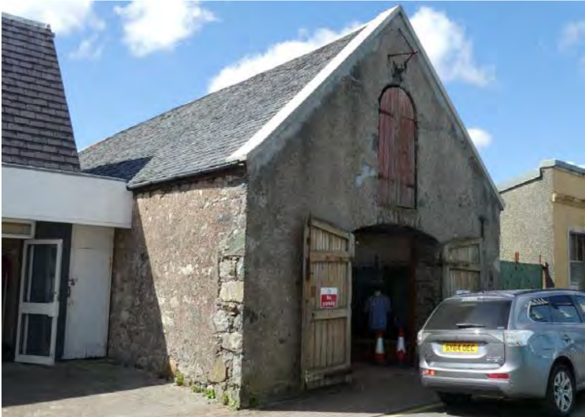
Figure 68.1. View of the warehouse from the main entrance.
