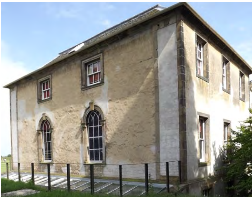
Figure 26.4. The subsidiary north elevation.
