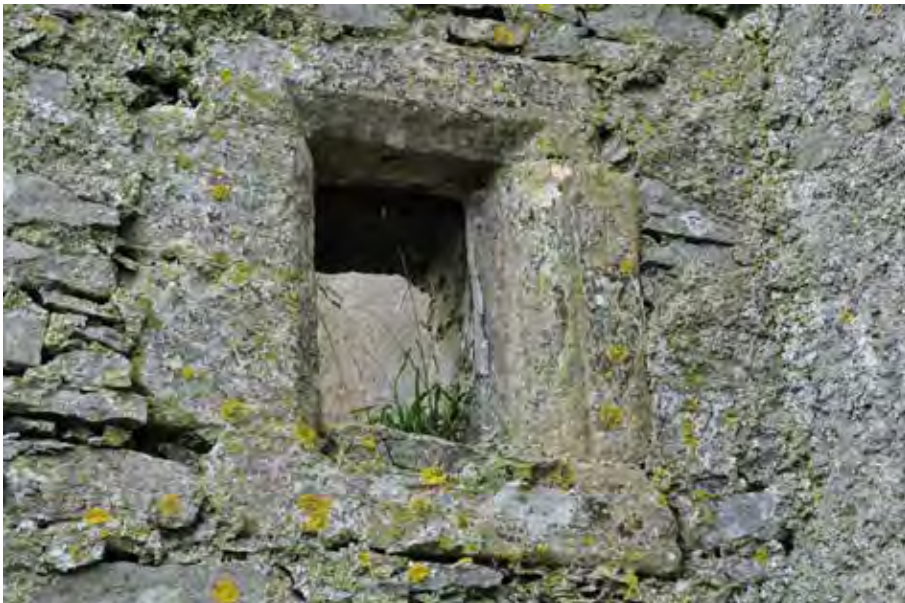
Figure 18.3. Area of harl surviving around window detail.
