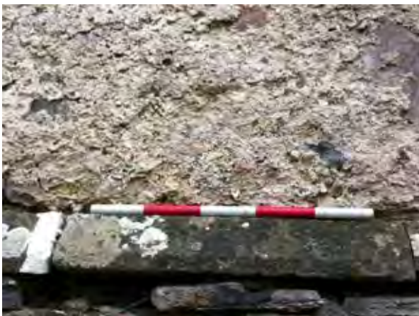
Figure 30.4. Large area of surviving harl.
