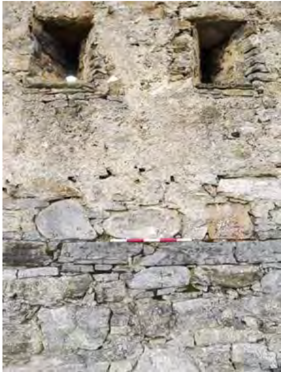
Figure 25.4. Well preserved harl remains on the exterior of the perimeter.
