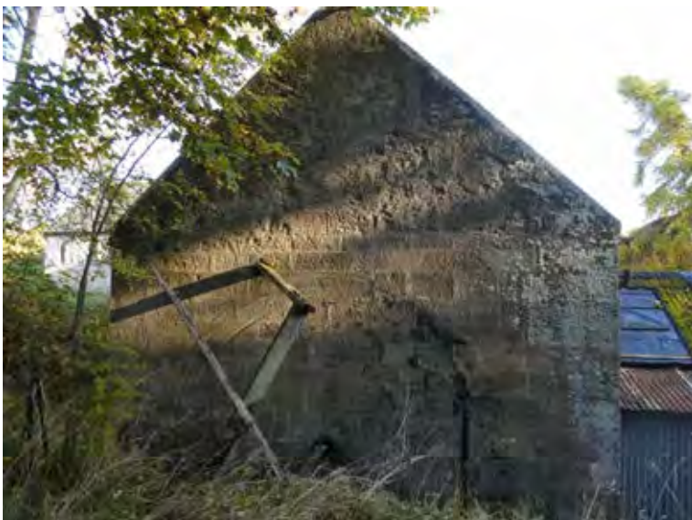
Figure 47.4. The mill gable end, with more dressed masonry blocks laid in lime mortar.
