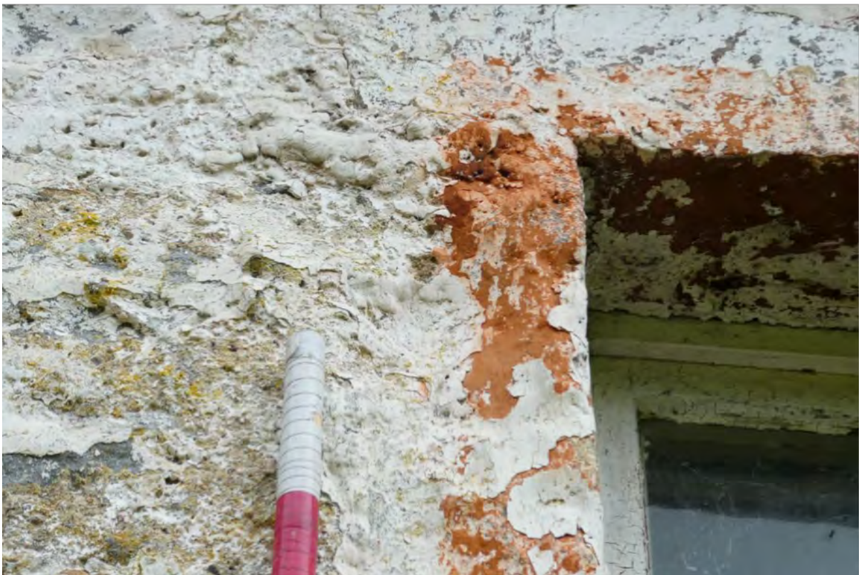
Figure 9. Multi-layered limewash at Gorstan Cottage, Garve.
