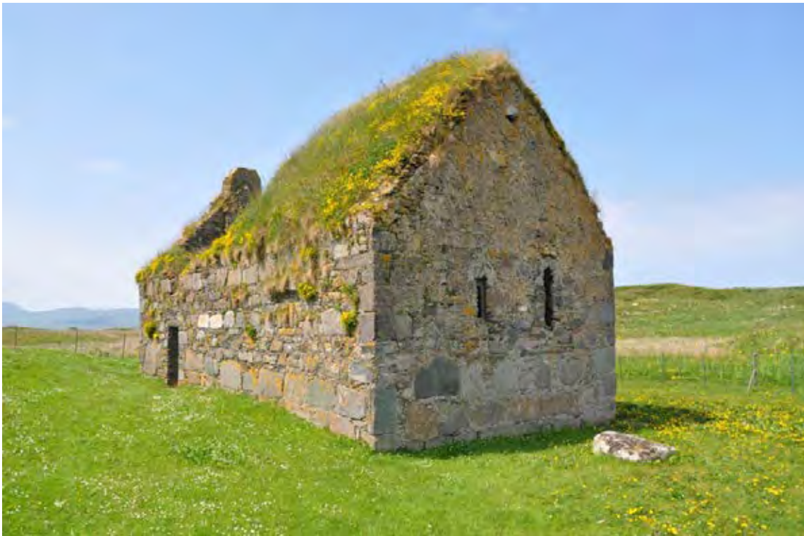
Figure 01.1. The 13th century chapel on Eilean Mor, viewed from the northeast.
