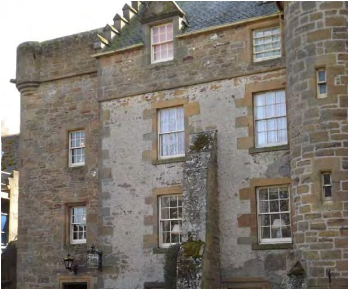
Figure 49.1. General view of the south range of the north frontage.
