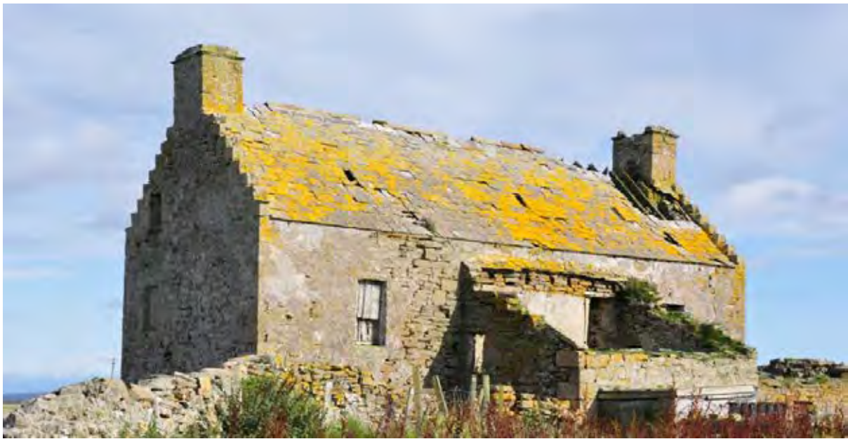
Figure 18.1. The north elevation of Howan.
