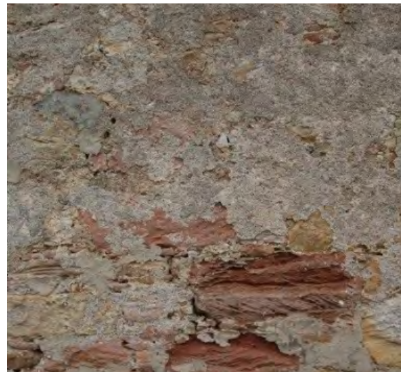
Figure 15.3. Detail of harl.
