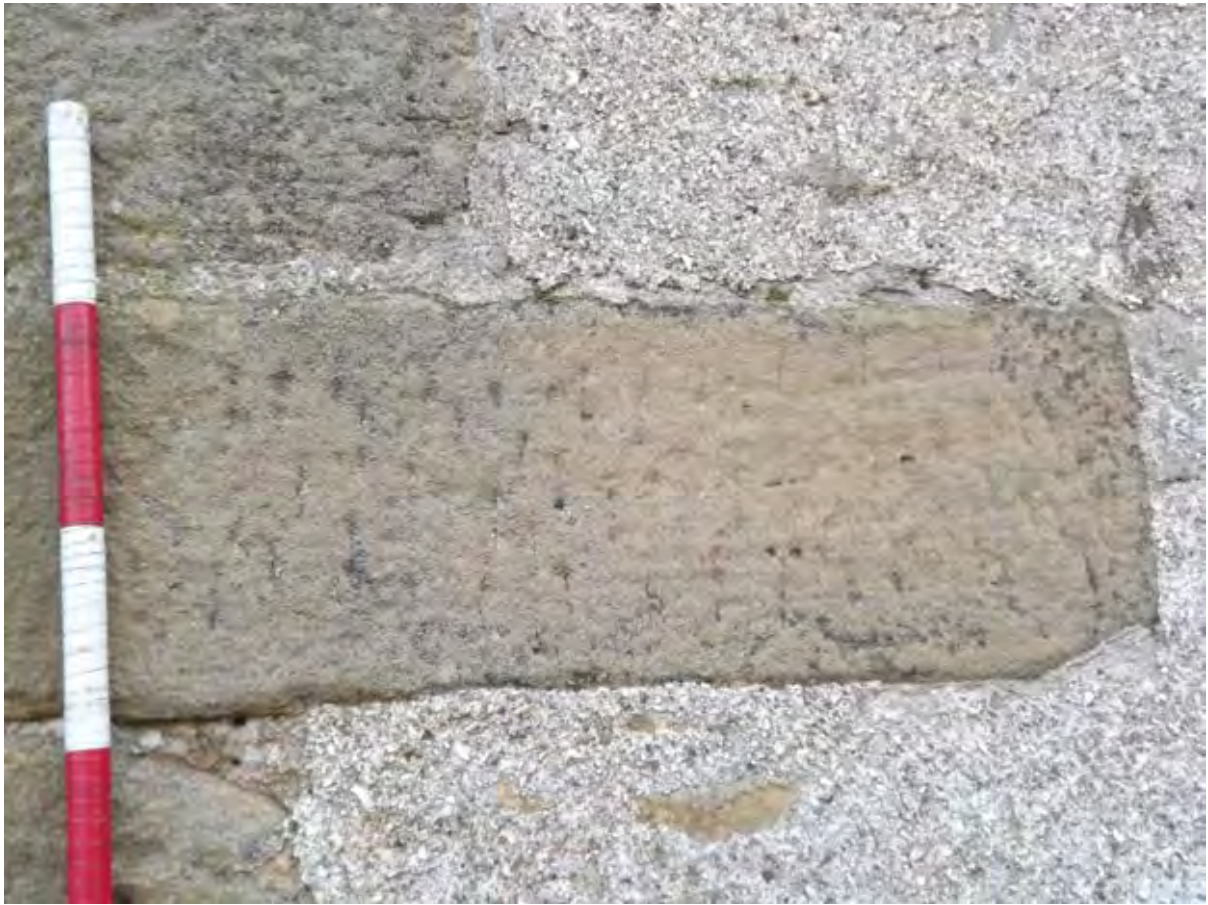
Figure 49.3. Detail of harl running up to quoin.
