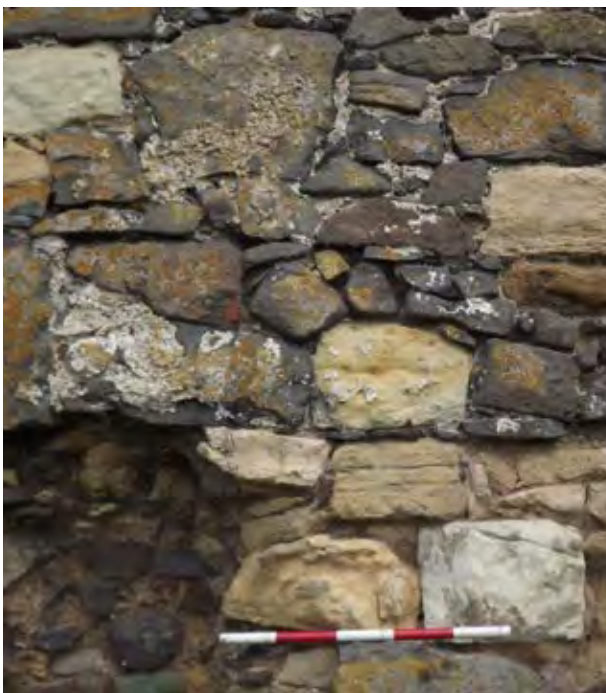
Figure 08.2. Small areas of remaining harl.
