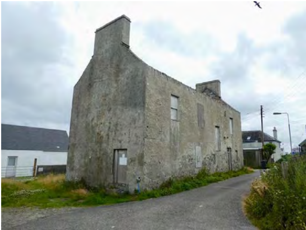
Figure 57.1. General view of McLeans Mansion from the north east.
