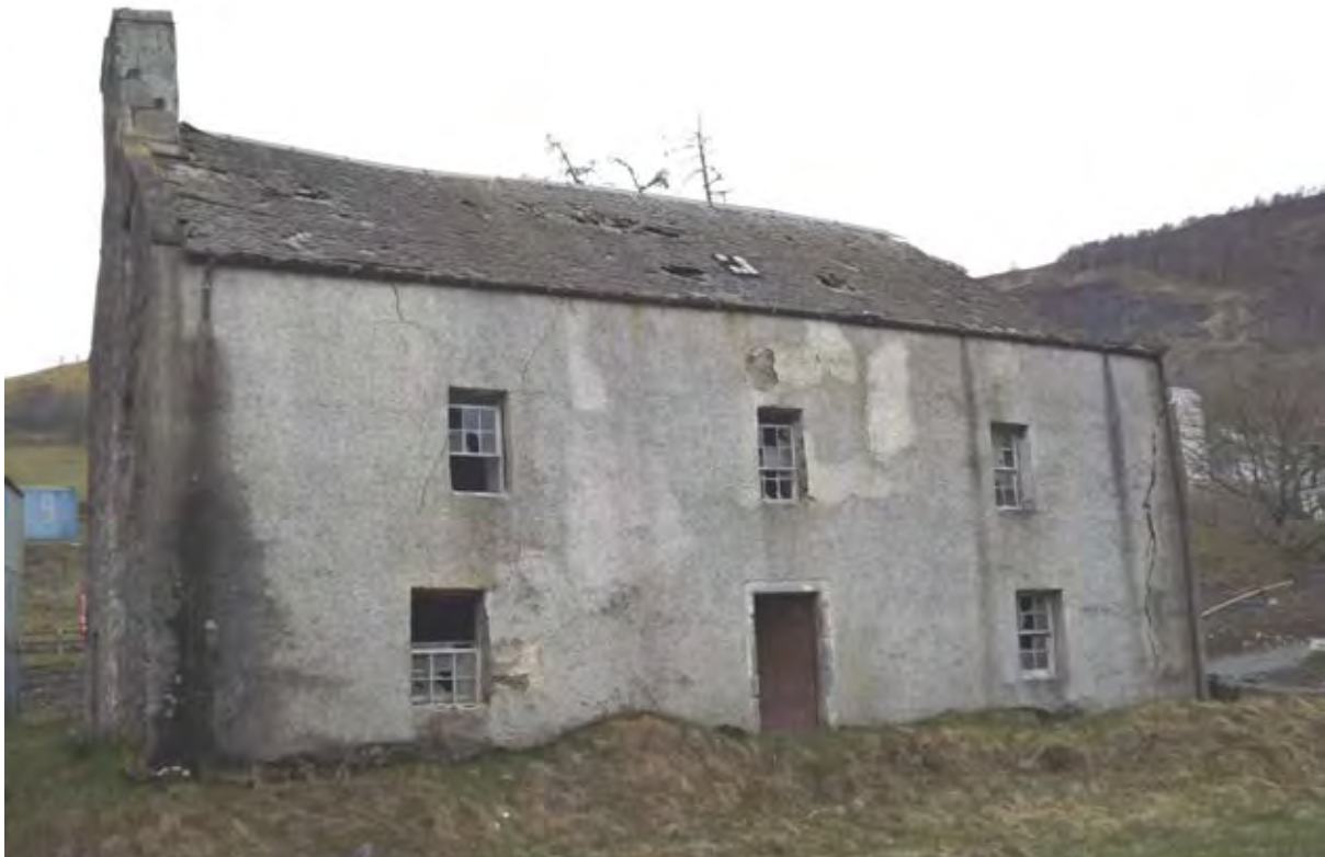
Figure 32.1. General view of the principal elevation.
