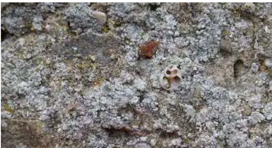
Figure 61.2. Detail of remaining lime harl.
