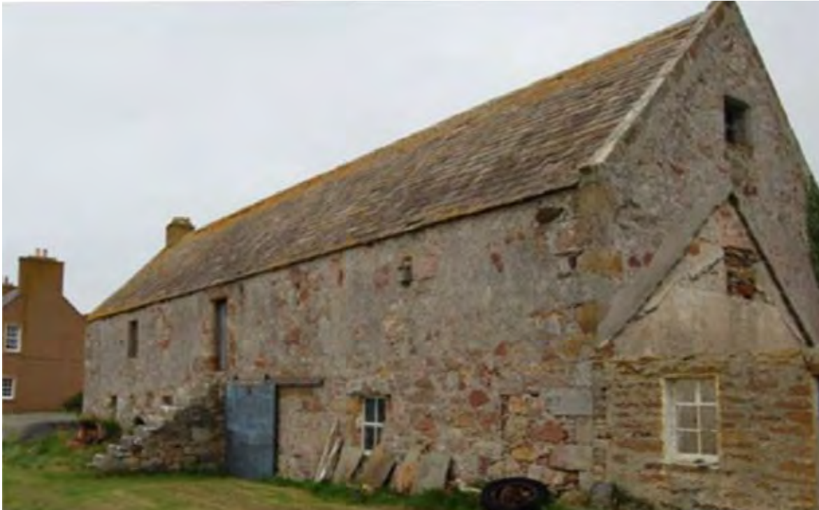
Figure 15.1. Principal elevation of the barn.
