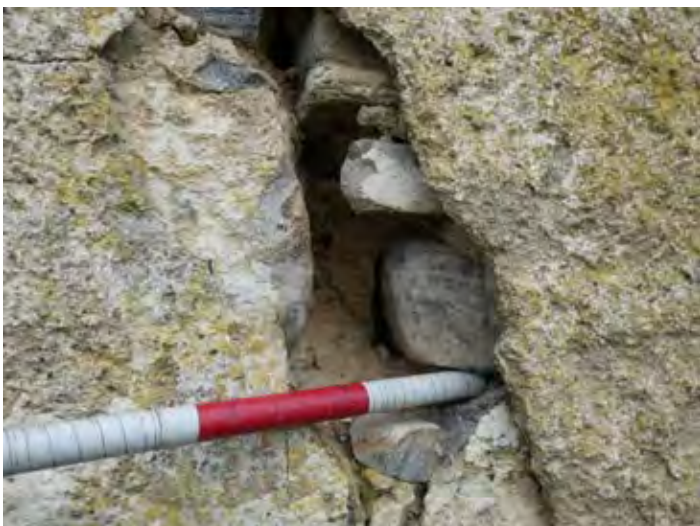
Figure 63.4. Detail of remnants of lime harl finish.
