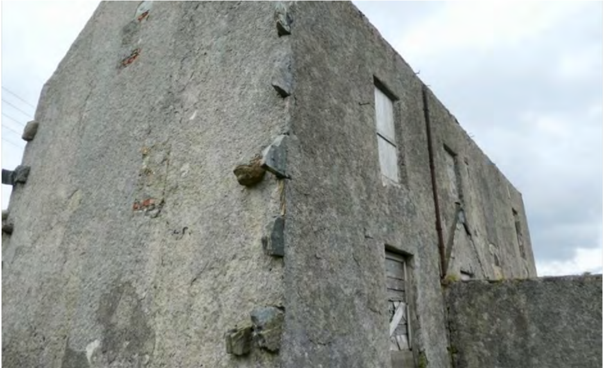
Figure 57.2. General view of the front and west elevation, showing the tusking for an unbuilt addition.
