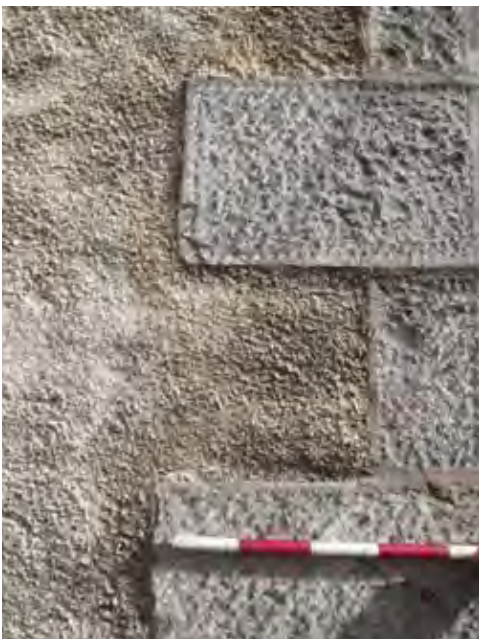
Figure 75.2. Detail of harl running up to the quoins.
