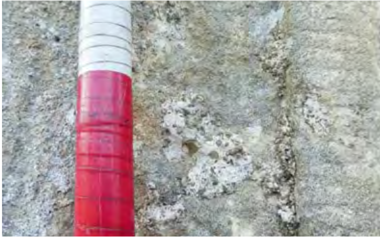
Figure 27.2. Area of remaining harl.
