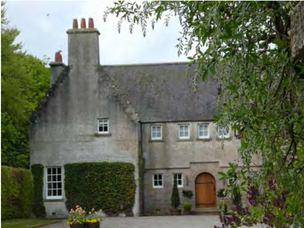
Figure 74.1. Front elevation of the house.
