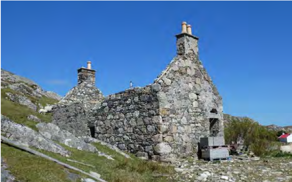
Figure 58.1. The west corner of the cottage at Groseby.
