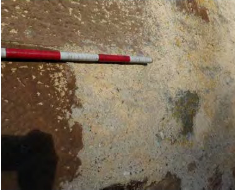
Figure 47.2. Detail of sandstone quoins.
