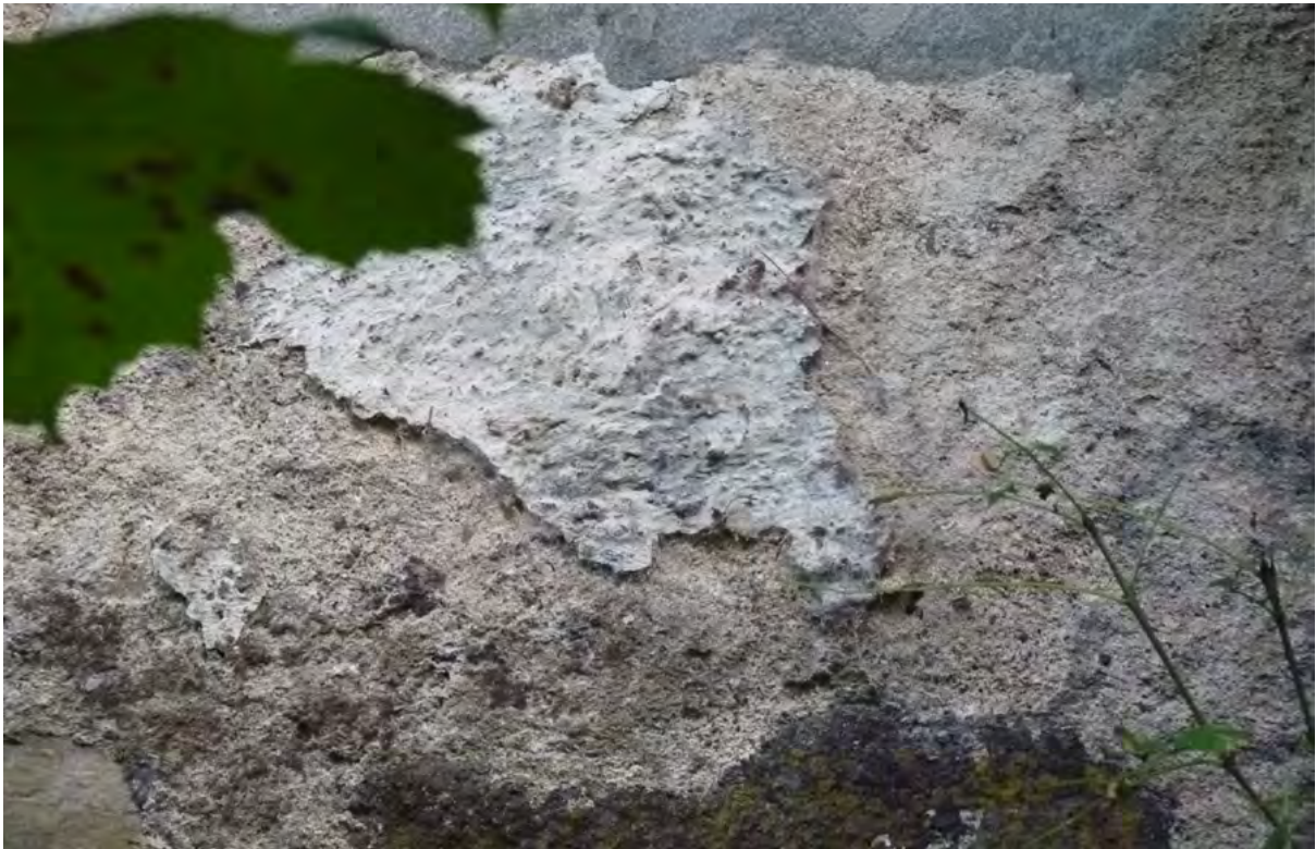
Figure 64.3. White limewashed harl to rear elevation.
