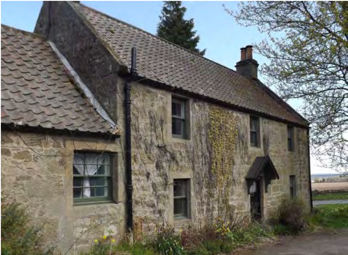
Figure 66.1. Front elevation of the cottage.
