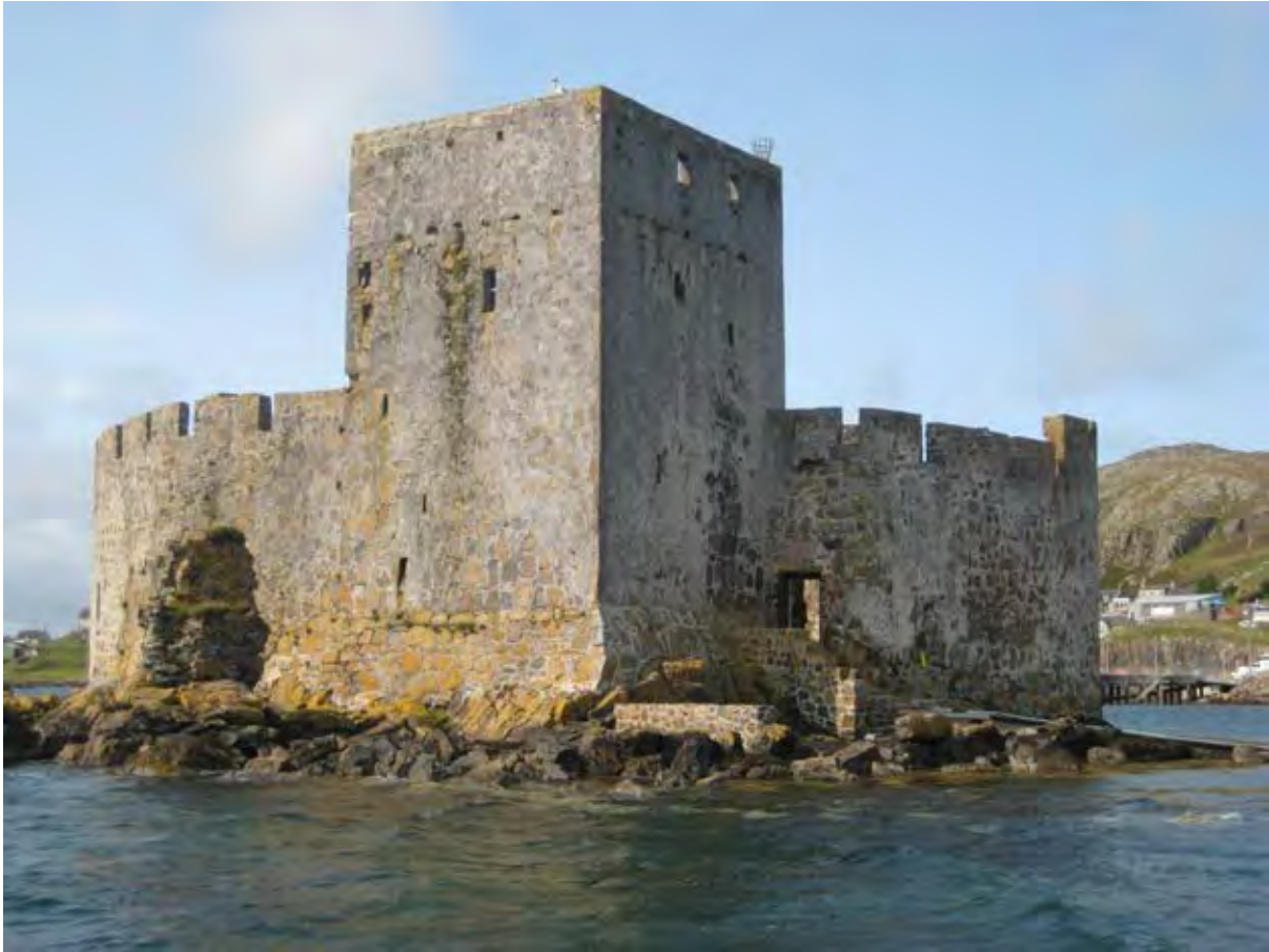
Figure 07.1. Kisimul Castle from the south east. The surviving historic harl is visible on the walls of the tower and the masonry of the curtain wall to the right.
