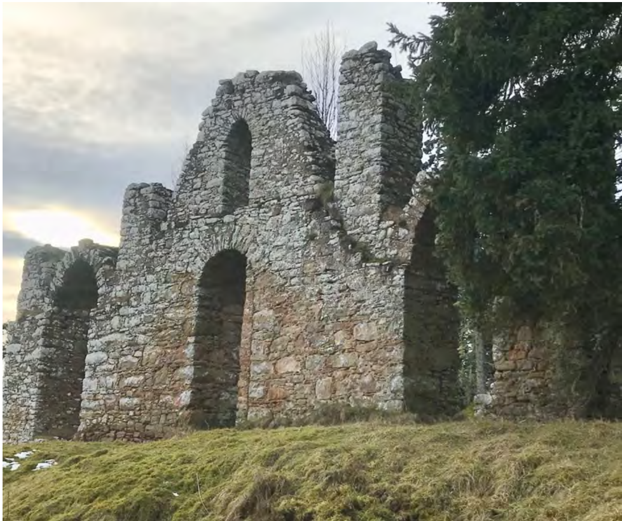
Figure 45.1. General view of the monument.
