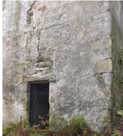
Figure 42.2. The east frontage showing well-preserved harl taken over the dressings and quoining.
