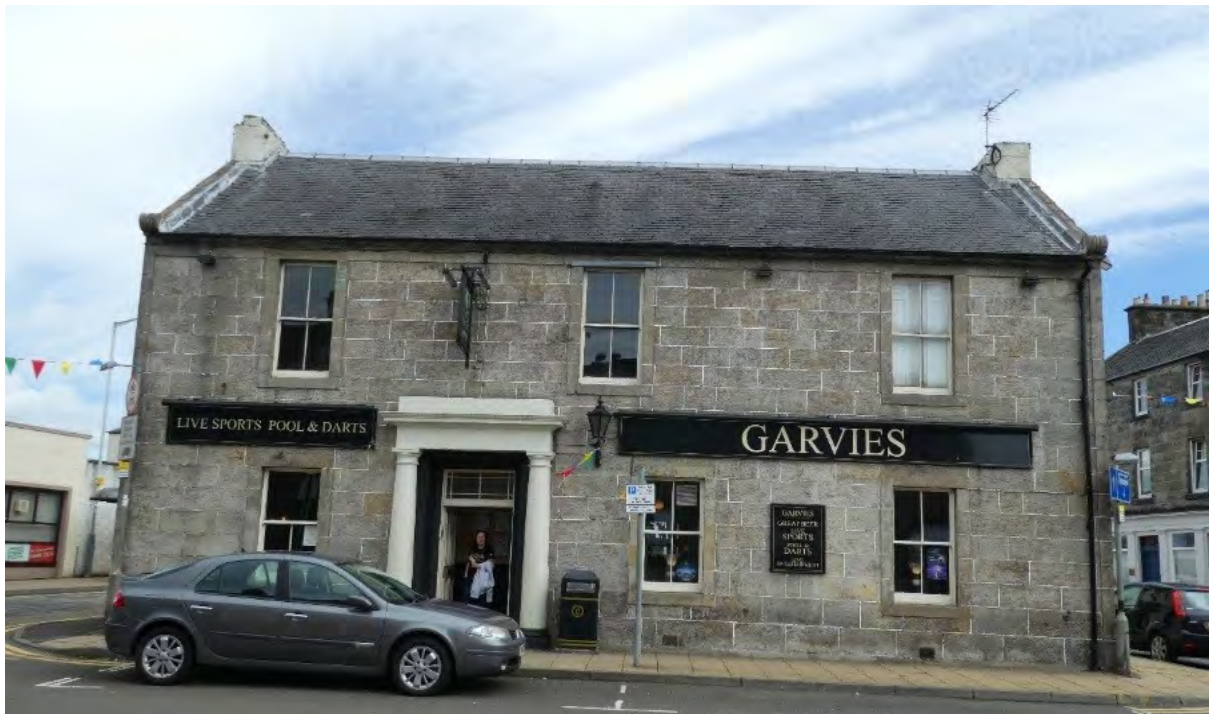
Figure 52.1. Front elevation of the inn.
