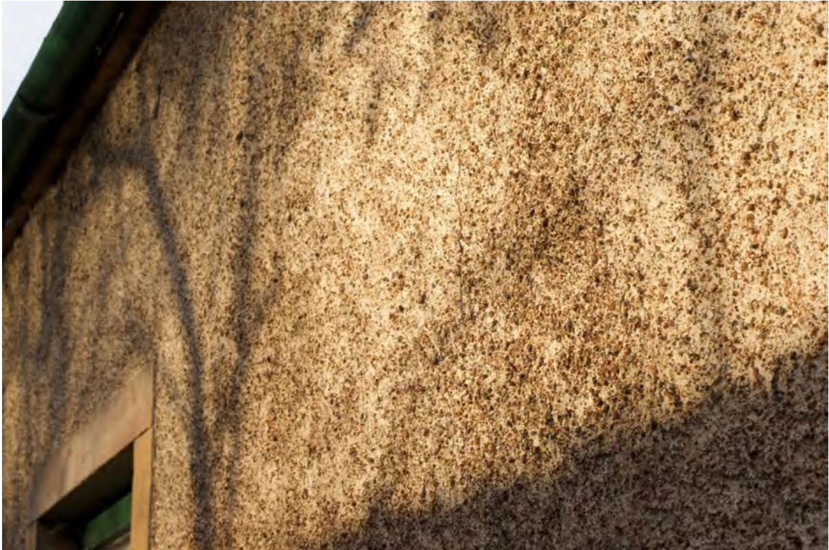
Figure 67.2. The complete lime harl in good condition on the front elevation.
