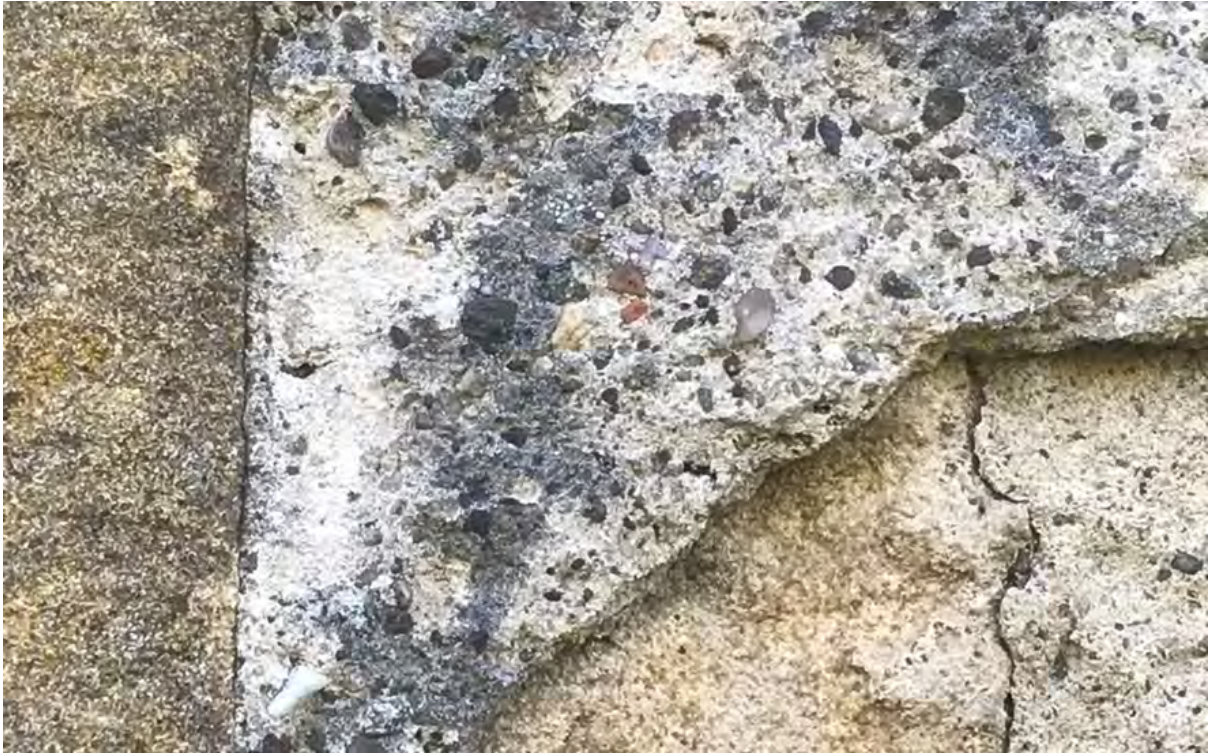
Figure 51.2. The thick single coat harl.
