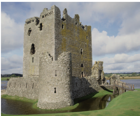
The great tower house at Threave was built in the 14th century, and the following century saw the addition of artillery defences encircling it. A typical gunloop pierces the angle-tower. © Crown copyright: Historic Scotland
