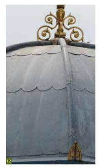
**Fig. 12** Decorative leadwork, such as this scalloped dome detail, can be replicated but is expensive.
