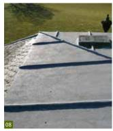
Fig. 5 Lead sheet on roofs can last for well over 200 years.
