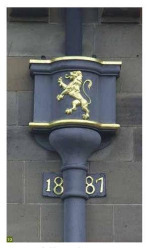
**Fig. 10** Decorative lead downpipe and hopper head.
