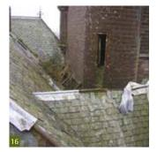
Fig. 14 Damage to stonework and other building elements is a common complication where lead is stolen.
