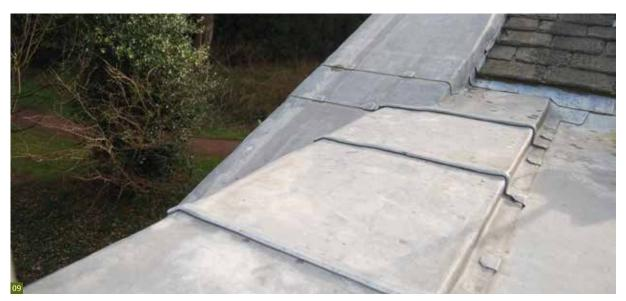
Fig. 9 Milled lead sheet.
