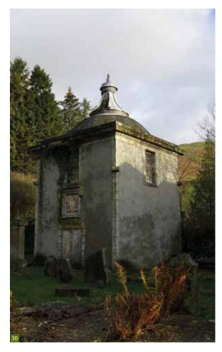
Fig. 30 Original lead detail, in poor condition and vulnerable.
