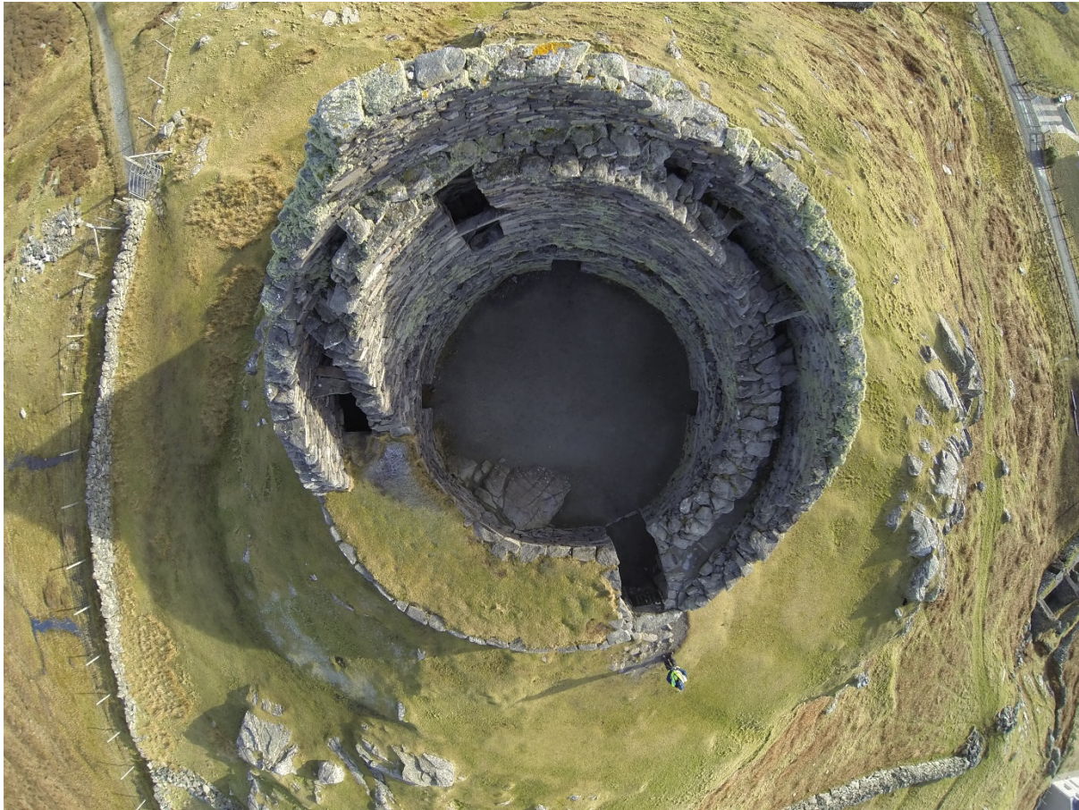
Figure 2: Dun Carloway close near-vertical aerial view showing hollow wall construction. © Historic Environment Scotland.
