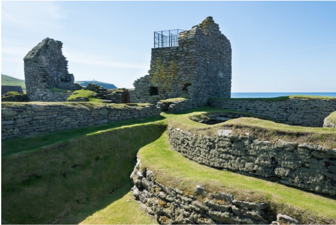
Laird's house (shows modern cast-iron viewing platform)
