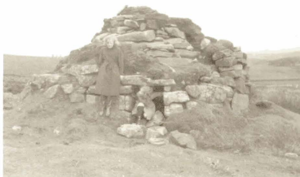
Illus 12 A corbelled stone shieling hut at Cnoc Dubh near Gearrannan in 1937 (photograph by EC Curwen, reproduced by kind permission of Mrs E Saville).
