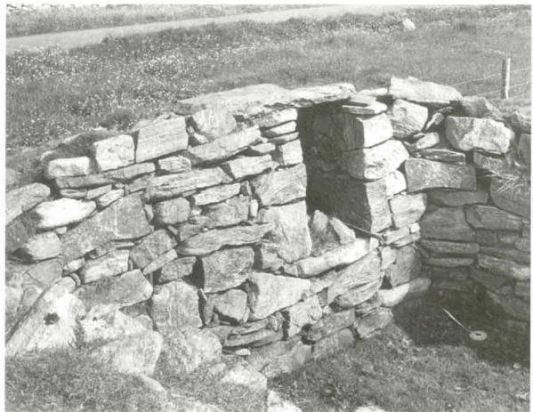
Illus 58 No. 39 A window inserted in the bedroom end of the building, from the interior (photograph by Headland Archaeology Ltd).
