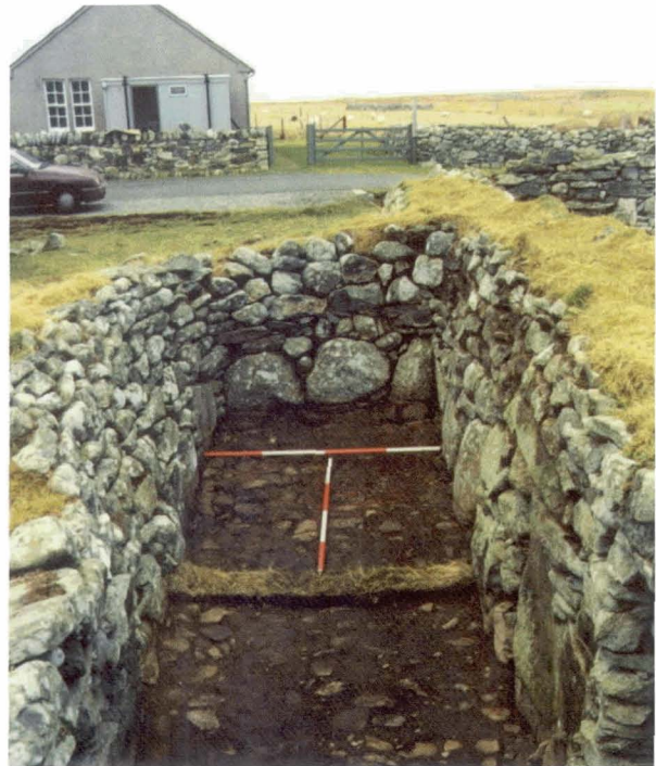
Illus 23 No. 39 Field boulder construction with an additional room abutting the byre/dwelling (photograph by Headland Archaeology Ltd).
