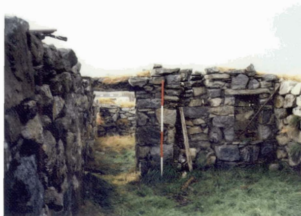
Illus 34 No. 10(ii) Partition with door, hearth and shelves (photograph by Headland Archaeology Ltd).
