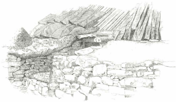
Illus 57 No. 42 Window to room exposed during the replacement of the roof and wall turves (© Chris McGregor).
