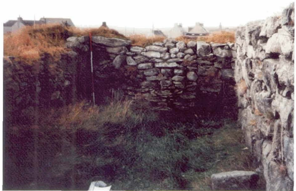
Illus 45 No. 10(i) A horse hole (toll each) blocked with smaller diameter stones (photograph by Headland Archaeology Ltd).
