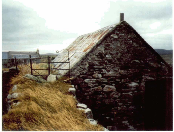
Illus 50 No. 10a Corrugated iron roof (photograph by Headland Archaeology Ltd).
