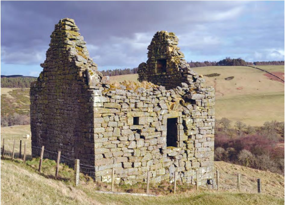
*Fig. 3 Mervinlaw Tower in the Scottish Borders dating from c.1600. Many ruins can appear to be drystone built, however in this case much of the clay mortar has simply been washed out.*
