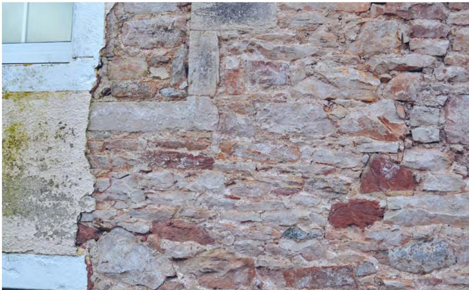
*Fig. 9 Dampness necessitated the removal of the cement render from this clay-bonded wall.*
