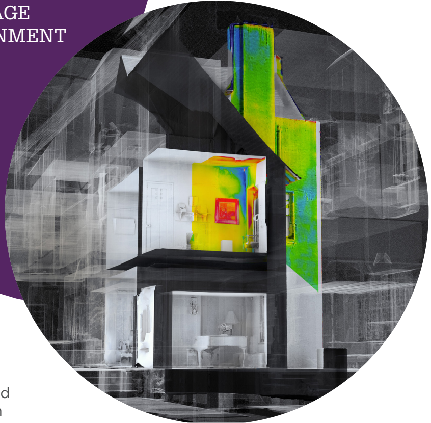
Thermal imaging combined with the 3D dataset highlighting areas of damp located on the South Column of the Hill House
