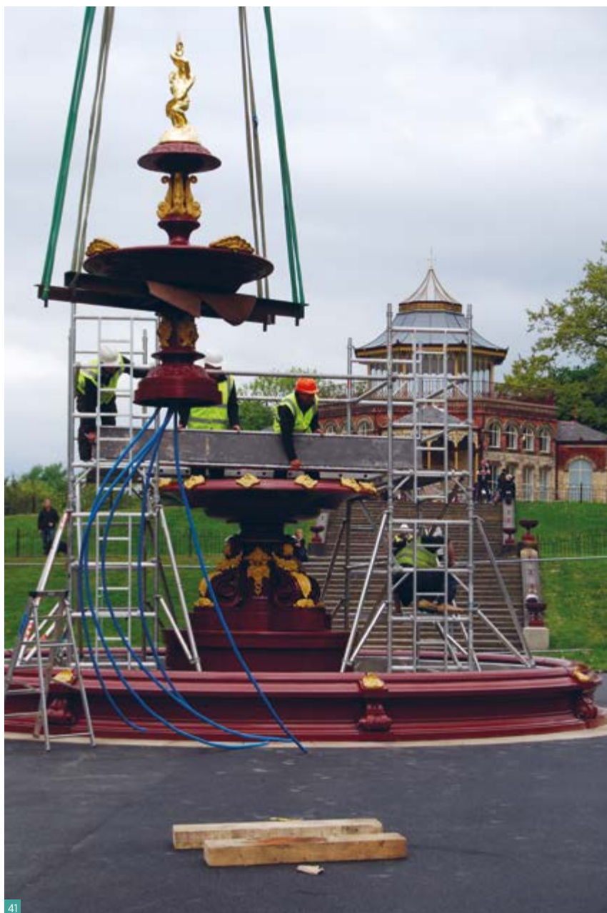
Fig. 41 Installation process and completed fountain at Mesnes park, Wigan.
