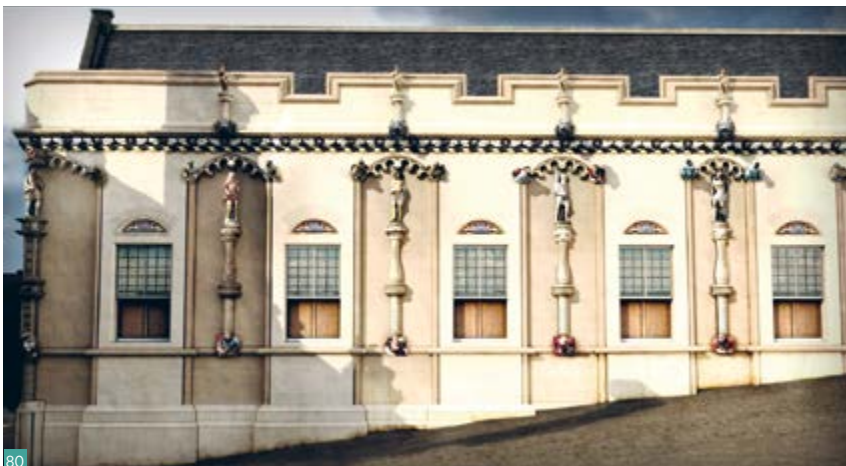
Fig. 80 Stirling Castle palace showing the lime harled façade with the painted Figs in context.
