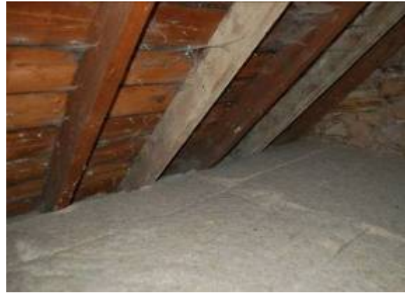
Fig. 5. Attic insulated with 270 mm flexible hemp batts
