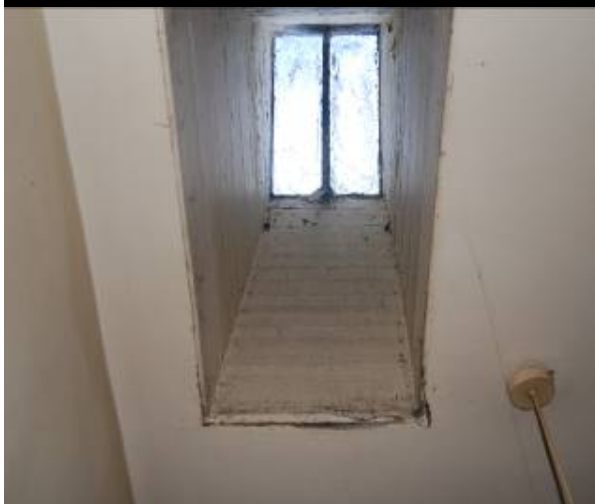
Fig. 8. The original iron rooflight was retained, but the glazing was replaced
