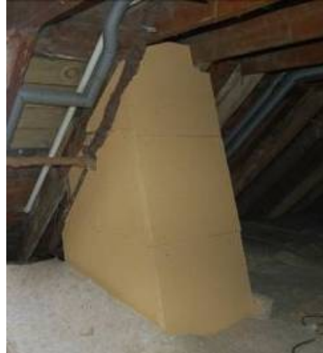
Fig. 9. The lightwell was insulated with wood fibreboard
