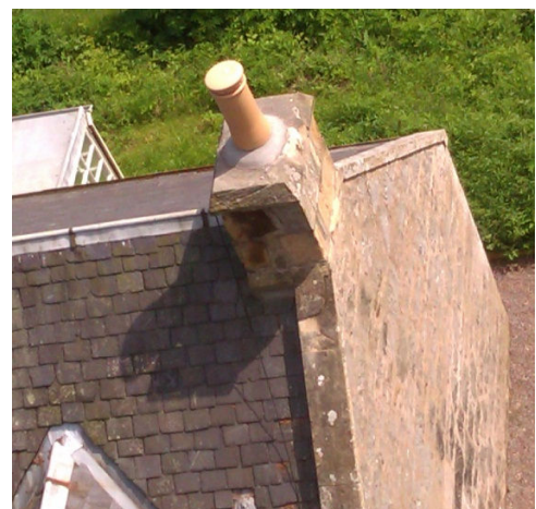
Photograph taken 26 June 2012, showing capping to flue from living room
