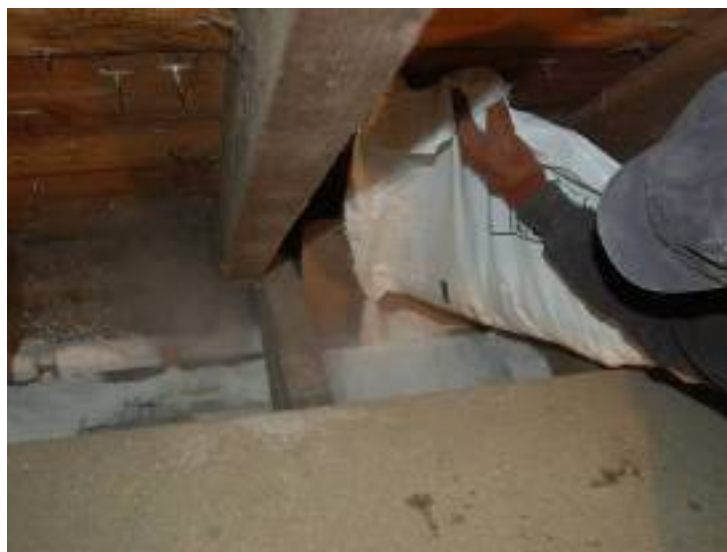
Fig. 15. Perlite insulation poured into wall voids from the attic space
