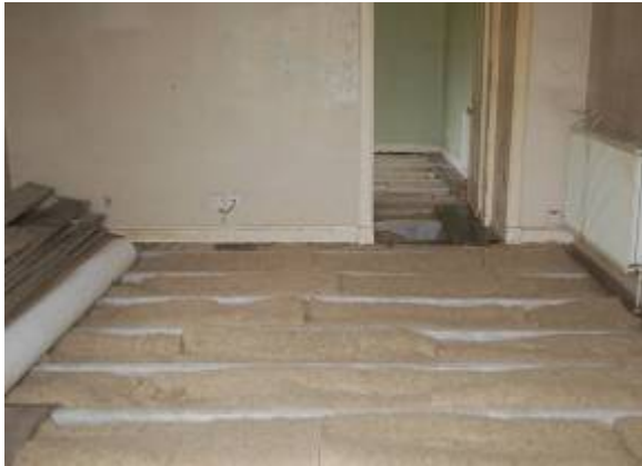
Fig. 13. Hemp insulation prior to re-laying floorboards
