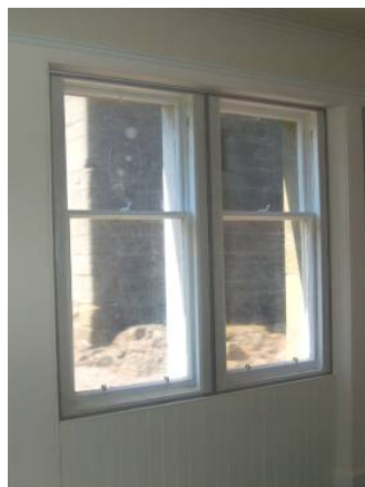
Fig. 10. The windows were fitted with polycarbonate secondary glazing
