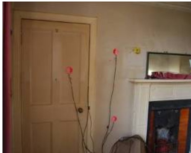
Fig. 2. The U-value of various elements being tested using heat-flux sensors
