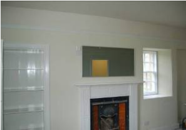
Fig. 19. The redecorated living room showing radiant heated mirror above fireplace
