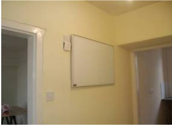
Fig. 21. Radiant heating panel in hallway
