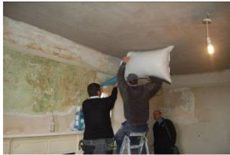
Fig. 16. Insulation being poured into the window reveals
