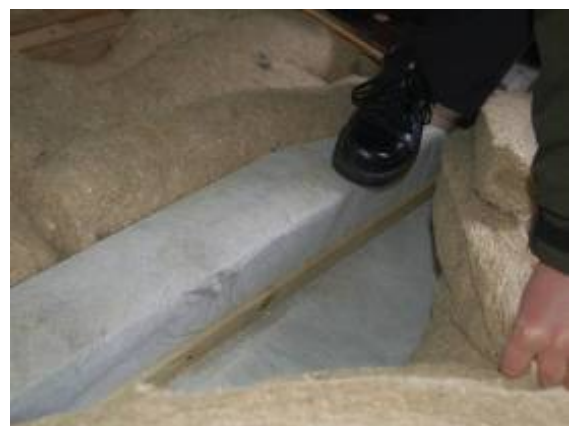
Fig. 12. The hemp batts were supported with a breather membrane
