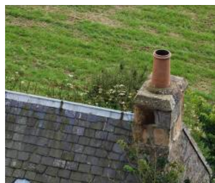
Fig. 18. The open chimney pot before refurbishment works
