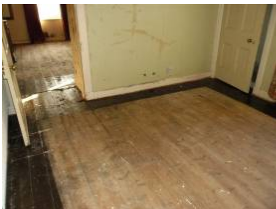
Fig. 11. Suspended timber floor showing 19 th century staining at edges
