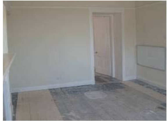
Fig. 14. Floor re-laid following insulation, showing areas of repair
