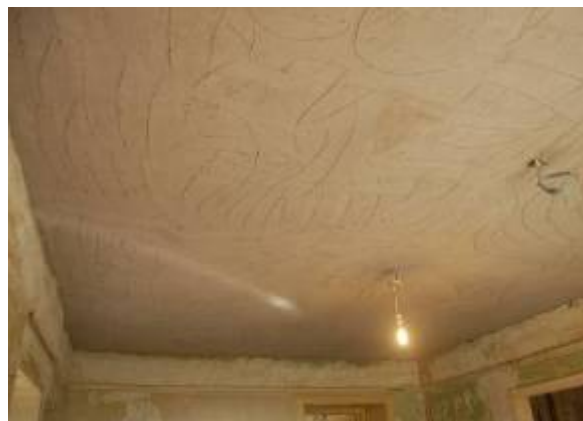
Fig. 7. The ceiling was repaired using haired lime plaster on lath
