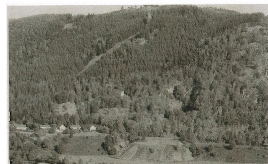
Plate 46 Overall view of the Newtyle Quarries as seen from Birnam Hill (NO045413)
