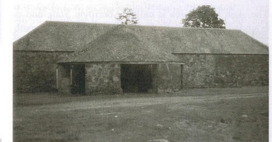
Plate 41 Horse Engine house on the Aberuchill Estate roofed with slates from the quarry
