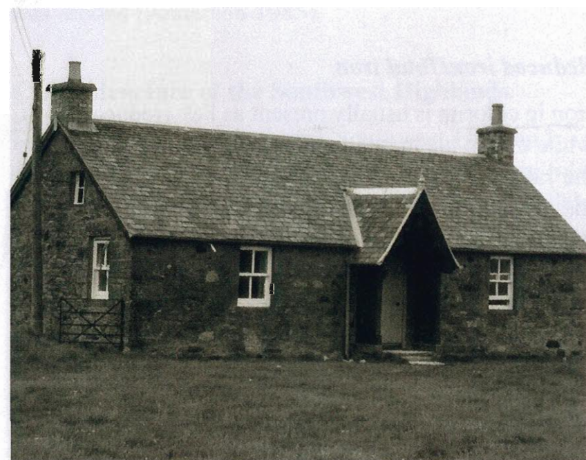
b) Bonellas Cottage has recently been re-roofed using the original slate with less than 10% wastage
