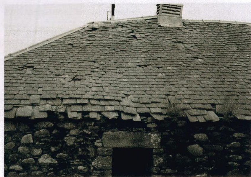
a) The barn at Frances Field (Kipney) is now suffering from nail sickness
