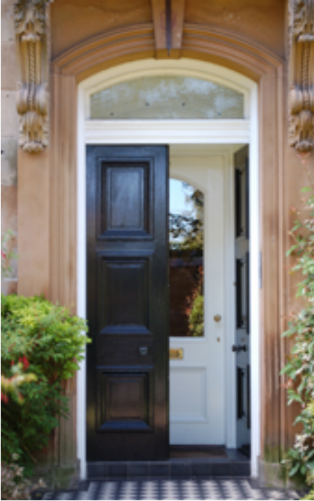
Fig. 2 Outer door opened to reveal vestibule.
