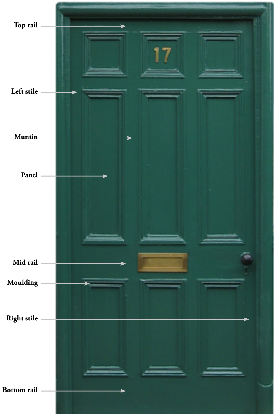
Fig. 3 The components of a traditional timber door.
