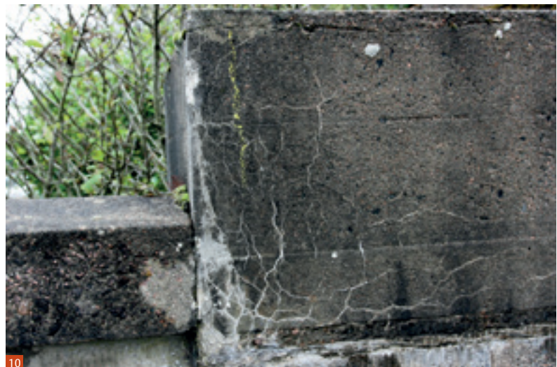
Fig. 10 Concrete deterioration as a result of chloride attack, bridge built c. 1937 (Category B-listed).
