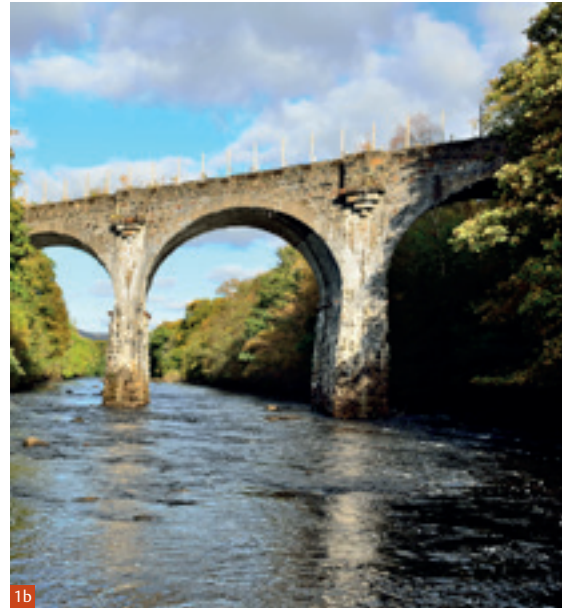
Fig.1a and Fig.1b Dochart Viaduct 1885-6, second oldest mass concrete viaduct in Britain (Category A-listed), © John Gray.
