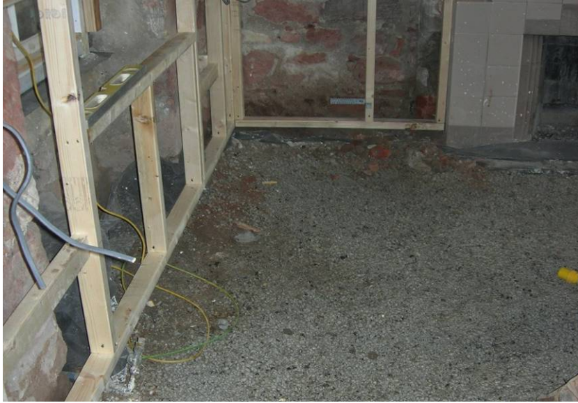
Fig. 11. The lime concrete layer in situ
