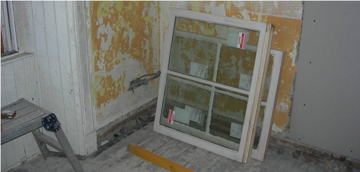
Fig. 14. New double glazed sash windows awaiting hanging
