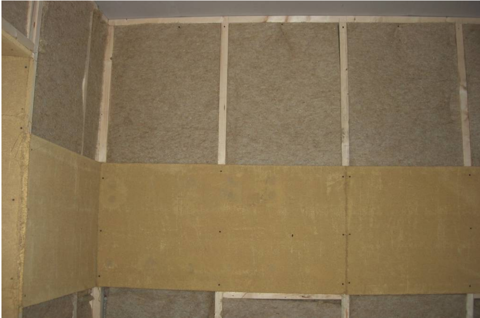
Fig. 5. Wood fibre insulation applied between timber straps with clay board being applied on top of this
