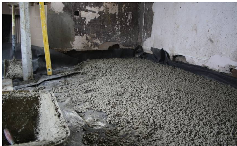
Fig. 10. The lime concrete screed being laid
