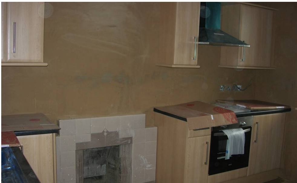
Fig. 6. The clay plastered walls with kitchen units in place
