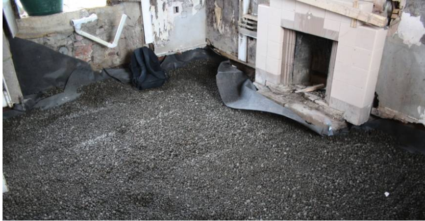
Fig. 8. The loose LECA laid down over a layer of geotextile
