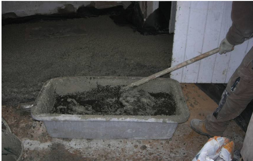
Fig. 9. The lime concrete being mixed using a traditional larry
