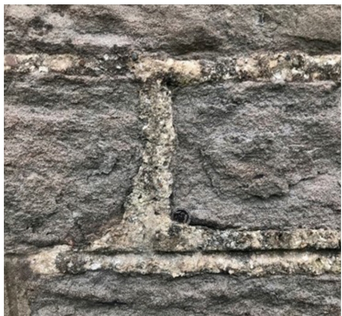
Figure 16 - Bridge of Allan. The weathered surface of bare stone with ruled out Victorian flush finishing, standing proud of the worn surface.
