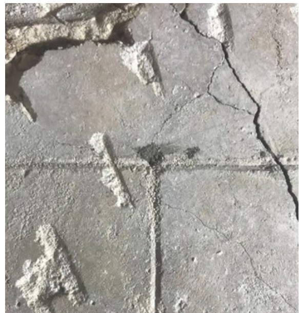
Figure 6 - Lined out external render at Newhailes House.
