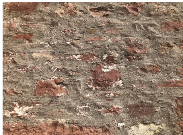
Figure 23 - A traditional type of finish, the flush point, using a more modern material, cement. The style is a fair repair of what was there before, but with a different material.
