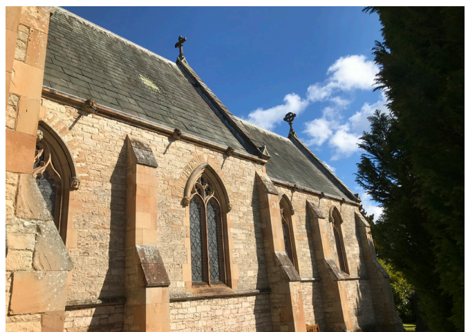
Figure 14 - The south elevation of St John's Episcopal Church, Jedburgh. A 19th century recreation of a pre-reformation church with many architectural details taken from the middle ages, except for the treatment of the masonry surface.
