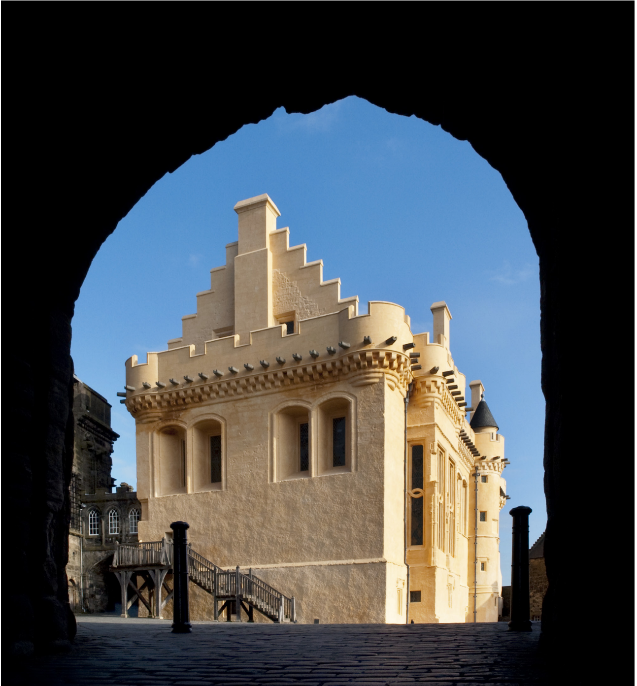
Figure 4 - The Great Hall at Stirling Castle; the limewash transforms the architectural appearance of the structure, highlighting the carved elements.
