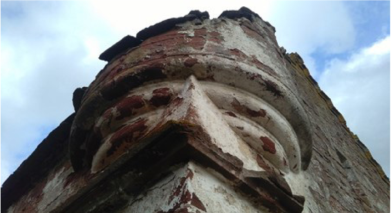
Figure 3 - Edzell Castle, limewash still adhering on a sheltered corner. This corner of the building represents a significant survival of an original coating. Image: Tom Addyman.
