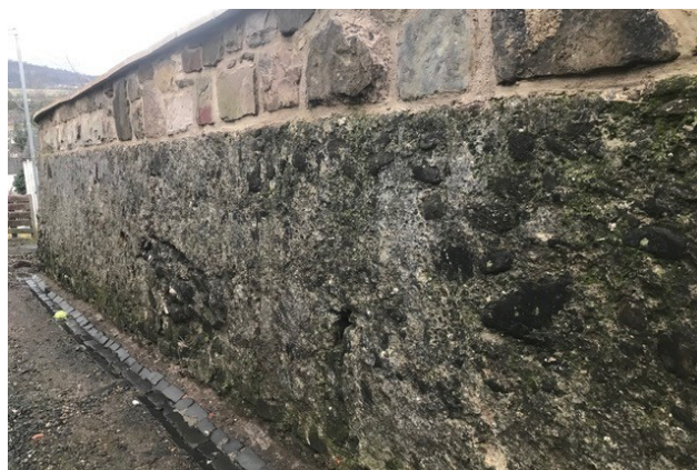
Figure 25 - A boundary wall in Stirling, probably dating from the early 19th century. The masonry finish on the raised section of the wall illustrates well the ambiguous approach to masonry finishes that this Technical Paper seeks to highlight.
