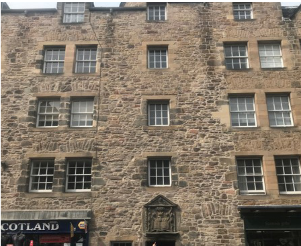
Figure 19 - ‘Bible Land’, 183-187, Canongate, Edinburgh, shown here with modern recessed pointing.
