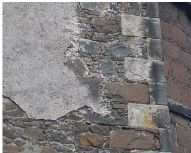
Figure 8 - A late 18th century building in Stirling showing harled rubble on the gable elevation, and more costly uncovered masonry work to the front. Note the harl fragment on the middle quoin.
