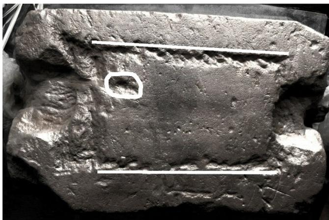
Figure 15 Roughly punched lines out of parallel. © Historic Environment Scotland.
