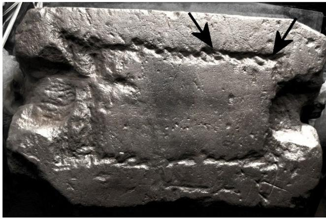
Figure 14 The neat start of cutting in for a sinking. © Historic Environment Scotland.
