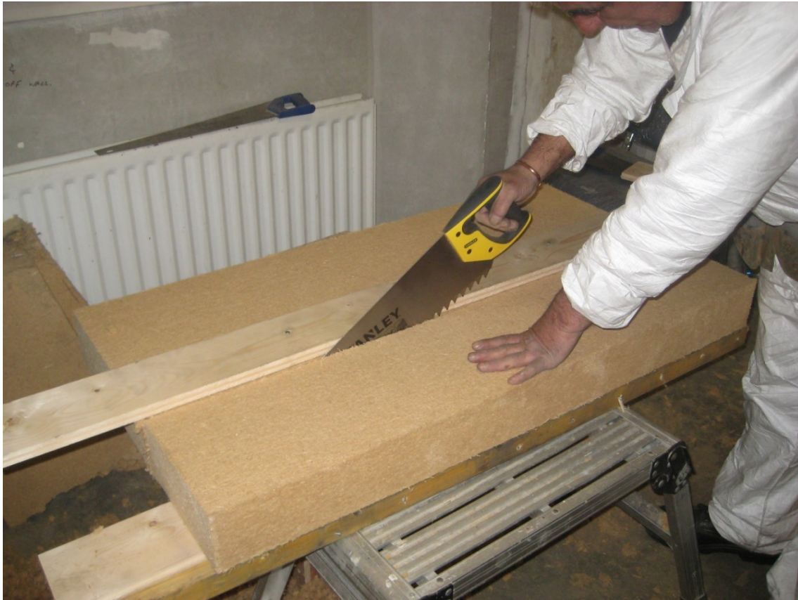
Figure 16. Cutting the wood-fibre board with a wide toothed hand saw.
