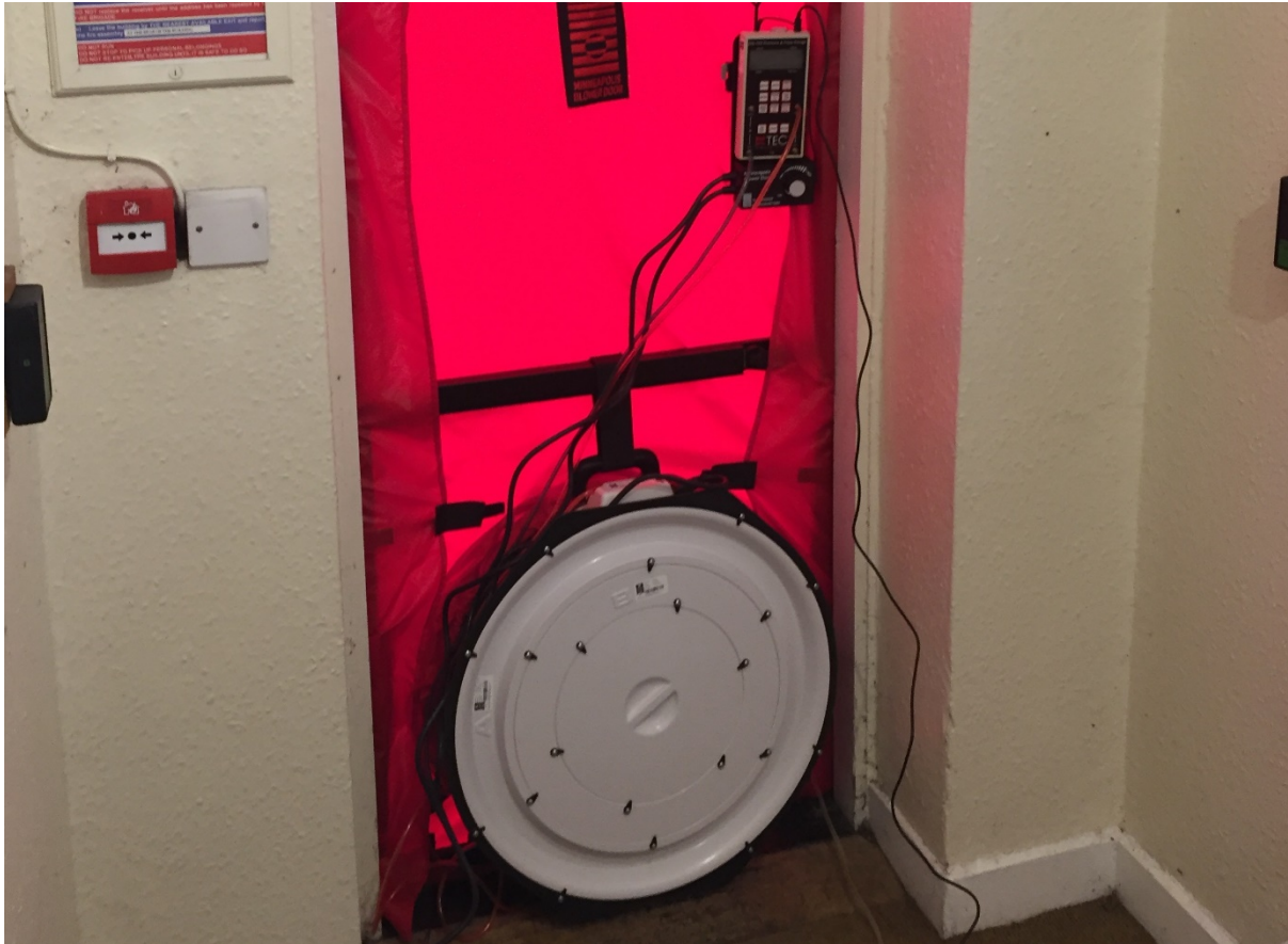
Figure 11. The fan on the back door for the air pressure test in Winter 2017.
