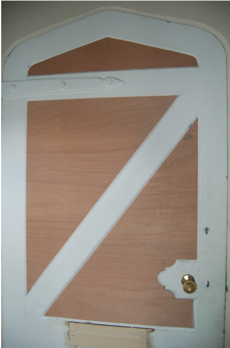
Figure 22. One of the ledged and braced doors at the lodge before being redecorated, showing the plywood panel on top of the aerogel board.
