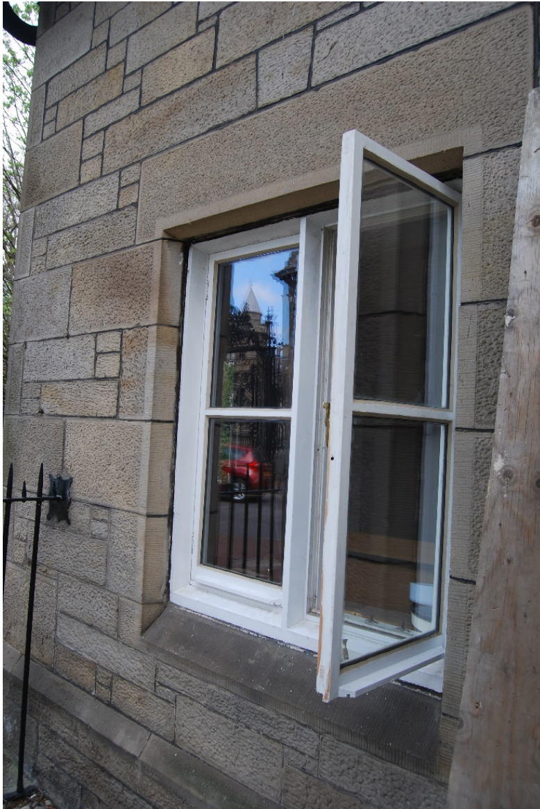
Figure 20. The new double-glazed units set into the existing casements.
