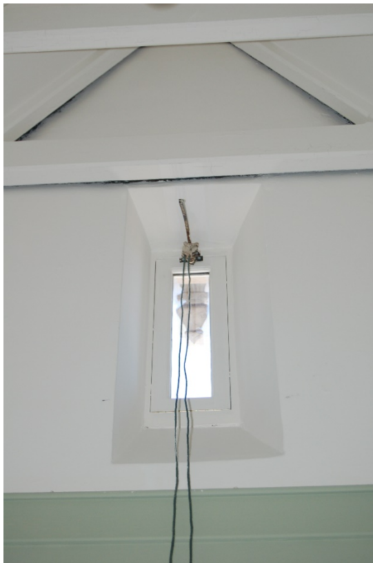
Figure 25. Internal view of the opening light.
