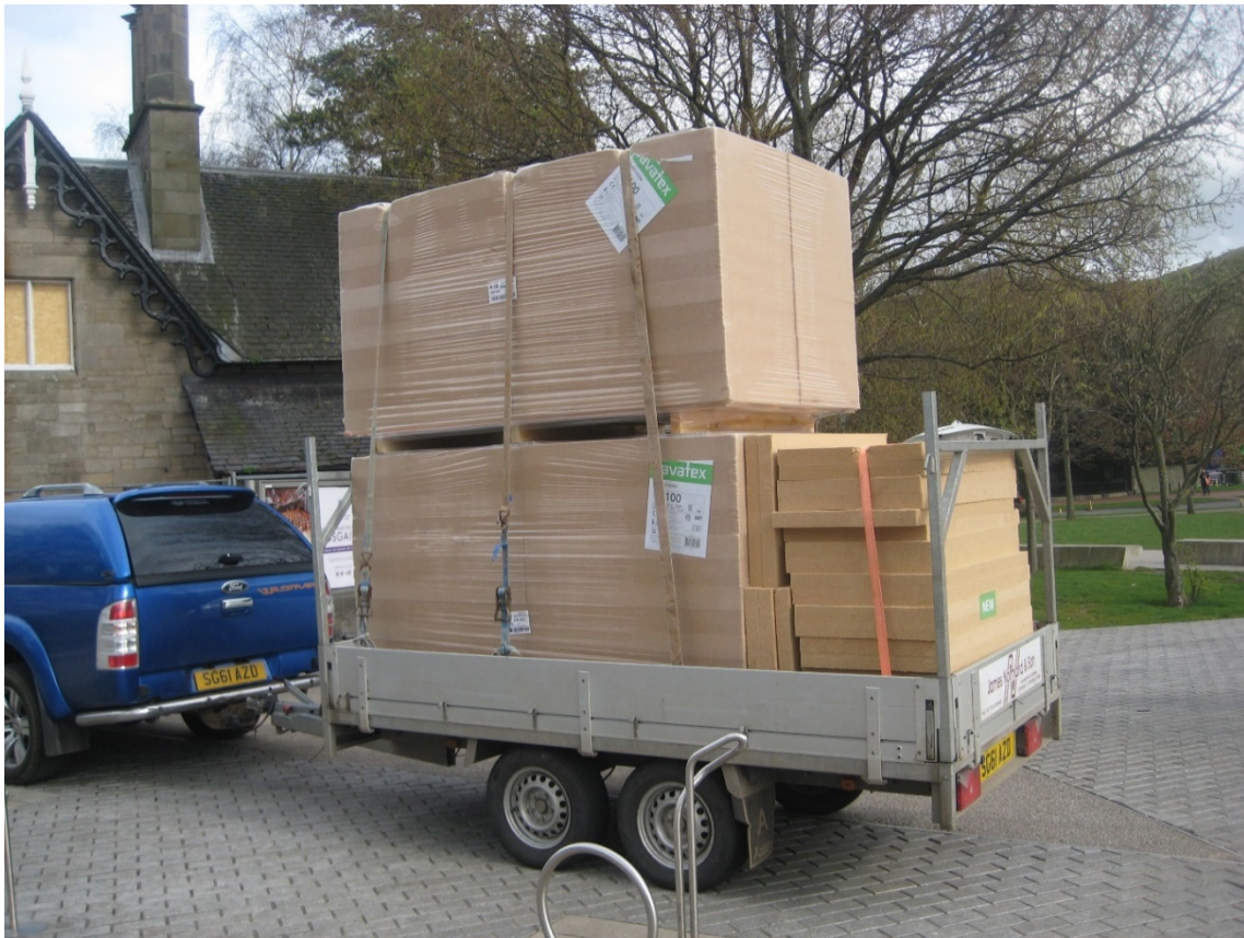
Figure 15. The wood-fibre insulation batts for use in the floor and the roof spaces.
