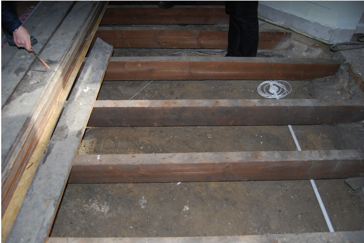
Figure 13. The cleaned-out floor void prior to the insulation being fitted.
