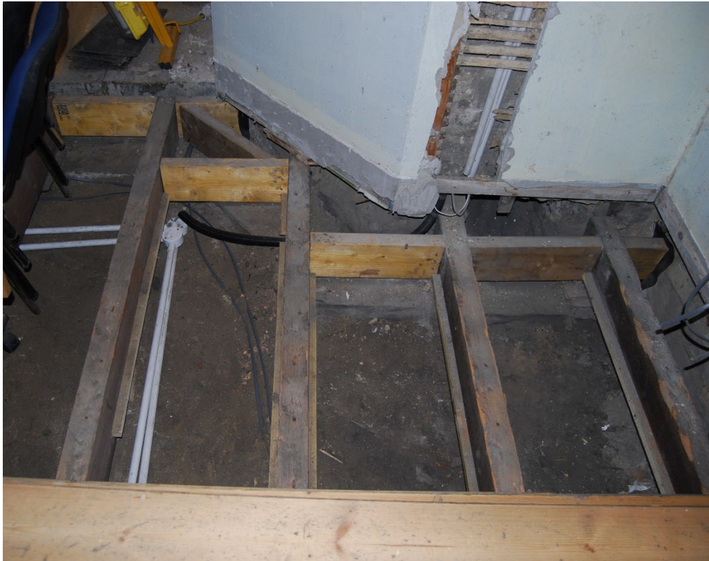
Figure 12. The additional stiffening put into the ground floor joists using 'dwangs'.
