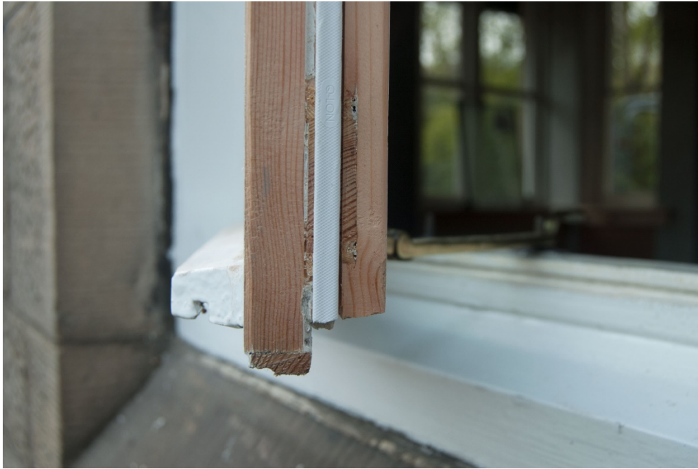
Figure 21. The cushion-type draught strip fitted to the casements.
