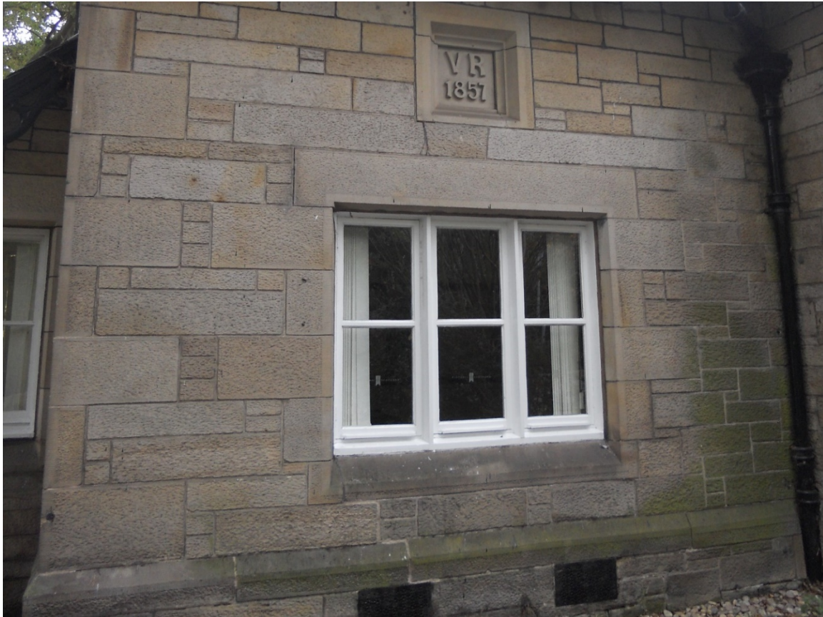
Figure 3. Single-glazed windows from the 1990s works.
