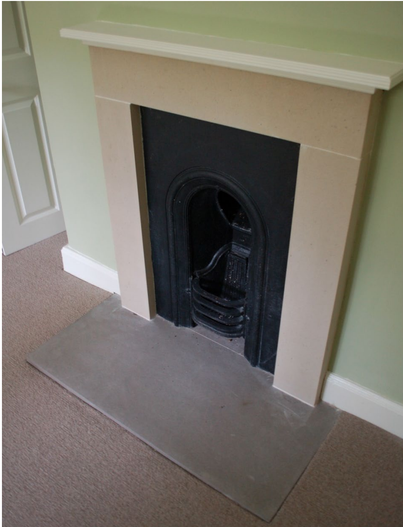
Figure 28. The re-instated chimney piece and hearth in the meeting room.
