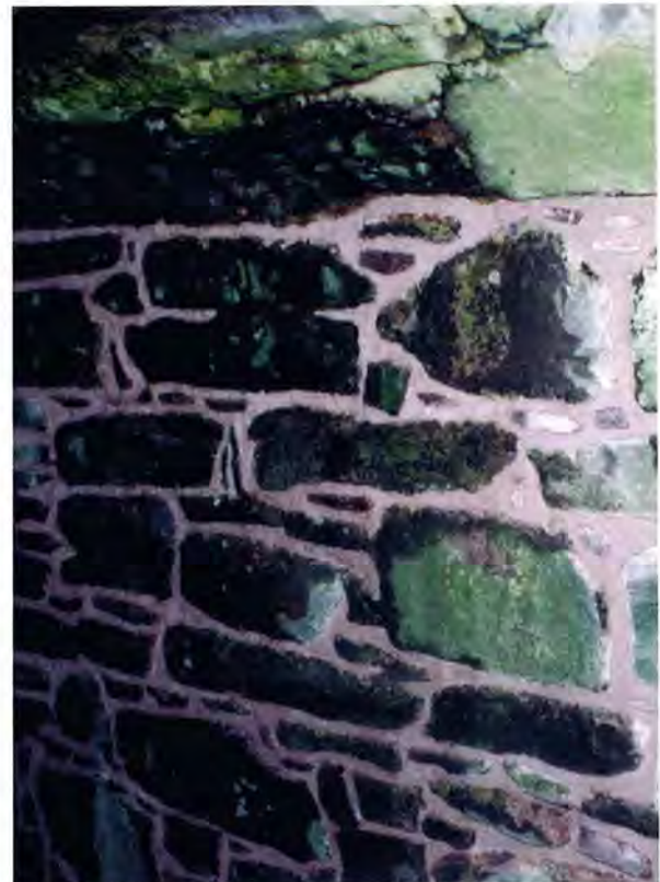
Figure 5.13: Doune Castle; external lime leaching on the left hand side and new lime repointing, slightly pink colour is becoming whiter by the uncarbonated lime transported on the surface on the right hand side.
