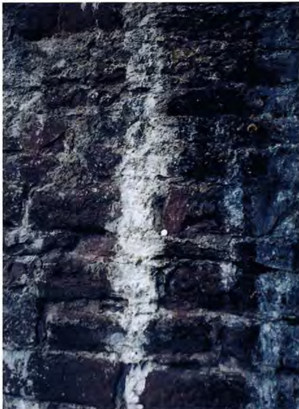
Figure 5.13: Doune Castle; external lime leaching on the left hand side and new lime repointing, slightly pink colour is becoming whiter by the uncarbonated lime transported on the surface on the right hand side.
