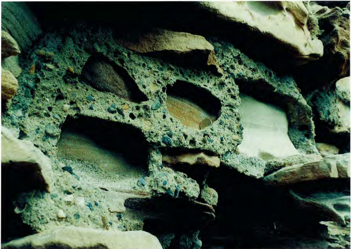
Figure 3.1: Tantallon Castle and detail of its deteriorated masonry. There are many historic buildings with repointed masonry, which have undergone some preservation treatment that resulted in a loss of original pointing and bedding mortar. For example Tantallon Castle with its 4m thick, red sandstone ashlar curtain walls which were repointed and consolidated before the Second World War. The appropriateness of this kind of intervention may be questioned. However, the work was done with the best knowledge and skills of that time. On the other hand, how much of the original mortar was there when it was treated? Pointing mortar is often the first to deteriorate so repointing has been a common practice in building maintenance in the past. The compatibility of such treatments and application of traditional techniques should be considered.
