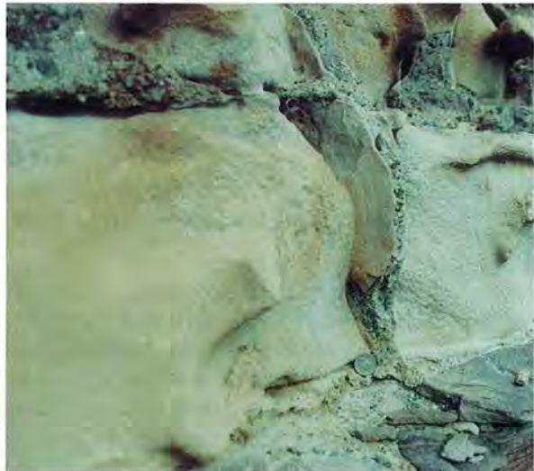
Figure 5.4: Is this mortar compatible with masonry? Cement-based mortar is a good binder and can locally support the adjacent stone to mortar joint. However, the masonry still weathers and its appearance is changing. The mortar in joints is protruding and visually expanding but stones are diminishing.
