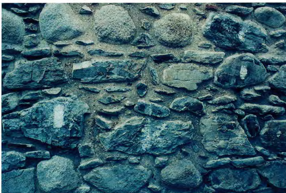
Bottom: Trial panel of repointing at Inverlochy Castle.
