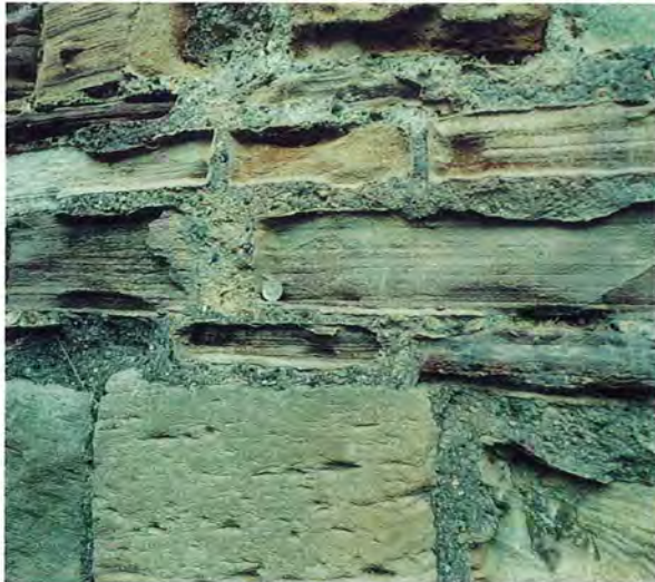
Figure 5.4: Is this mortar compatible with masonry? Cement-based mortar is a good binder and can locally support the adjacent stone to mortar joint. However, the masonry still weathers and its appearance is changing. The mortar in joints is protruding and visually expanding but stones are diminishing.
