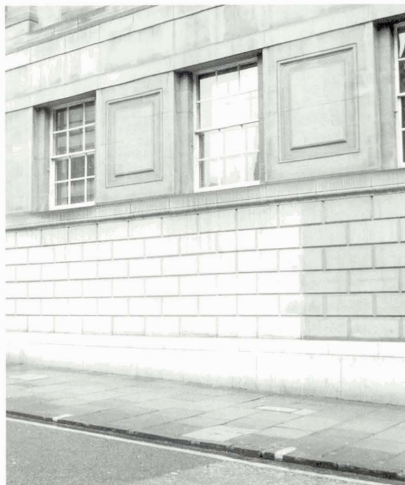
Illustration 6. Part cleaning of a sandstone façade.
