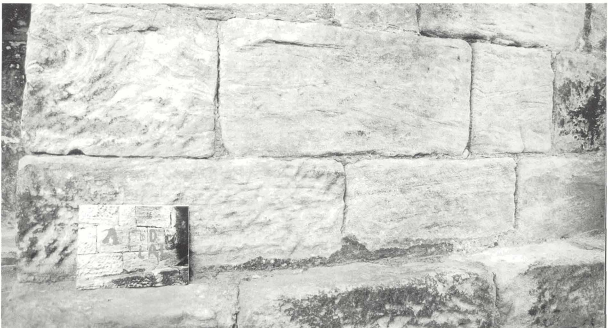
Illustration 8. Graffiti removed from an historic sandstone surface. The inset photograph shows the graffiti before removal. Complete removal was not attempted and some residual paint remains after cleaning. (Crookston Castle)
