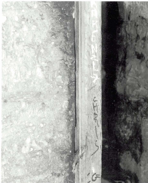
Illustration 20. Graffiti on an original timber door frame in a castle. Note also the scratches and gouges on the timber.
