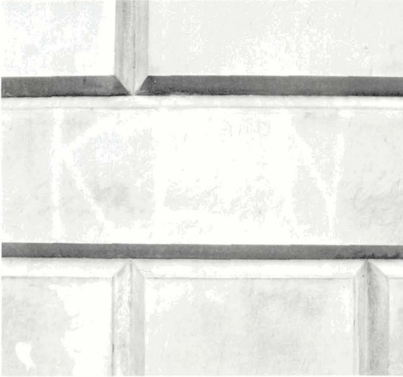
Illustration 7. Graffiti cleaned from soiled sandstone around 30 years previously.
