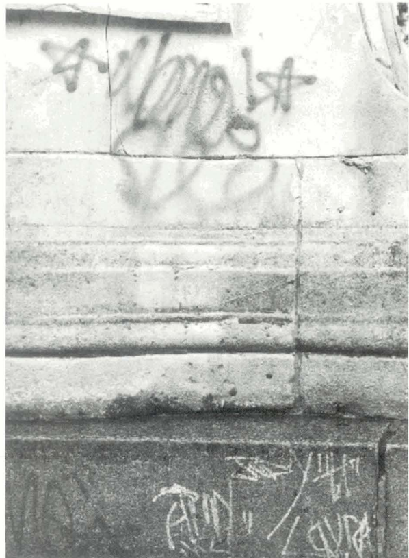
Illustration 11. Graffiti attack on limestone and granite monument. Note the greater variety of graffiti marker types used on the granite.
