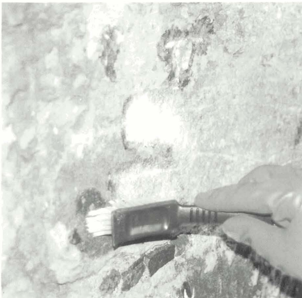
Illustration 29. Gentle agitation of gel and dissolved graffiti paint with a nylon brush.
