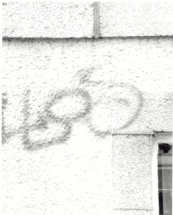
Illustration 17. Aerosol spray-paint on harled surface of a listed building. Removing the graffiti in this case is made more difficult by the continuation of the graffiti onto the granite window margin.
