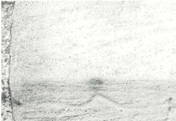
Illustration 10. Graffiti removal from sandstone showing loss of iron-rich minerals and 'bleaching' of the surface.
