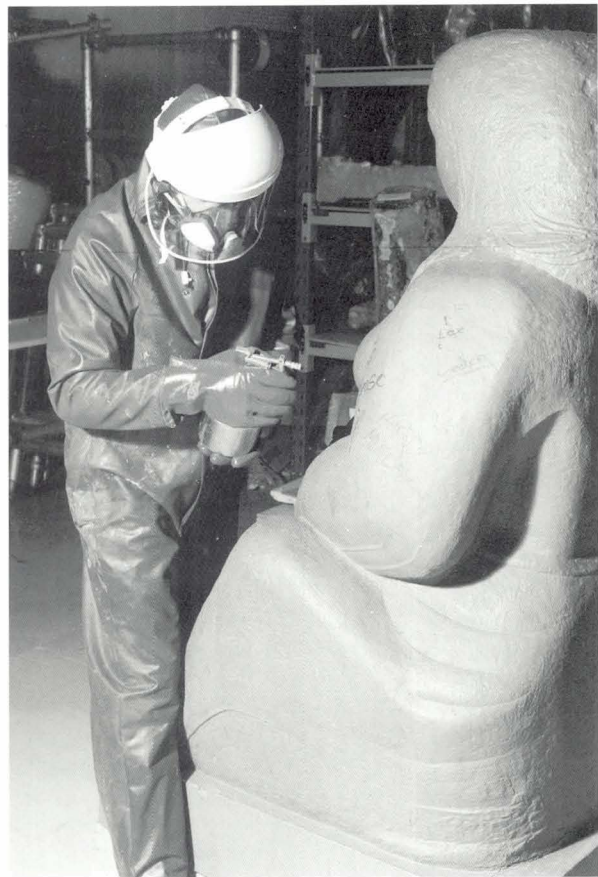
Illustration 36: Fully protected operative removing graffiti from a carved figure.
