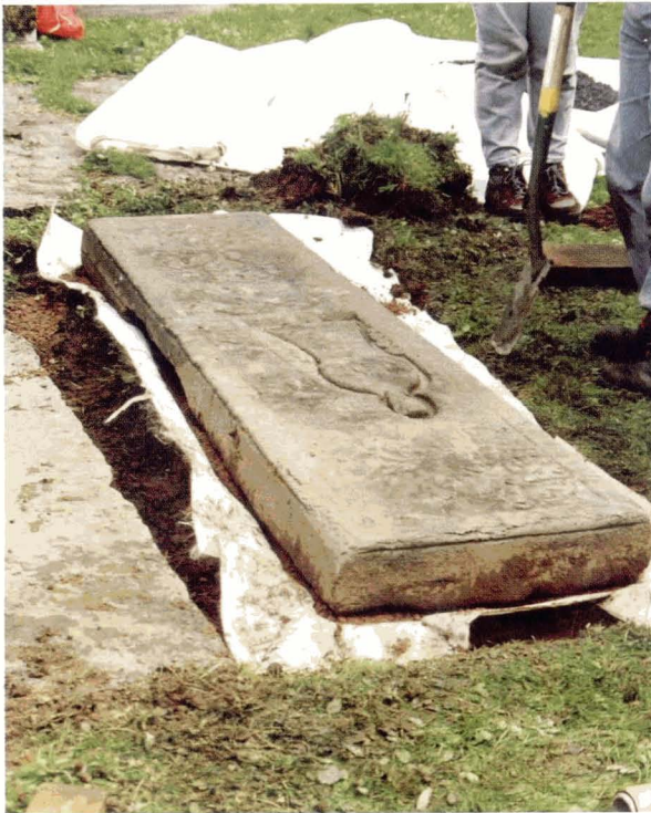
128. Slab on sand bed with textile based membrane
