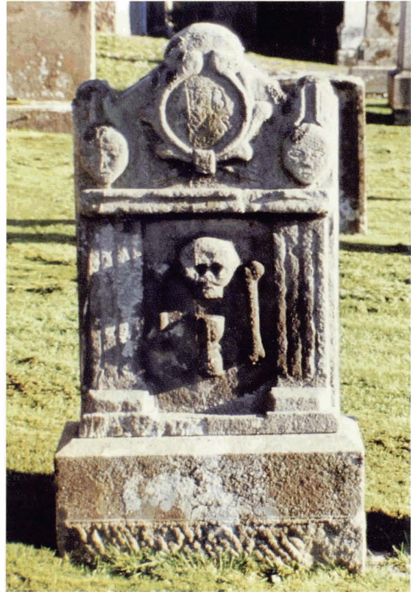
112. The potential to damage these historic gravestones by careless grass cutting is clear. In such cases hand trimming around the stones is recommended
