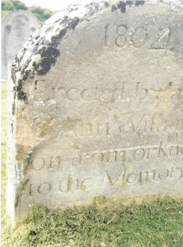
111. Historic headstone with arris damaged by grass-cutting equipment
