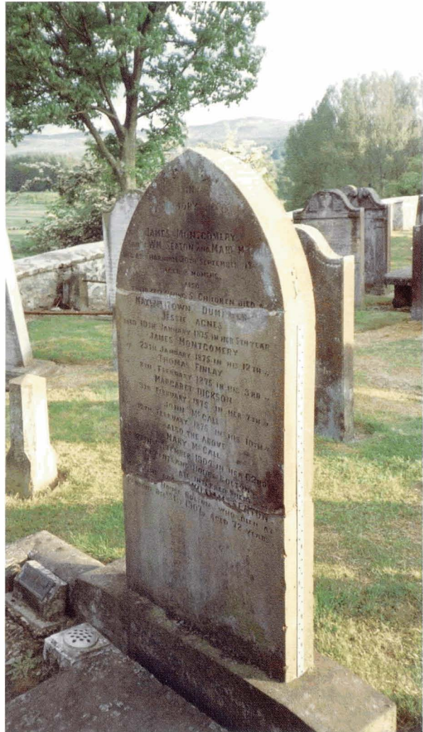
75. Headstone repaired with mortar. The galvanised strap fixed to the edge of the slab will add little to the stability of the repair
