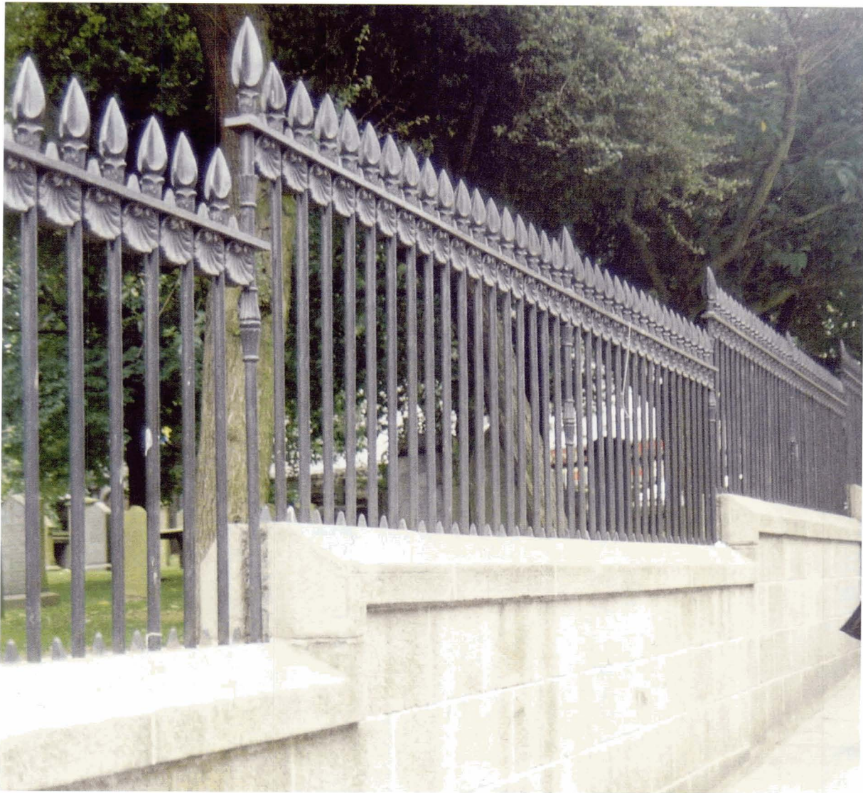
82. Well-maintained cast iron railings at St Nicholas Kirkyard, Aberdeen
