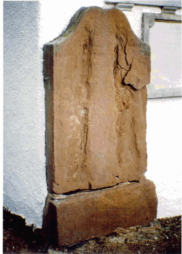
45. Stone erosion reflecting water run-off patterns
