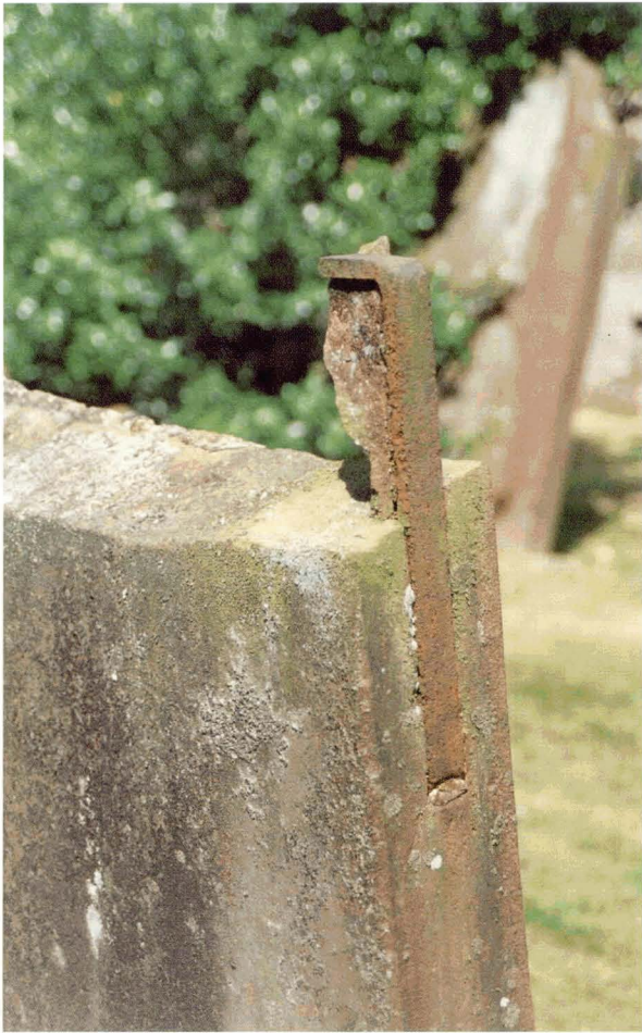
73. An iron cramp has been used to repair the headstone. A volume expansion of the cramp due to corrosion has caused the stone to fracture and increase the scale of the damage
