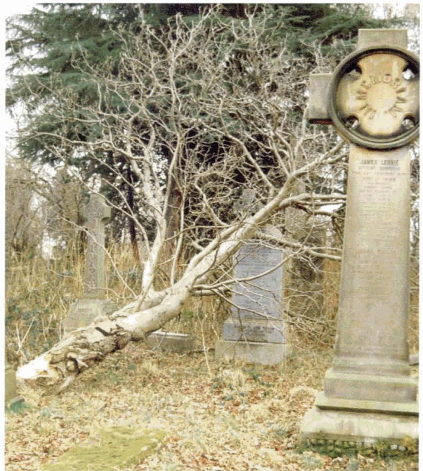
105. Fallen tree causing damage to headstones. This tree should have been carefully removed before it was allowed to collapse and cause damage to headstones
