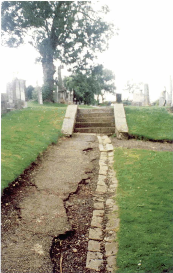
115. Inadequate design of the path to accommodate surface water run-off has resulted in disruption of the tarmac. In this case the use of tarmac has increased maintenance problems and is inappropriate in a graveyard setting of this type
