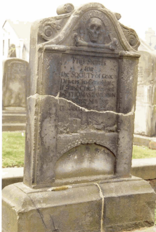
68. Snapped headstone repair with lime mortar joint
