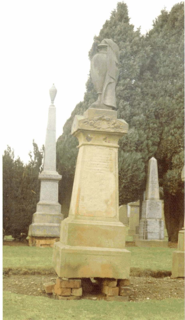
114. Significant erosion, as a result of turf removal, has led to this memorial becoming dangerously unstable
