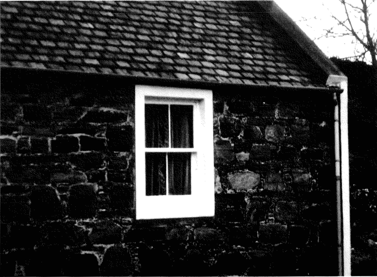
4. Original lime pointing and pinning stones.
