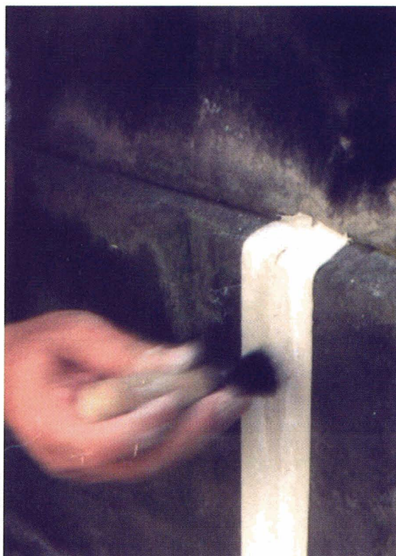
25. Tamping the mortar firmly back with a bristle brush.
