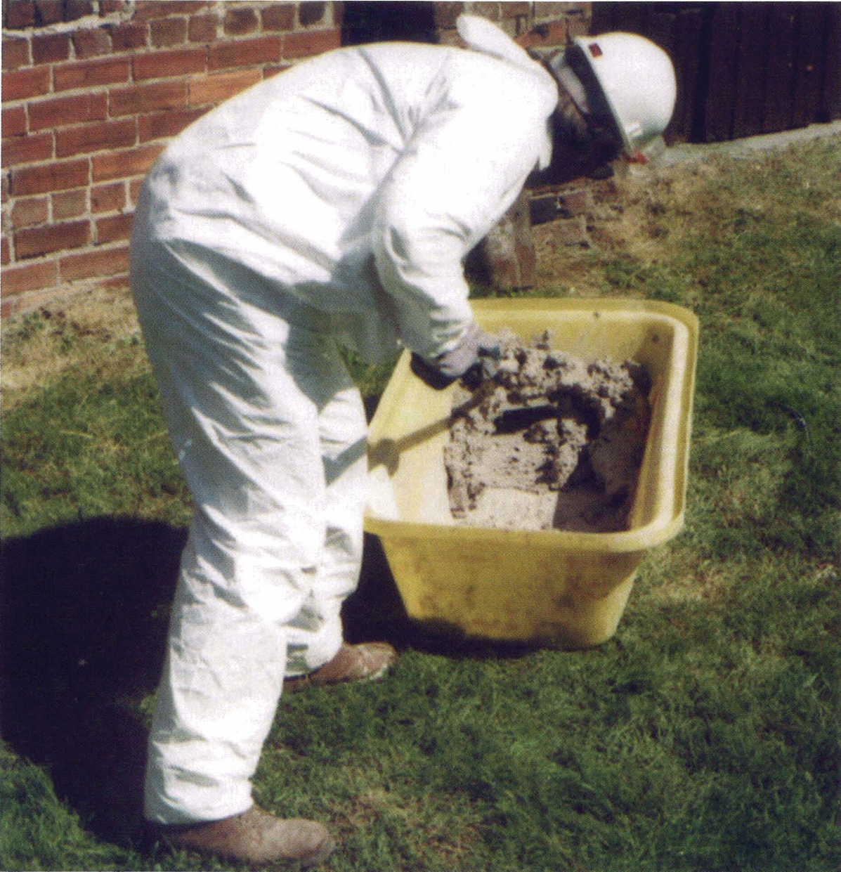
14. Knocking up mortar by hand using drag hoe.
