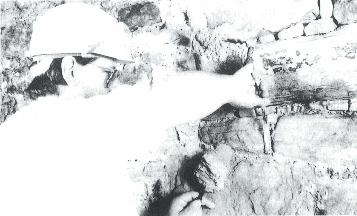
20. Repointing rubble masonry.
