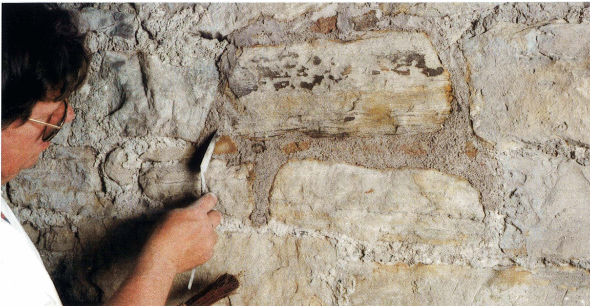
21. Finishing the surface of mortar joints using a small tool.
