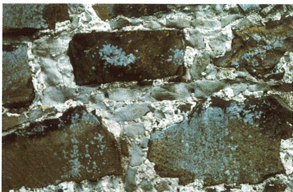
17. Closely packed sandstone pinnings in a whinstone rubble wall.
