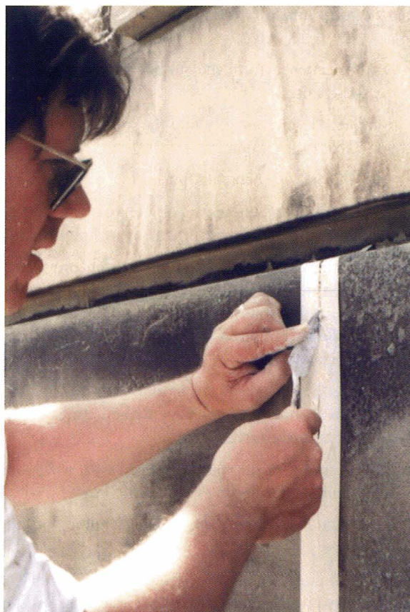
24. Pressing mortar into a fine ashlar joint protected by masking tape.
