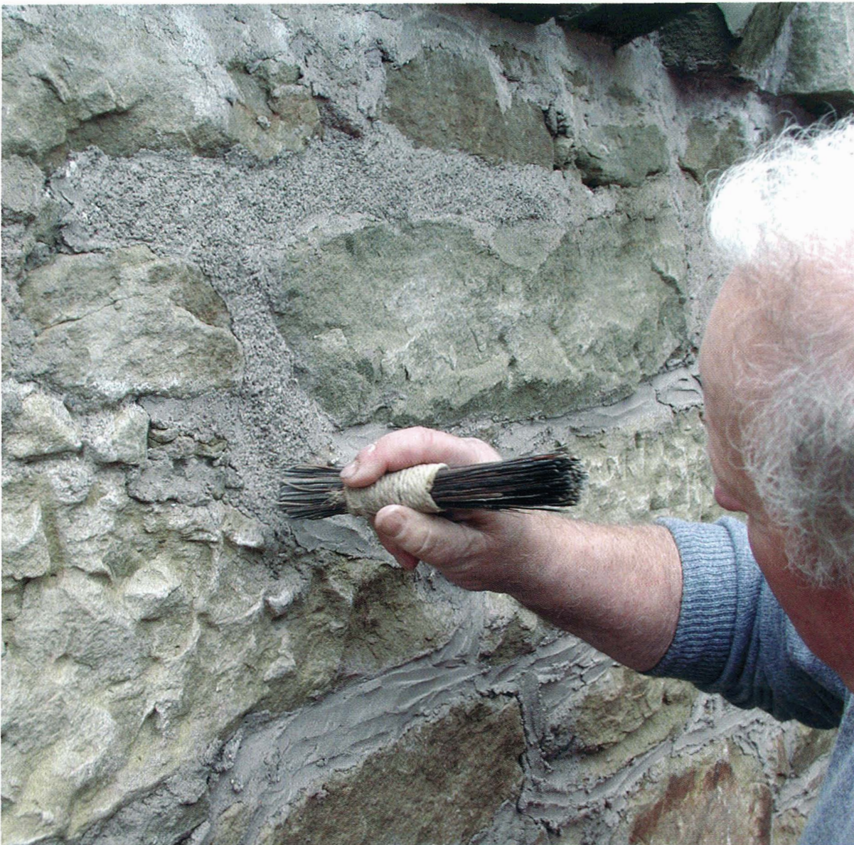
6. Faired-out lime pointing with good open texture
