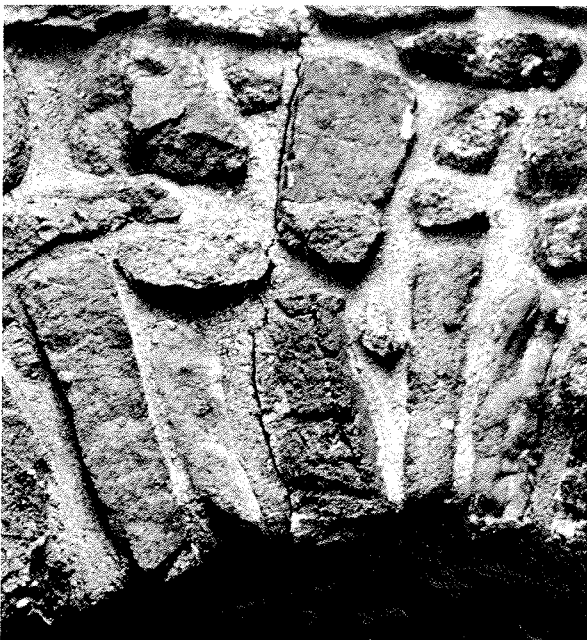
2. Movement joint in old masonry consolidated in cement-based mortar.
