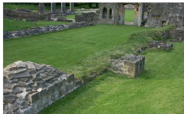
Fig. 2.6: Hailes Abbey, Gloucestershire, England. Although they obscure the covered surface, soft cappings protect masonry from thermal cracking, leaching of soluble minerals, frost and mechanical damage. Though the core construction of the capped walls cannot be read, their form is clear as a result of the sites closely mown lawns.
