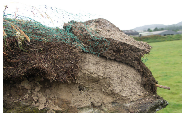
Fig. 2.14: Black Castle of Moulin, Perthshire (CS13). Locally at an exposed end, the turf has died and clay dried out, though with only minor cracking.
