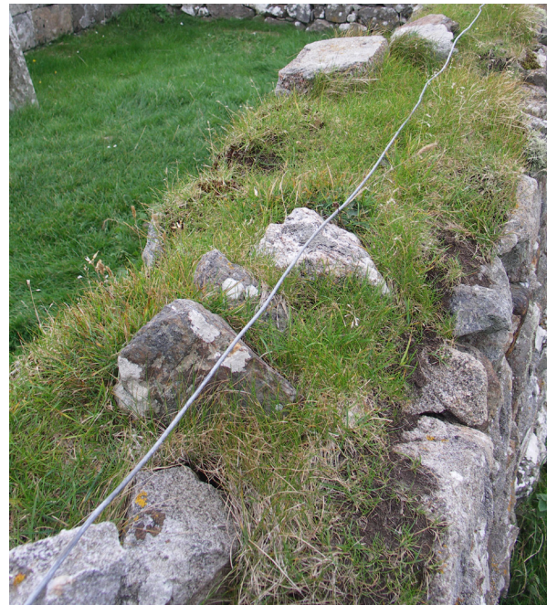
Fig. 4.5: Stones to counteract wind uplift, Roghadal Church, Harris (CS37).
