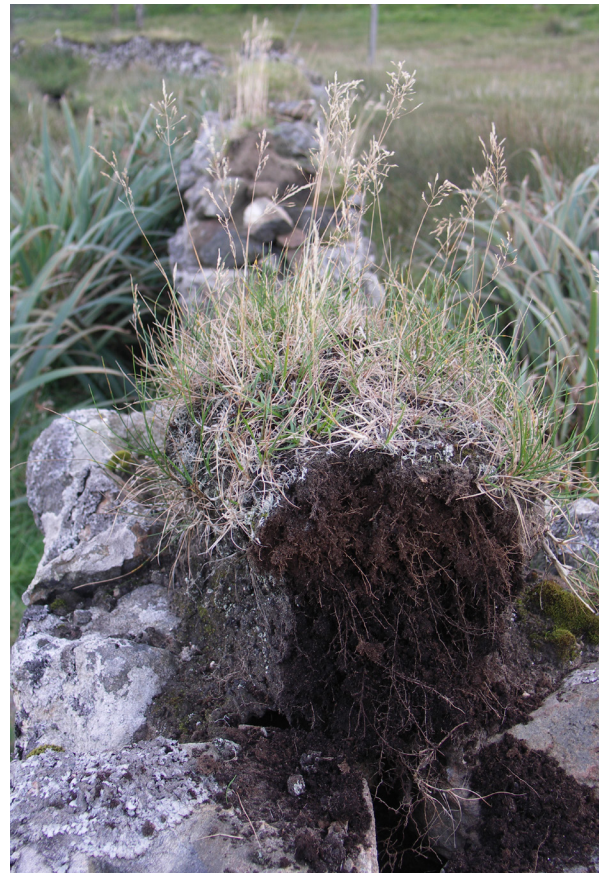
Fig. 4.11: Roghadal, Harris (CS5). The turf soil is clearly lighter than the soil dome beneath. Note the deep root penetration.
