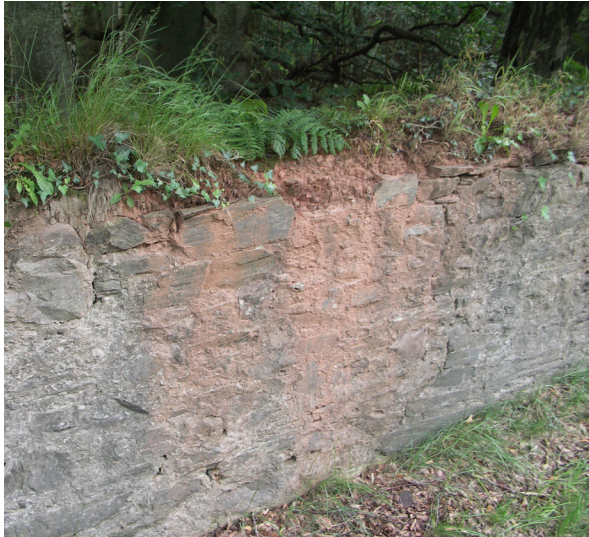
Fig. 4.15: Gordon Castle Estate (CS4). Where the clay changes to a red colour, it is much less durable.
