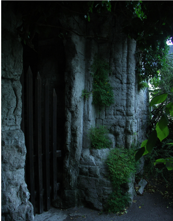
Fig. 8.3: St. Olof's Church, Visby. Entrance is carefully preserved.
