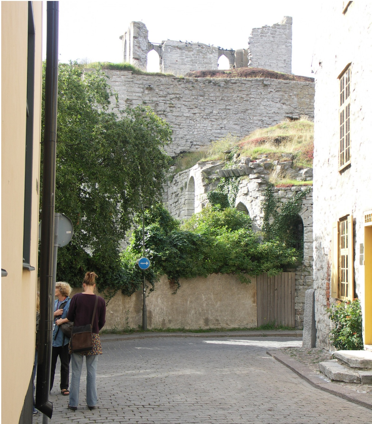
Fig. 2.41 : St. Lar's Church, Visby, Sweden. One of a series of soft capped ruins in an historic urban setting.
