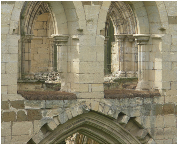
Fig. 7.25: Rievaulx Abbey, Yorkshire. Failure of turf on relatively sheltered sills, though rainwater penetration and run-off may still be reduced.
