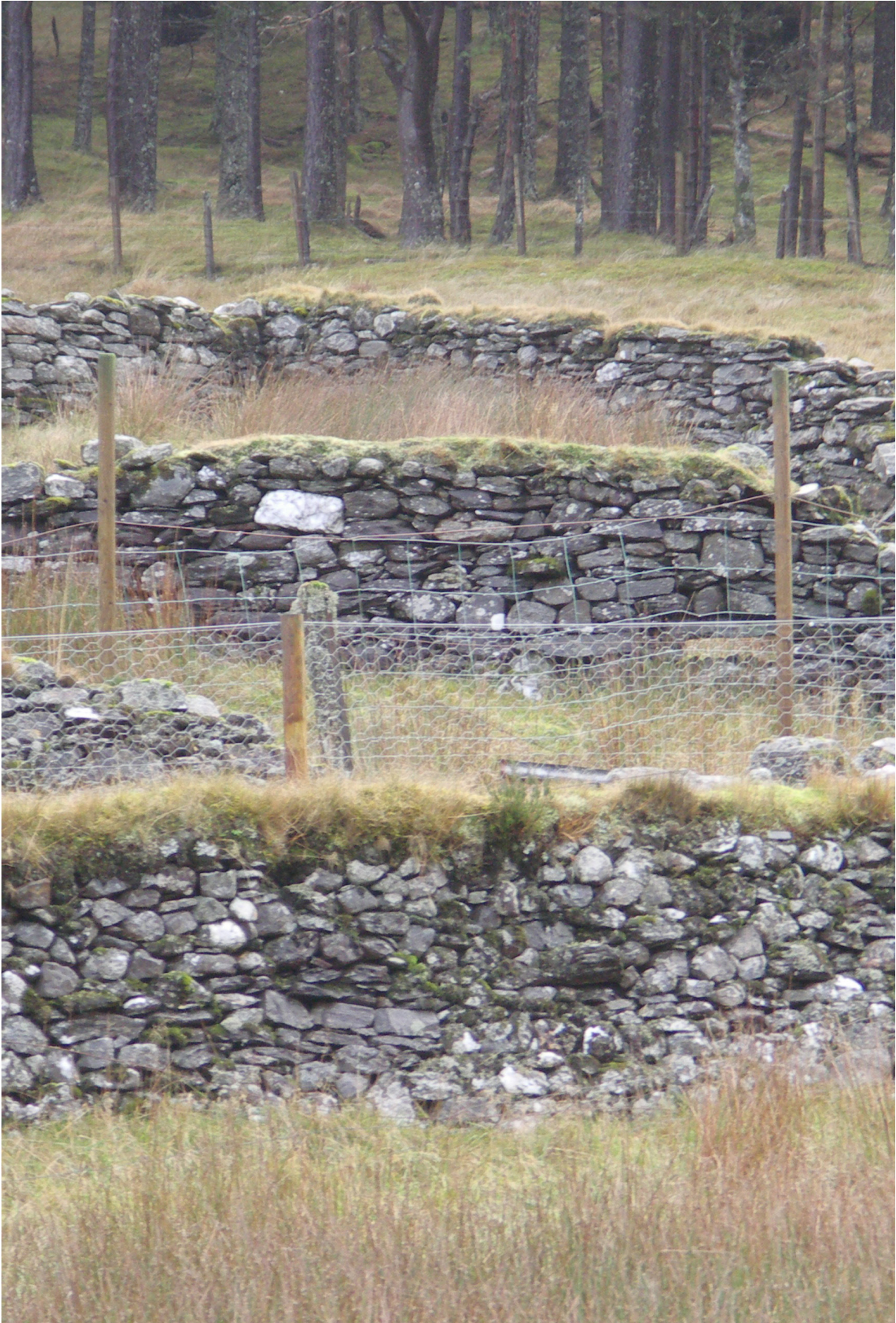
Fig. 4.1: Vernacular soft capped drystone enclosure walls, Glen Lochy.
