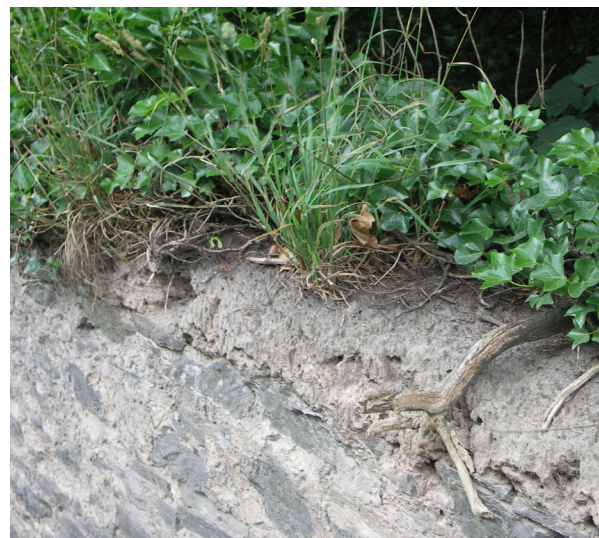
Fig. 4.14: Gordon Castle Estate (CS4). The original domed profile of the clay cap is revealed where there is no plant cover.
