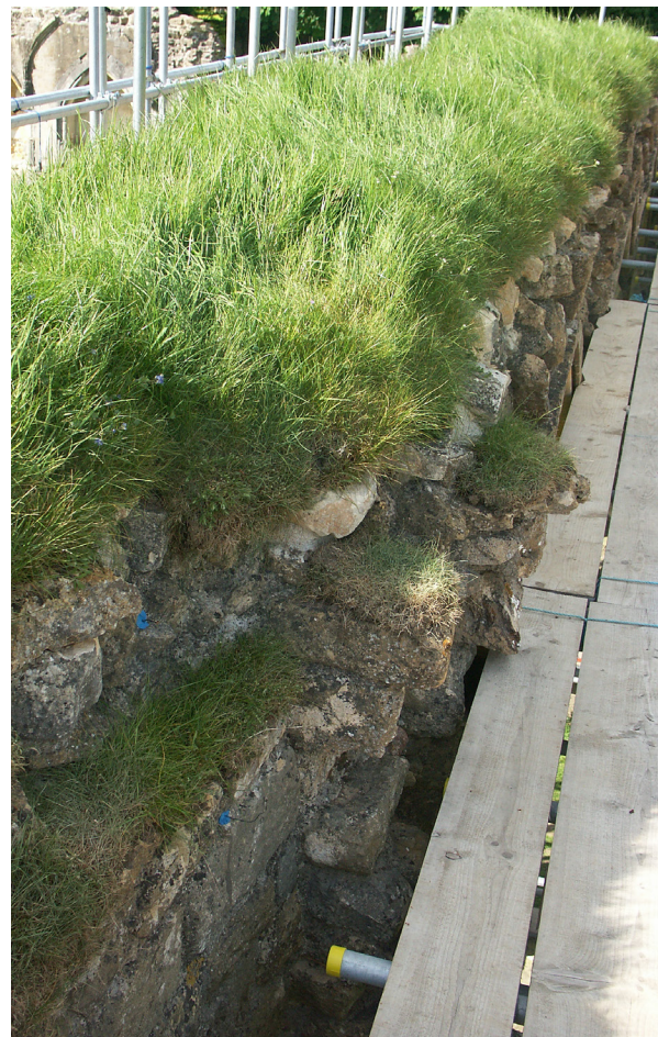
Fig. 7.22: Hailes Abbey, Gloucestershire. tests show good lush growth, but some failure of small sections.
