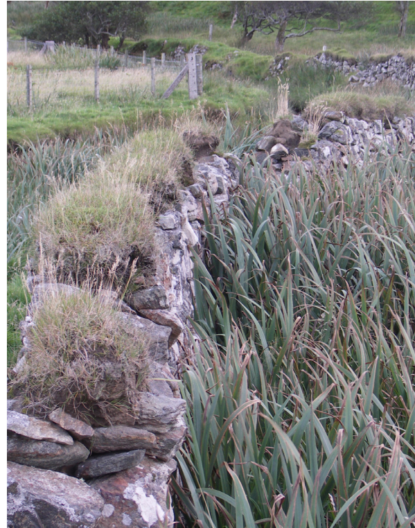
Fig. 4.10: Roghadal, Harris (CS5) Turf and soil dome capping.
