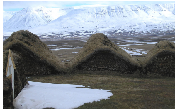
Fig. 7.33: Traditional parallel ranges with turf over timber structures and turf cross-walls.
