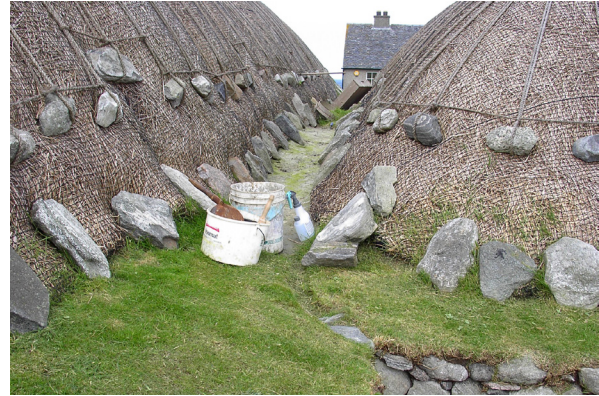
Fig. 4.21: The Blackhouse, Arnol, Lewis (CS9.) The valley gutter has clay, but not turf.
