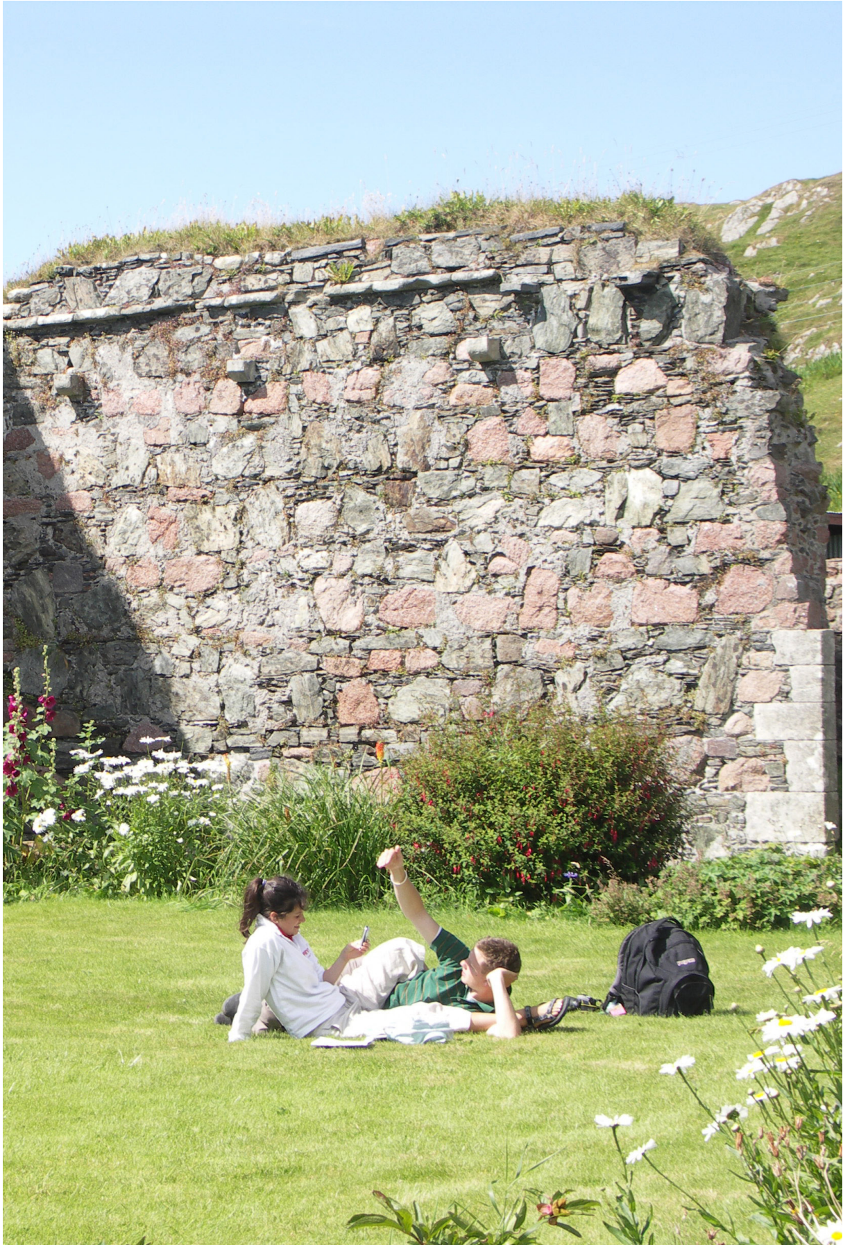
Fig. 1.3: Naturally established cappings, the Nunnery, Iona, Argyll.
