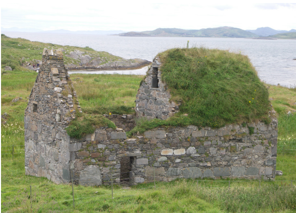
Fig. 3.21: St. Cormac's Chapel, Eilean Mor, Argyll (CS1). Although the large inclined, and narrow flat surfaces are naturally colonised, the narrow, inclined gable remains essentially bare.
