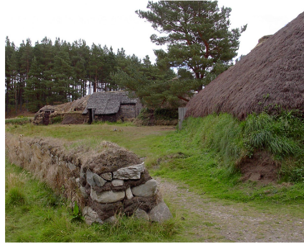
Fig. 4.17: Modern turf walled building at the Highland Folk Museum, Newtonmore. The verdant face of the turf wall, compared to the dry turf and stone enclosure wall, is a result of rain shed from the roof onto the wall face.
