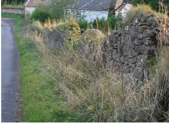
Fig. 4.8: Turf and soil dome capping, near West Linton, Peebles-shire.
