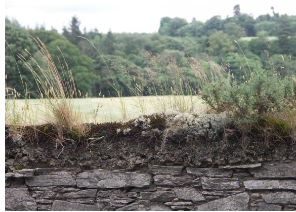
Fig. 3.40: Gordon Castle Estate Wall, Moray (CS4) . Mosses form a stable central cap, augmented by lichen, through which grasses rise thinly.
