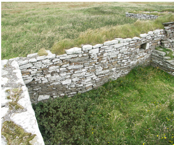
Fig. 3.28: Eynhallow Monastery, Orkney (CS18). Surface texture created by lime mortared stones fails to prevent wind decay.
