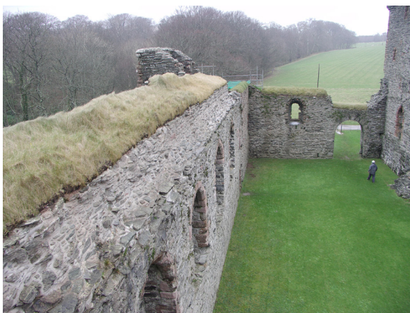
Fig. 2.39: Skipness Castle, Argyll (CS35). A turf capping cut from the grazed field in the background has limited diversity, but arguably link the building to its setting and is in tune with the lawned monument grounds.
