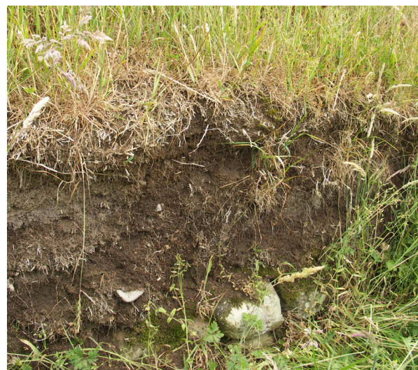
Fig. 3.31: Leannach Enclosure, Culloden, Inverness-shire (CS6). The turf walls sustain good living wallheads, but little vegetation grows on the face.
