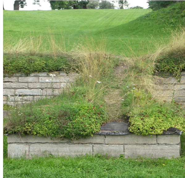
Fig. 2.18: Alvastra Monastery, Sweden. Pedestrian damage tends to be on focused routes, with the central grass more resilient than the edge sedums.
