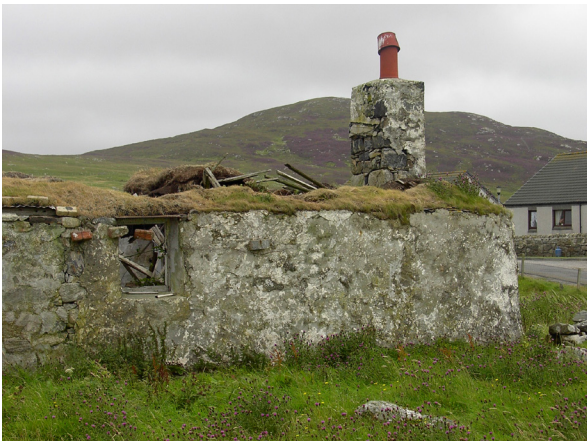
Fig. 5.5: Decaying Blackhouse, Howmore, South Uist. The process of deposition is complete. Note the lack of plants on the chimney head and window sill.
