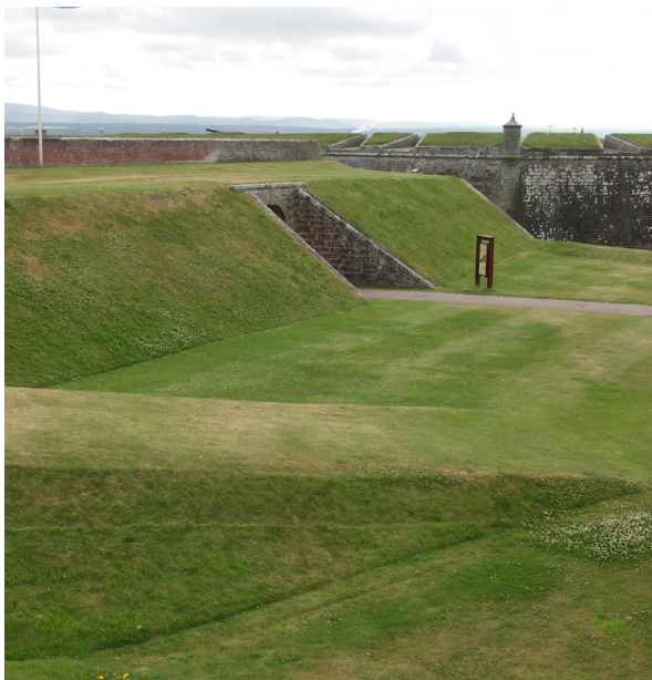
Fig. 1.4: Fort George, Inverness-shire, earthworks and embasures.
