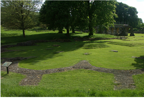
Fig. 2.30: Hailes Abbey, Yorkshire. The altar (centre right) has recently been re-buried, though its form still reads within the low-lying consolidated limestone wallheads, which remain more vulnerable to decay.
