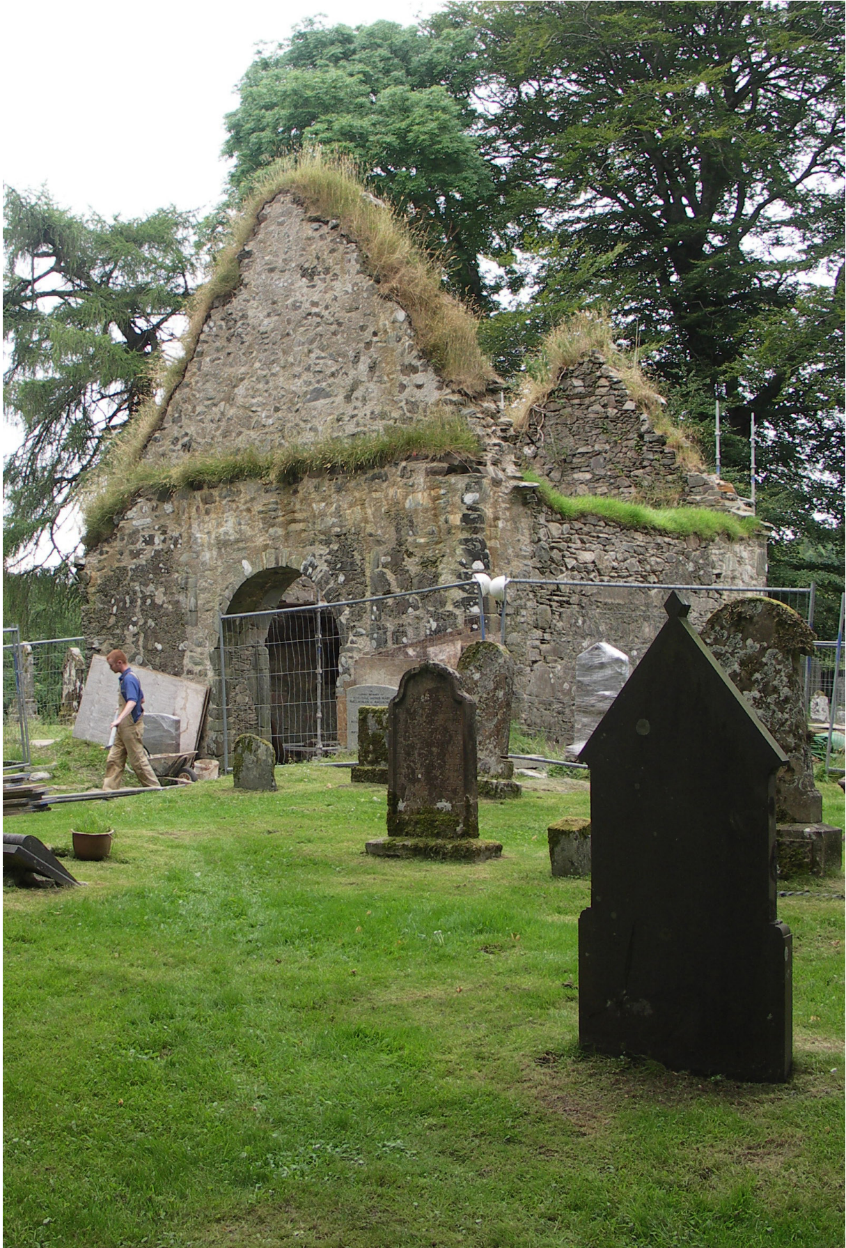
Fig. 1.2: Soft capping work in progress, Kilmory Chapel, Argyll.
