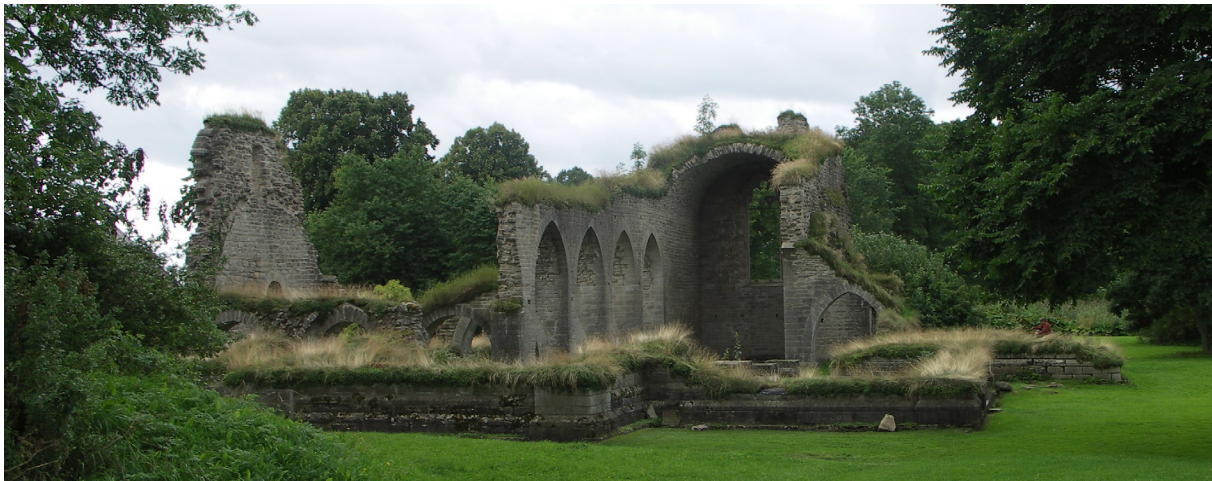
Fig. 7.2: The Alvastra Monastery, Sweden, a good example of the picturesque achievements of contemporary soft capping.
