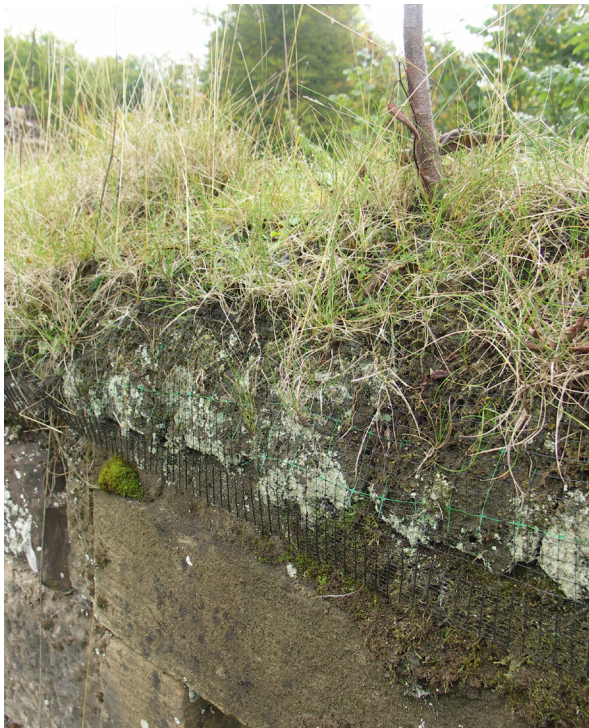
Fig. 3.2: Doune Castle Mill, Stirlingshire. High levels of moisture seem to have inhibited growth, especially at the edge.
