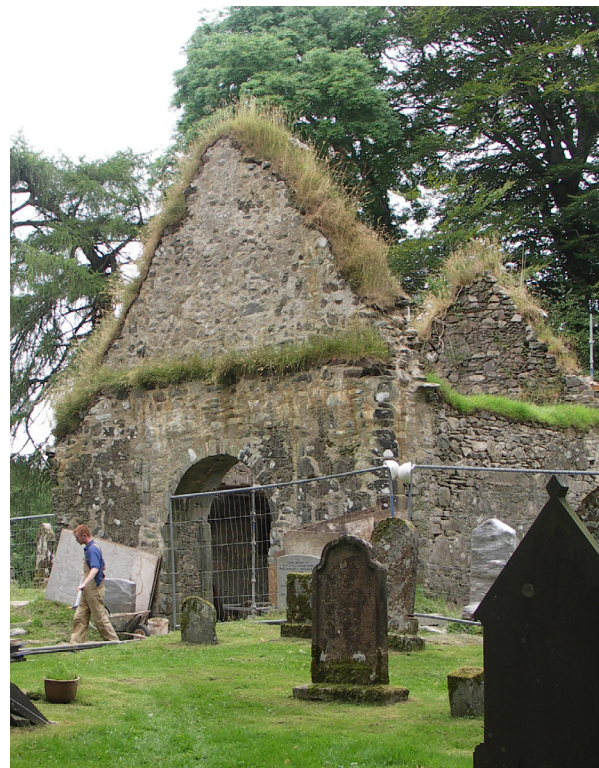
Fig. 3.23: Kilmory Chapel, Argyll (CS23). The mild, sheltered conditions on this site allow the steep gable in front to be successfully capped. The rear gable still retains its natural vegetation.
