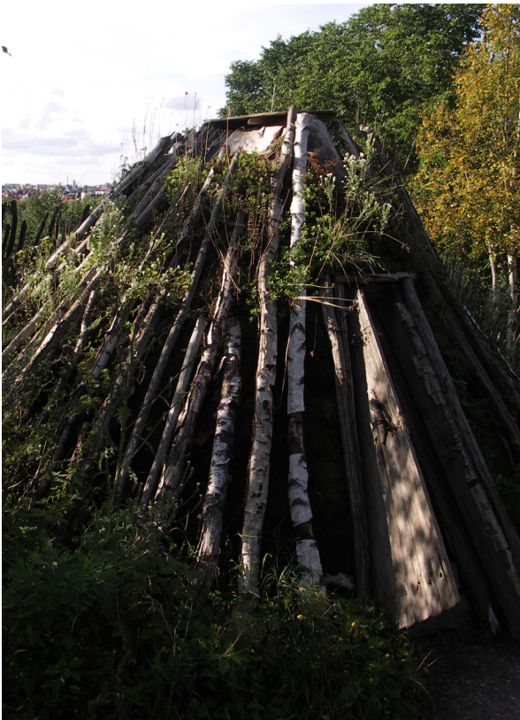
Fig. 4.24: Seasonal hut of the Sami people, Sweden. The birch bark layer under the turf was a valuable resource and often re-used. Birch poles over the turf prevent wind damage to the turf.
