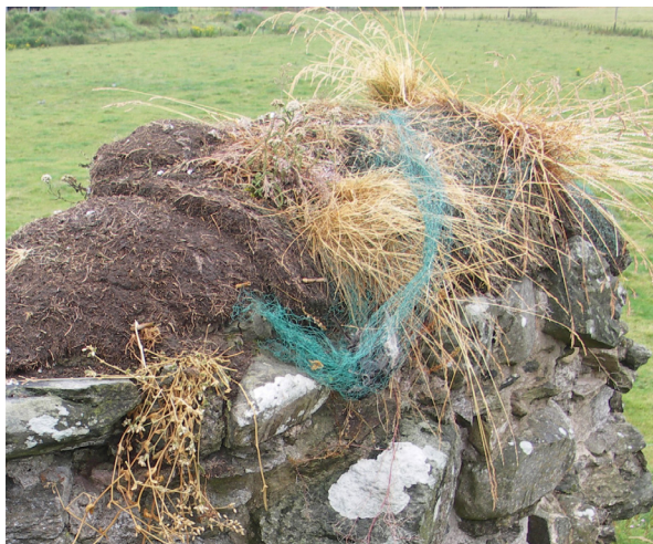
Fig. 3.62: Black Castle, Perthshire (CS13). Plastic mesh proved problematic in the long-term.
