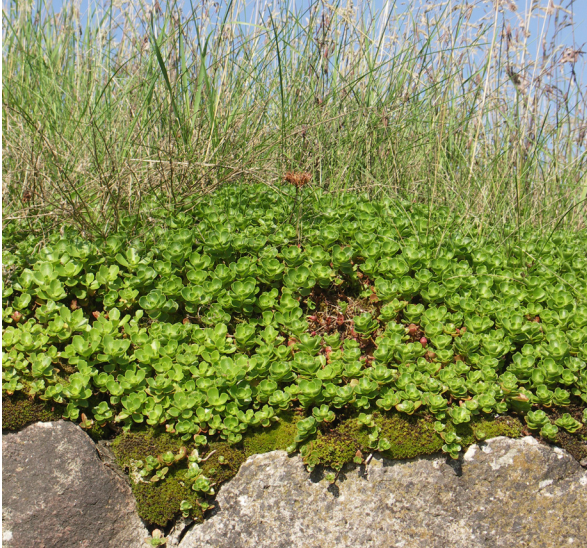
Fig. 3.49: Bohus Fortress, Sweden. A designed soft cappings, with a central strip of grass, sedum edge, and later colonisation by moss.
