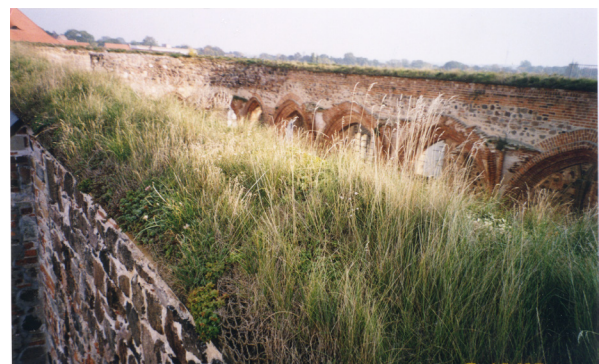
Fig. 7.32: St. Nicolai's Church. After three years the wallhead was stable and attractive.
