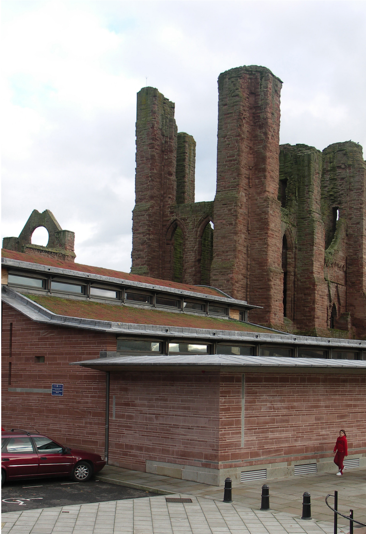
Fig. 2.1: Arbroath Abbey, Angus. The modern visitor centre in the foreground has a sedum roof. This complements the historic masonry ruin, which has been colonised by algae.
