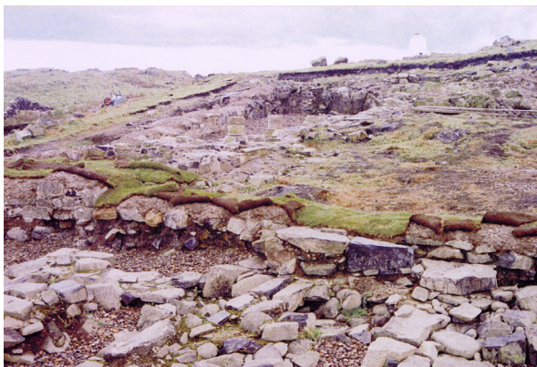
Fig. 3.15: Isle of May, Fife (CS36). Uplift from helicopters delivering materials lifted turfs off the caps during the works.
