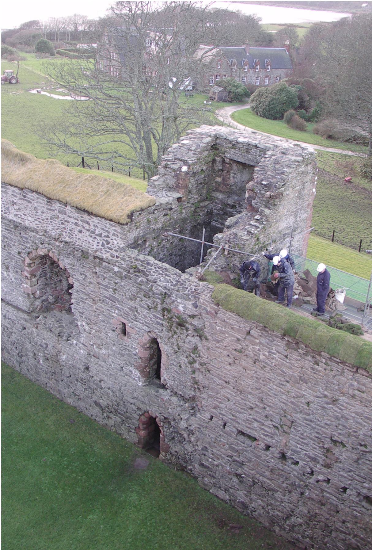
Fig. 1.1: Soft capping work in progress, Skipness Castle, Argyll. November 2004.
