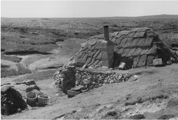
Fig. 4.19: Sheiling, Ness, c. 1958, The good condition of the thin turf covering to the stone wall suggests it may benefit from moisture retained in the earth wall core, as well as water received from the area of turf roof.
