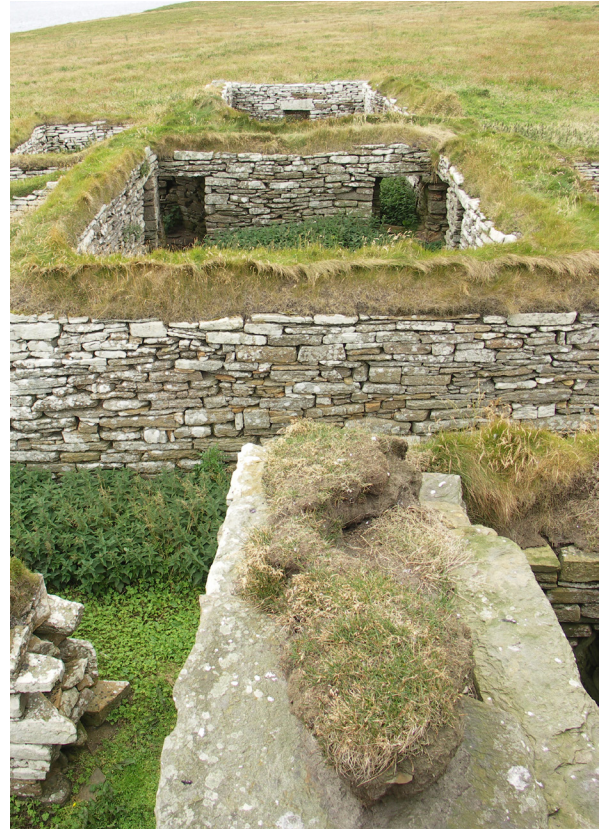
Fig. 3.12: Eynhallow Monastery, Orkney (CS18). The effect of elevation on cappings about seventy-five years old. In this location, wind gives any capping at high level a limited lifetime, irrespective of other factors.
