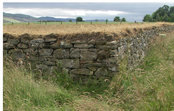
Fig. 4.7: Reconstruction at the Culloden Battlefield. The poor condition of the turf capping contrasts with that of the adjacent reconstructed turf wall, Fig 3.31, suggesting that the greater moisture retained by the turf was significant.
