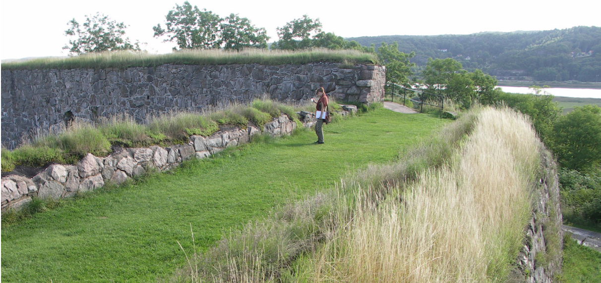
Fig. 7.7: Bohus Fortress, west Sweden, wallhead soft cappings over bitumen membranes.
