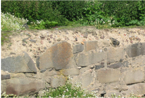
Fig. 3.14: Isle of May, Fife (CS36). Large stones in the capping soil, exposed by accelerated wind erosion of the soil.
