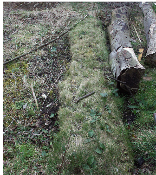
Fig. 3.26: Monimail Tower, Fife (CS27). An excavated wallhead protected by soft cappings.
