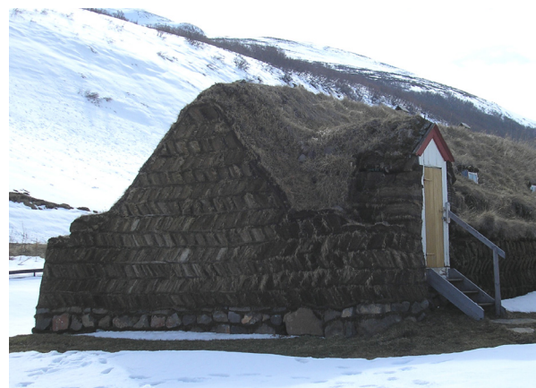
Fig. 4.18: Turf wall construction continues in Iceland, as part of the same bio-regional tradition that existed in Scotland.
