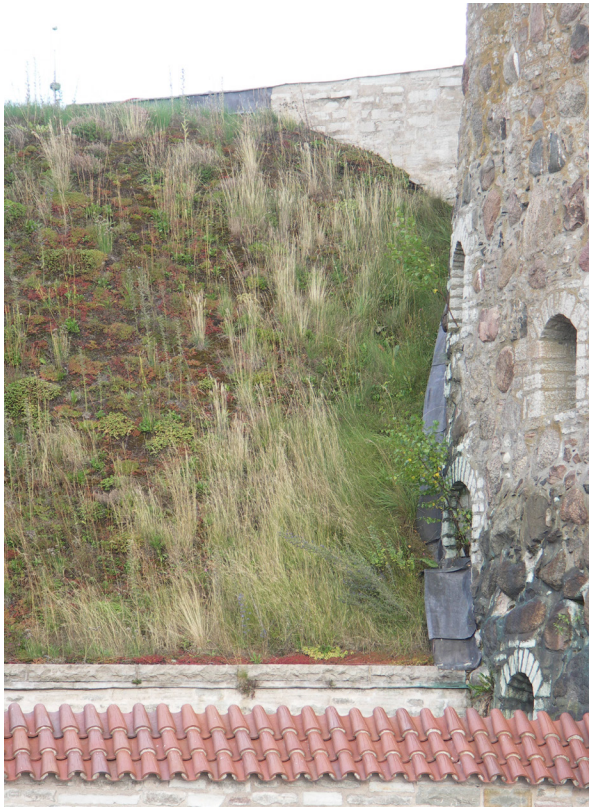
Fig. 3.53: Vadstena Castle, Sweden. Increased soil fertility has not improved performance on a site prone to drought conditions. In contrast, shade provided by corner towers encourages the desired grass growth over sedum.
