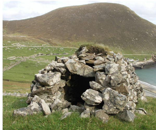
Fig. 4.30: Cleitean, St. Kilda (CS7). Progressive collapse of the masonry inevitably follows decay of the soft capping.
