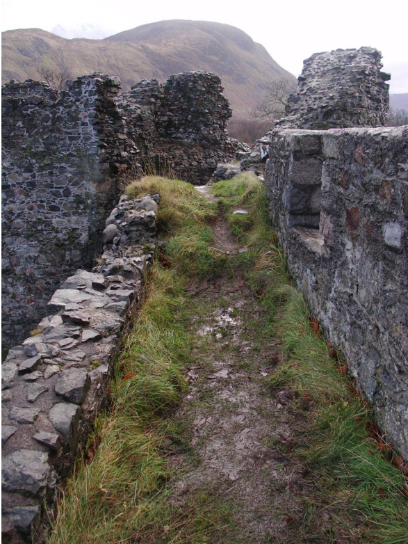
Fig. 3.63: Inverlochy Castle, Invernesshire(CS21). Although these high level soft cappings have been damaged by visitors, they have effectively protected the masonry beneath.
