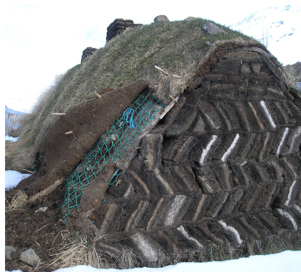
Fig. 7.34: New capping and turf wall.
