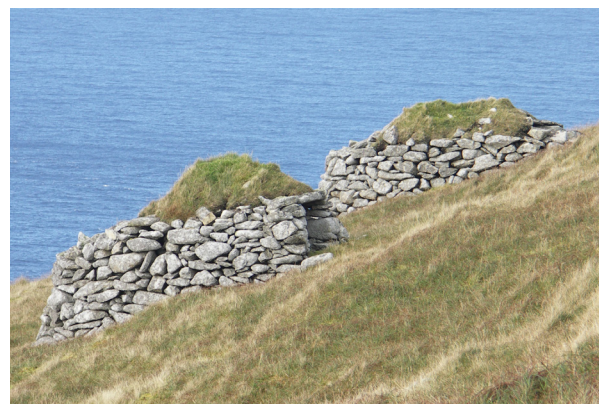
Fig. 3.13: St. Kilda, Western Isles (CS7). Cappings that are thought to be at least a hundred years old, at 600m altitude, west facing, yet proving stubbornly resilient to North Atlantic winds.
