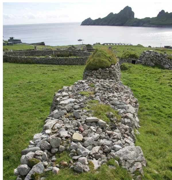
Fig. 4.29: Cleitean, St. Kilda (CS7). The soft cappings sit on a layer of small stones, over large stone slabs.
