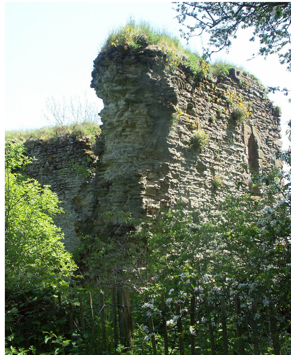
Fig. 7.18: Wigmore Castle, Herefordshire. While ivy was removed, other wall face plants were not.
