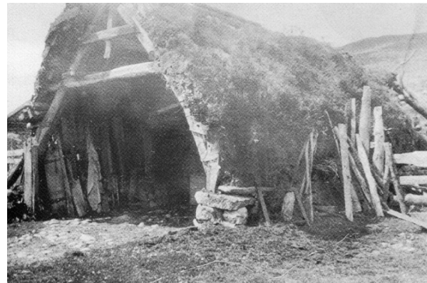
Fig. 4.22: Cruck framed building, Inverness-shire, 1920s. Apparently a living heather turf over timber framing at steep pitch.
