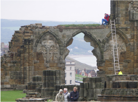
Fig. 7.19: Whitby Abbey, Yorkshire, experimental capping to test the effect of high winds.
