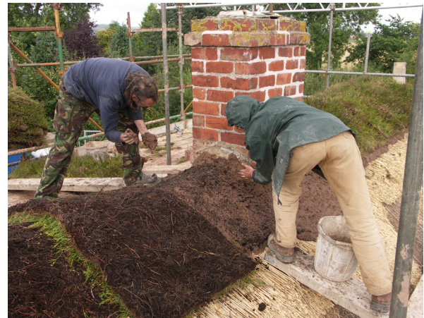
Fig. 4.25: Cottown, Perthshire. A layer of clay being laid over the thatch ridge, to be covered with two layers of turf, root to root.
