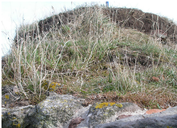
Fig. 3.43: Sedum alba stabilising a sloping edge at Cressford Castle, Roxburghshire (CS2).
