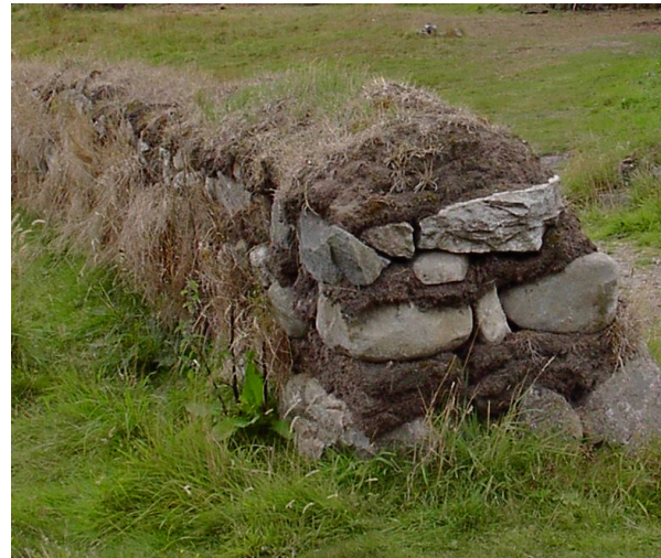
Fig. 4.4: Highland Folk Museum, Newtonmore. Composite turf and stone wall.
