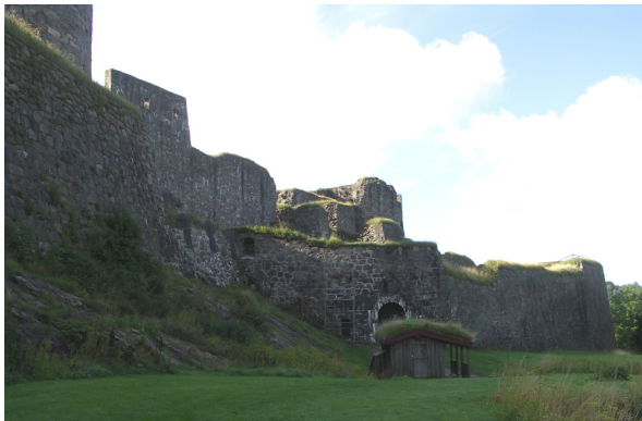
Fig. 7.5: Bohus Fortress, west Sweden, soft cappings on ruined masonry.
