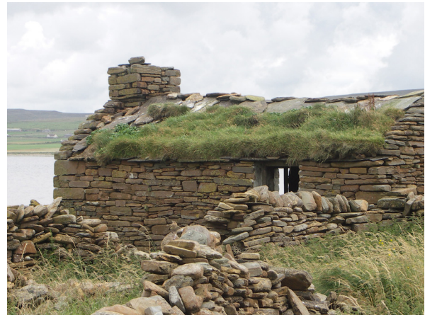
Fig. 2.37: Ruined Cottage, Eynhallow, Orkney. Less than 1km from the monastery, the vegetation on this roof is a decaying part of the original roof construction of a cottage abandoned around 1851.
