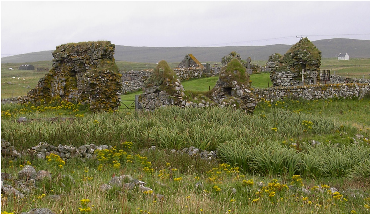
Fig. 5.2: Howmore Churchyard, South Uist. Amid a bio-diverse setting, only a limited number of relatively benign species have colonised the masonry.
