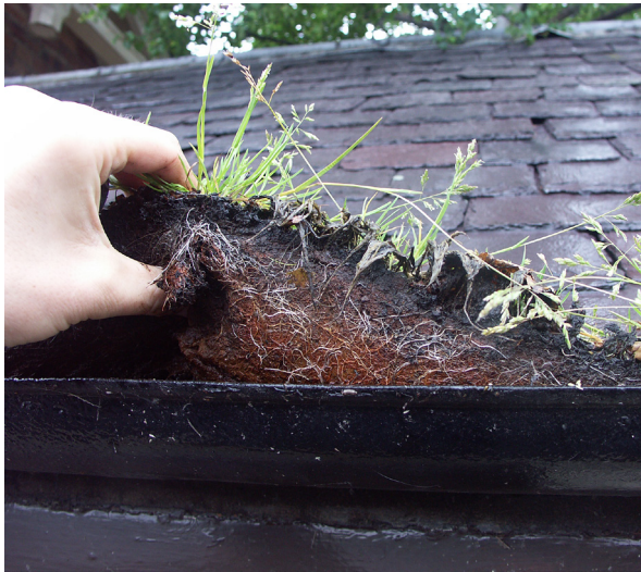
Fig. 5.3: Grass established in a gutter, collecting deposited material and decayed plant matter.
