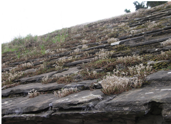
Fig. 3.42: Sedum alba naturally established on a sandstone slate roof in Angus.
