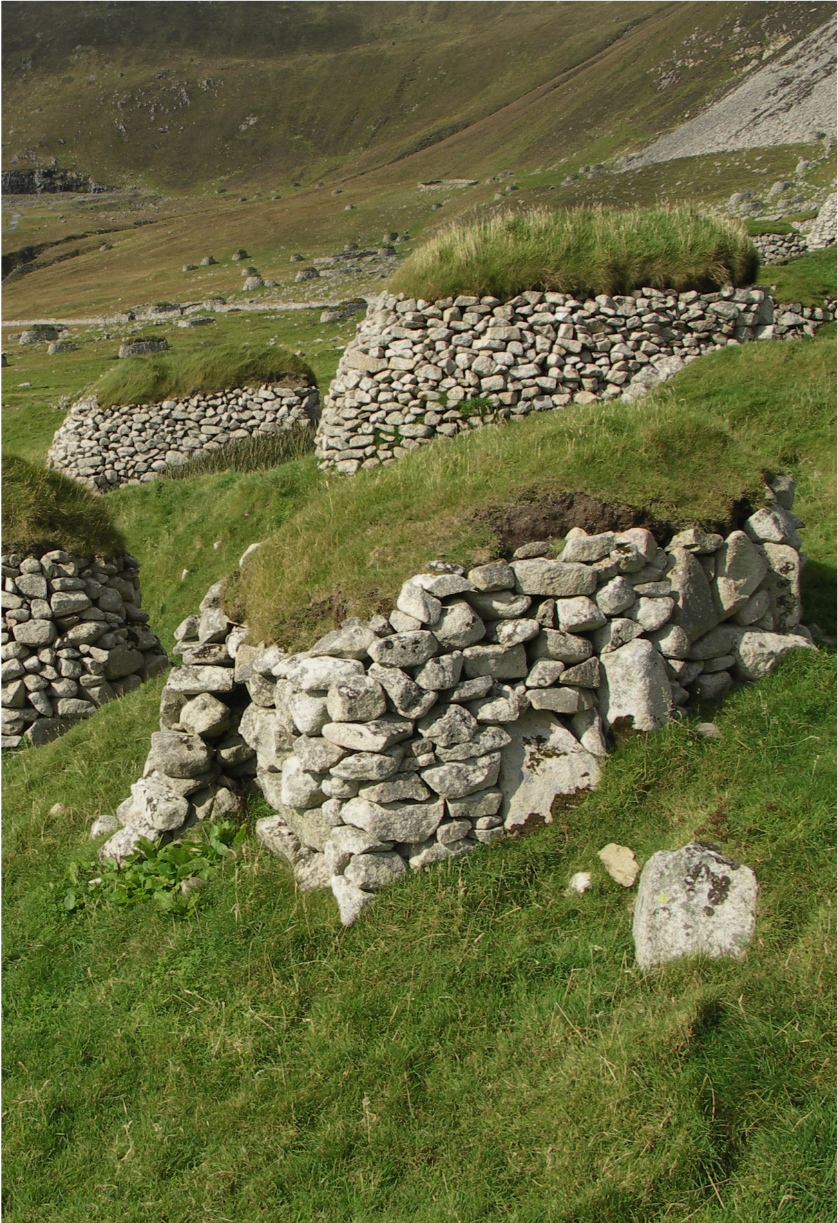
Fig. 3.1: Cleitean, St. Kilda, Western Isles. Performance of individual cappings varies dramatically for reasons that are not fully understood.
