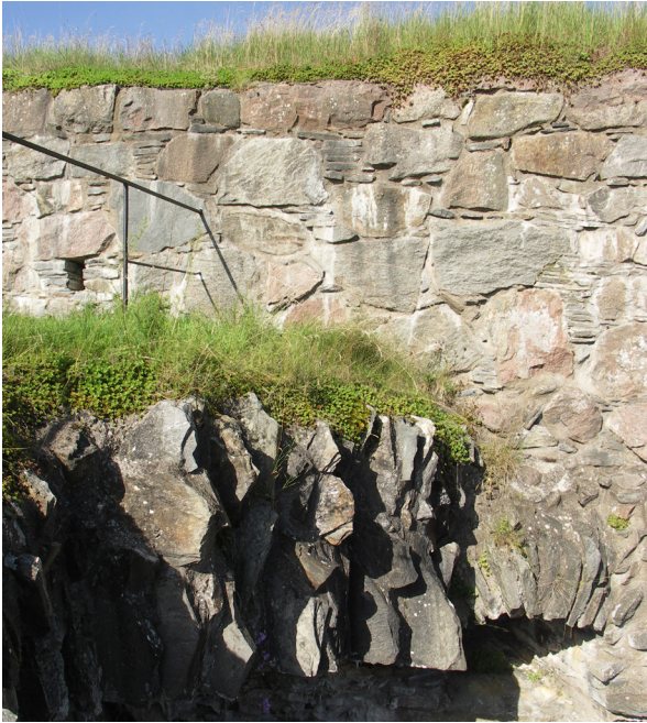
Fig. 7.9: Bohus Fortress. The edge is well defined, while concealing the hard cap.
