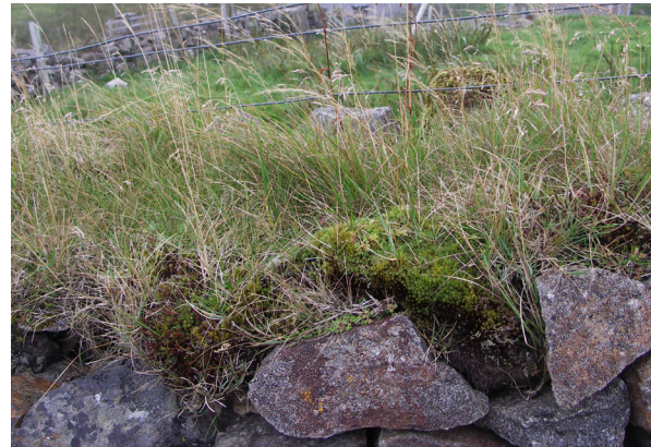
Fig. 3.30: St. Clement's Churchyard, Roghada, Western Isles (CS37). The vernacular soft cappings bind the drystone masonry at the vulnerable wallhead.
