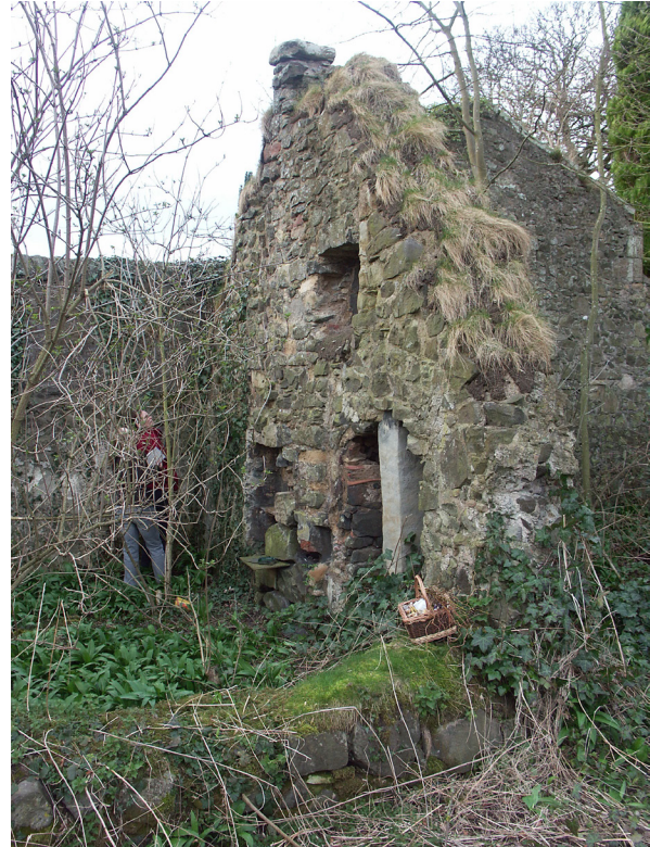
Fig. 3.22: Monimail Tower, Fife (CS27). Cappings on the gable have tended to stabilise onto shallower inclines, as a series of stepped cappings.
