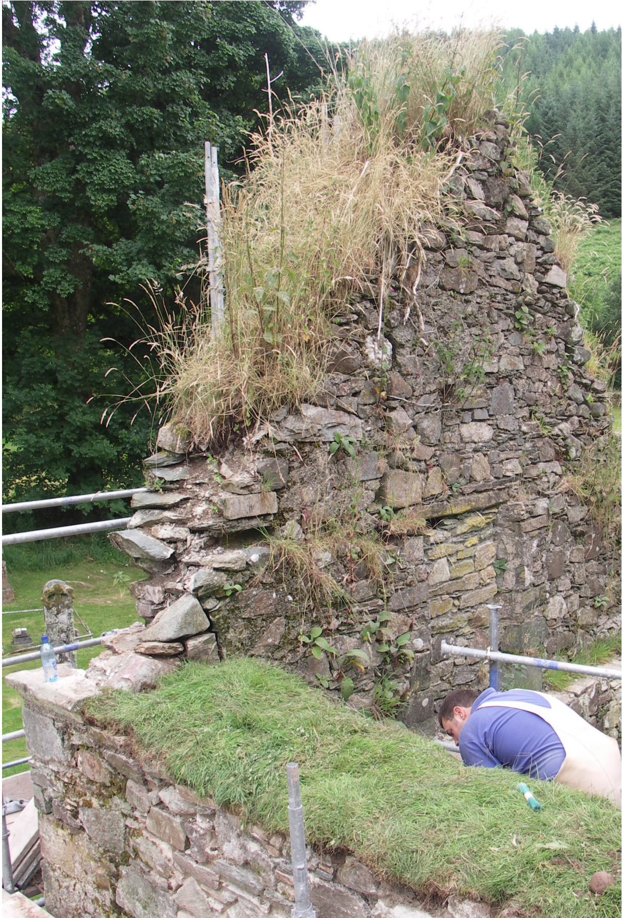
Fig. 6.1: Kilmory Chapel, Argyll (CS23), soft capping in progress.
