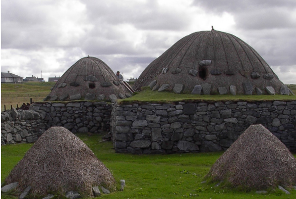
Fig. 4.20: The Blackhouse, Arnol, Lewis (CS9). The low pitch of the wall cappings implies that much of the rainwater from the roof was not shed off. The profile of the building is testament to the power of the wind.
