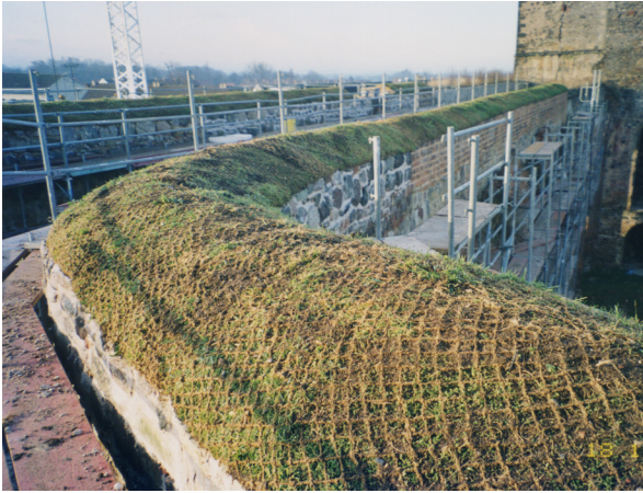
Fig. 7.29: St. Nicolai's Church. Hessian protecting the finished capping.
