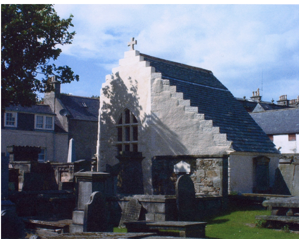
Fig. 6.5: St. Mary's Church, Banff, after full restoration.
