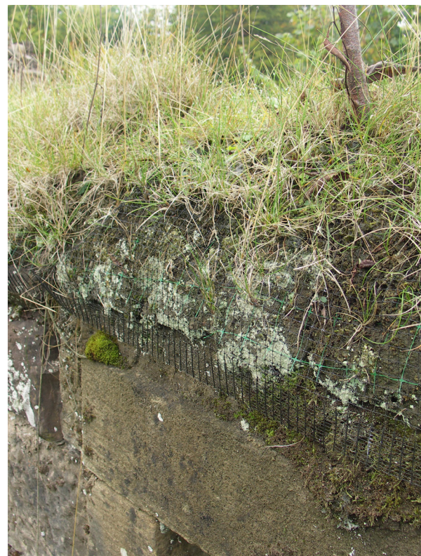
Fig. 3.48: Doune Castle Mill, Stirlingshire. Originally soft capped with commercial turf, dieback has allowed moss and lichen to colonise the sides, while trees invade the grass on top
