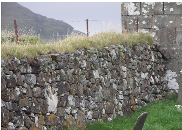
Fig. 2.23: St. Clement's Church, Roghadal, Lewis (CS37). This unmaintained capping has achieved a stable balance of species.
