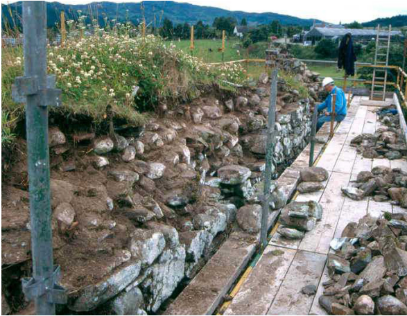
Fig. 5.6: Black Castle, Perthshire (CS13) Central section of natural capping retained as a seed reservoir.
