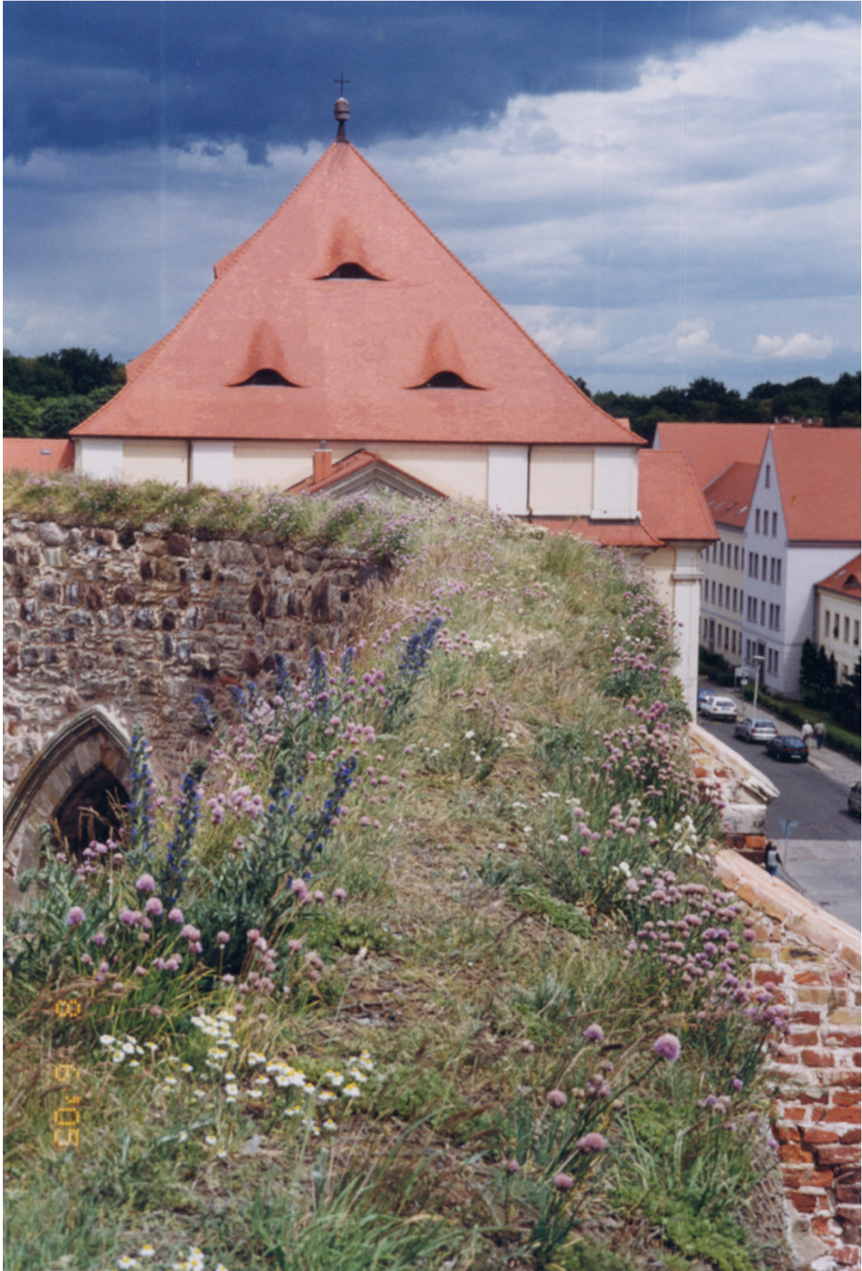
Fig. 7.1: Mature conservation cappings. St. Nikolai's Church, Zerbst, Germany.
