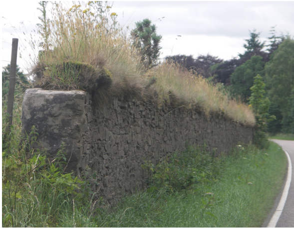
Fig. 4.12: Gordon Castle Estate, Moray (CS4). An extensive, mature and bio-diverse vernacular capping.
