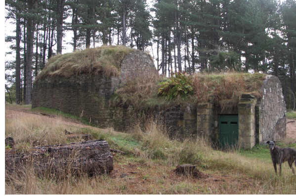
Fig. 4.32: Icehouse, Tentsmuir, Fife (CS11), early 19th century. The ice storage room has a steeper vault than the preparation chamber, presumably to keep the interior drier.
