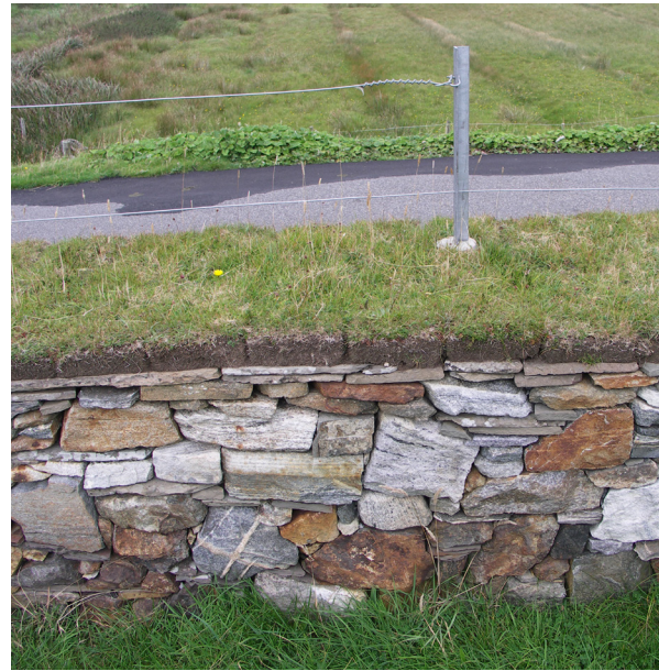
Fig. 3.55: St. Clement's Churchyard, Roghadal, Western Isles (CS37). This recent capping is flat, with no soil layer beneath the turf.
