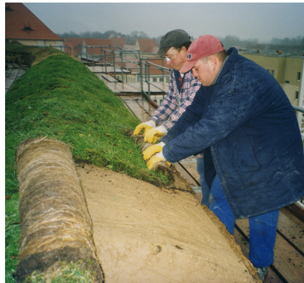
Fig. 7.28: St. Nicolai's Church. Turf rolled over carefully prepared clay caps.
