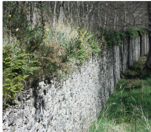
Fig. 3.33: Gordon Castle Estate, Moray (CS4). A bio-diverse setting, for mature, un-maintained soft cap.
