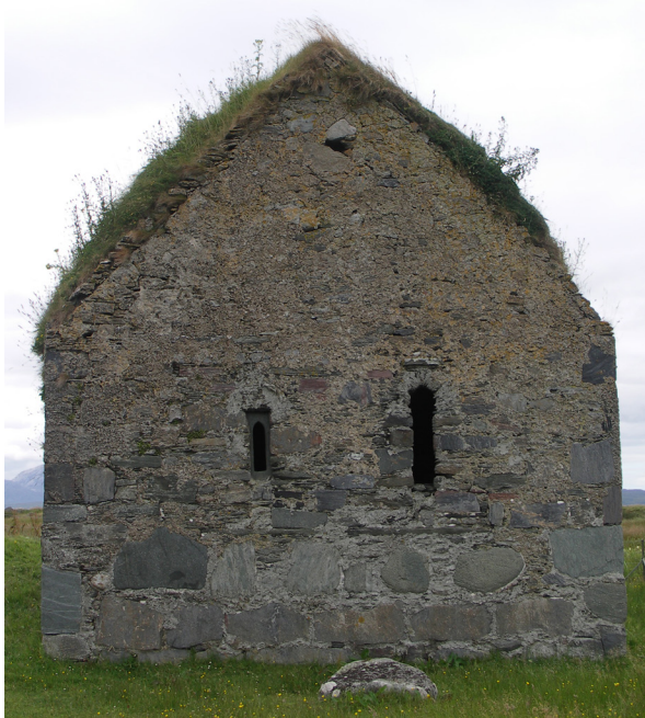
Fig. 3.24: St. Cormac's Chapel, Eilean Mor, Argyll (CS1). The capping thins towards the ridge and eaves.
