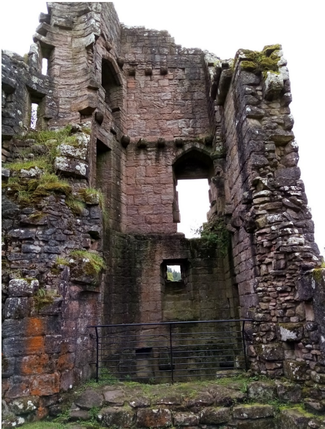
Figure 6: Interior of east tower of gatehouse
