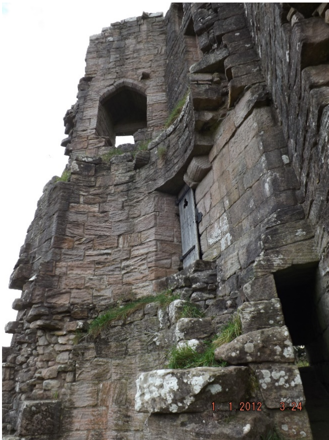
Figure 8: Interior of south-east corner tower
