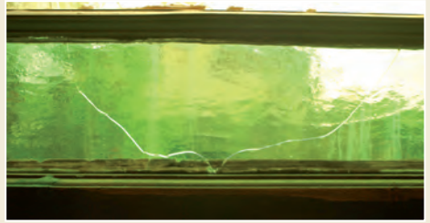
Fig. 9: A stress fracture in a pane of glass.
