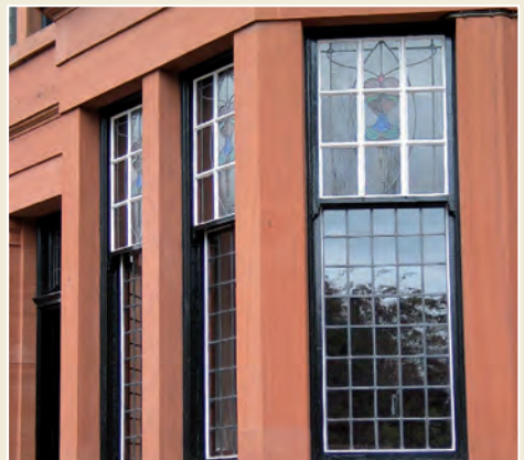
Fig. 8: Decorative glass fixed in a timber framed window.
