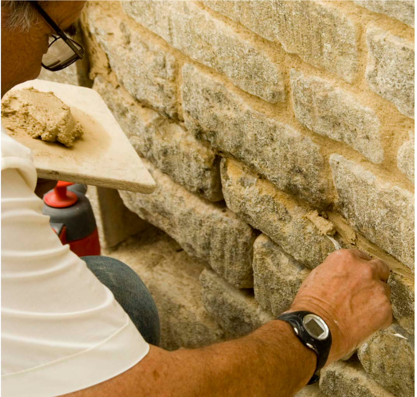
Above: Lime mortar is applied between stones.
