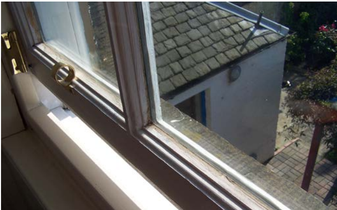
Left: The original timber window frame can accommodate new double-glazing, making the change visually discreet. Next page: Double glazed units in sash windows.
