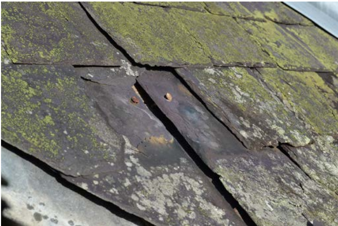
Above: Missing and slipped slates can cause water ingress.
