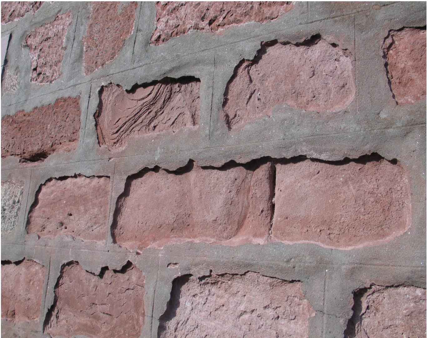
Above: Cement mortar applied to this stone wall has led to increased stone decay.
