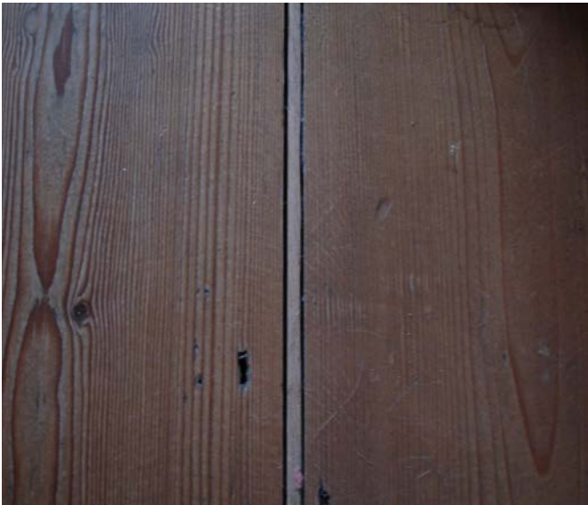
Left: Plugging gaps between floorboards.
