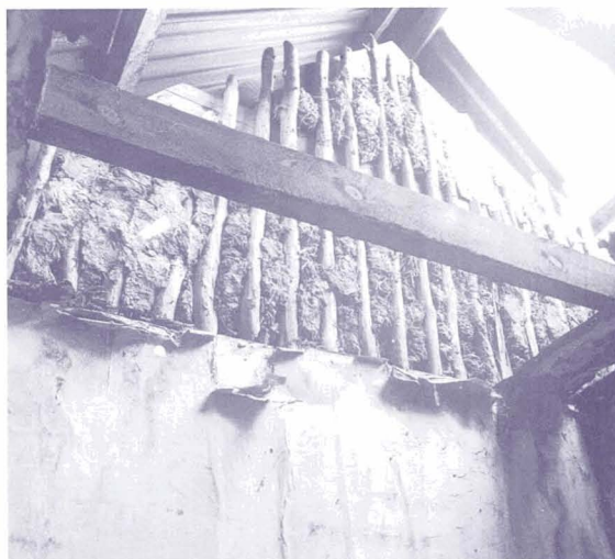
Hill of Fearn., Ross-shire. Kebber and mott internal gablet - untreated side
