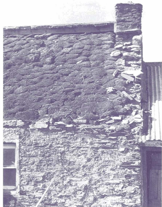
Auchterless, Aberdeenshire. Turf used as insulation under corrugated iron
