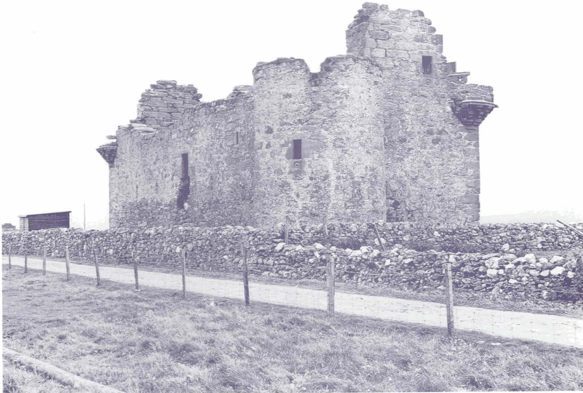
Clay mortared walls, Muness Castle, Unst, Shetland
