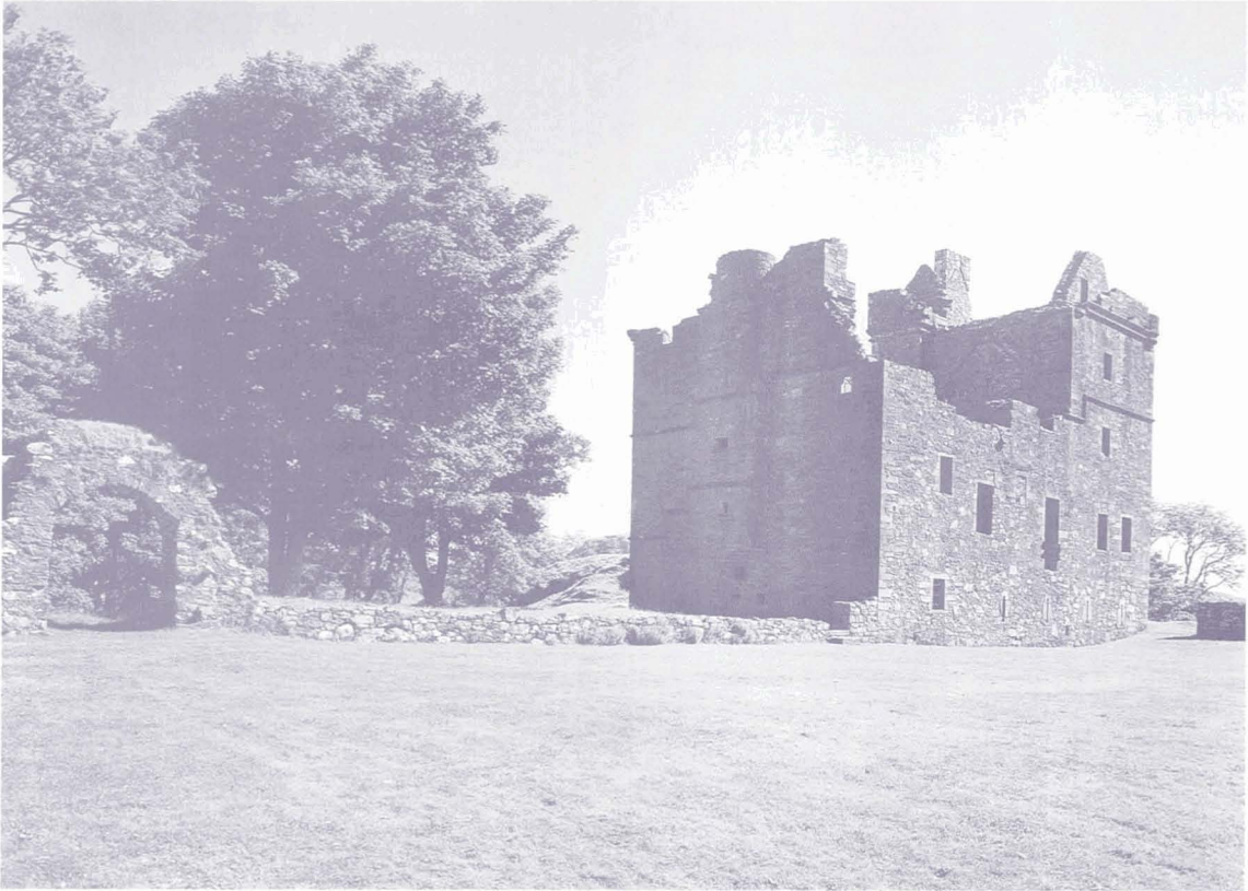
Clay mortared walls, Carnassorie Castle, Kilmartin, Argyll
