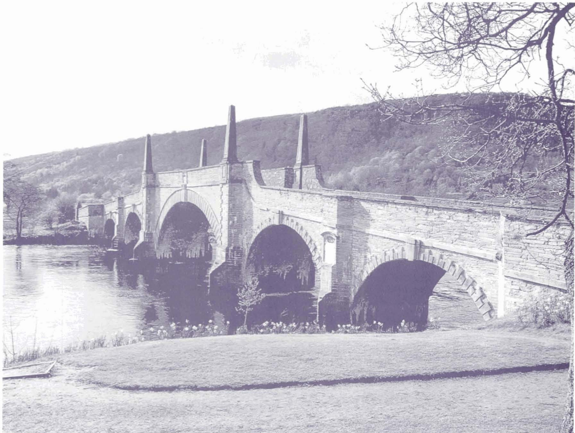
Wade bridge, Aberfeldy, Perthshire. Bridges of this type have puddled clay under the roadway, at the back of the masonry arches and spandrels. Damage to this clay is evident from the limescale visible under the arches.
