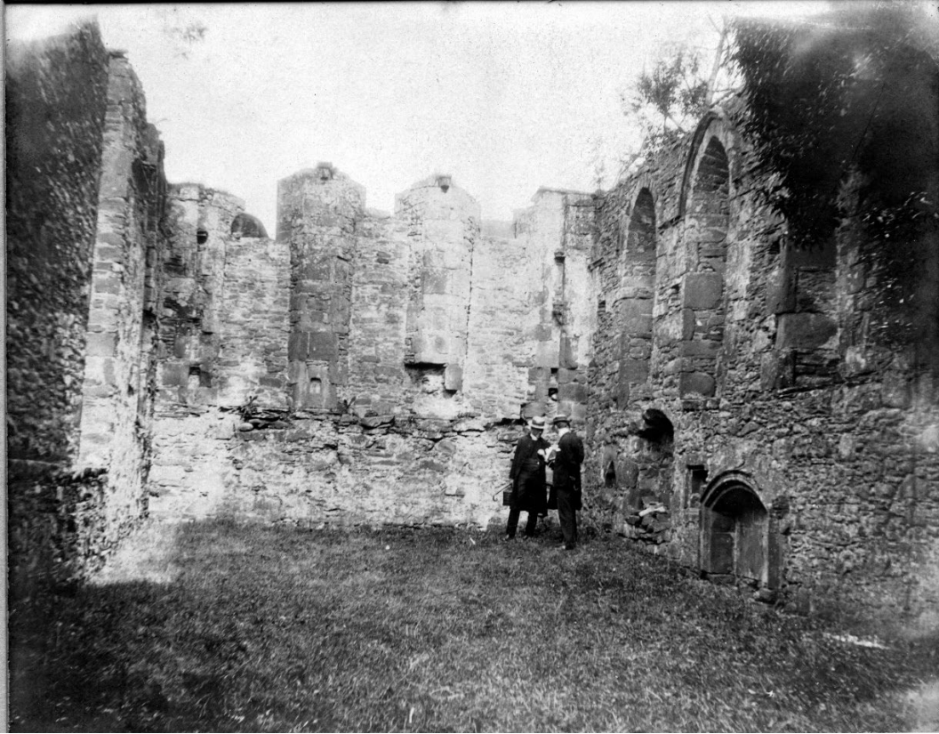
Figure 6: A view of the west end of the nave showing the 3 windows blocked up. © Angus Council Collections cared for by ANGUSAlive Museums, Galleries and Archives.
