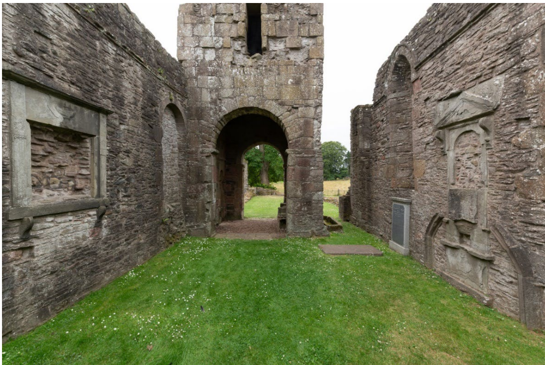
Figure 5: The same view as Figure 4, but after clearance works. Note the removal of walling between the tower and the chancel north wall. © Historic Environment Scotland
