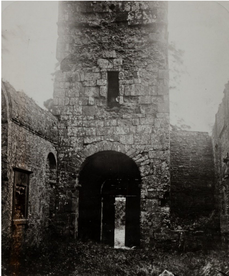
Figure 4 Interior of Restenneth Priory chancel in 1874, prior to consolidation and clearance works. © Courtesy of HES
