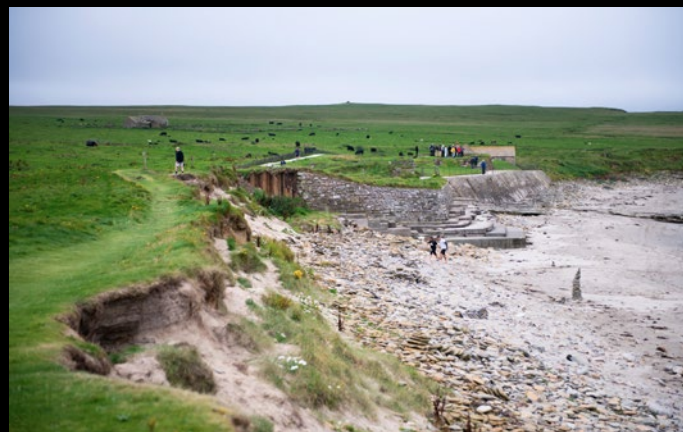
Coastal erosion and seawall at Skara Brae.
