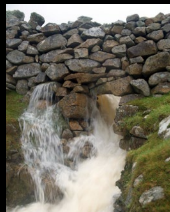
After heavy rainfall the drystone walls allow water to flow but are under stress. © National Trust for Scotland
