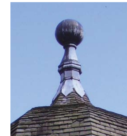
A lead concealed finial
