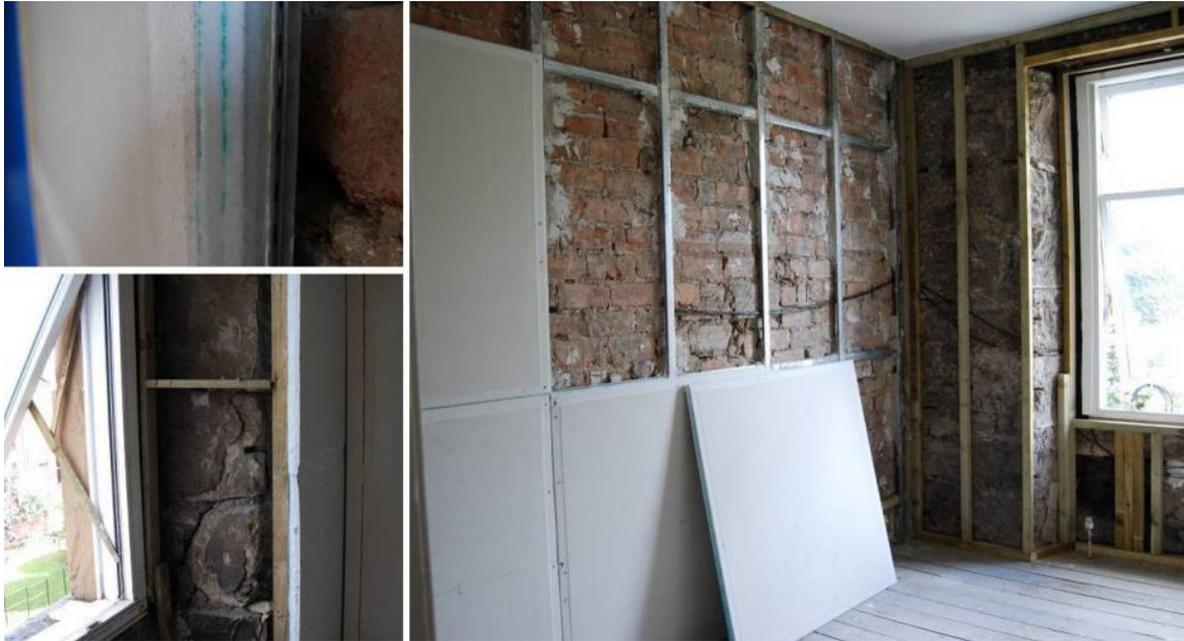
Figure 54 Aerogel blanket insulation bonded to plasterboards is fixed to metal studwork, leaving air cavities in between the studs and between insulation and masonry.
