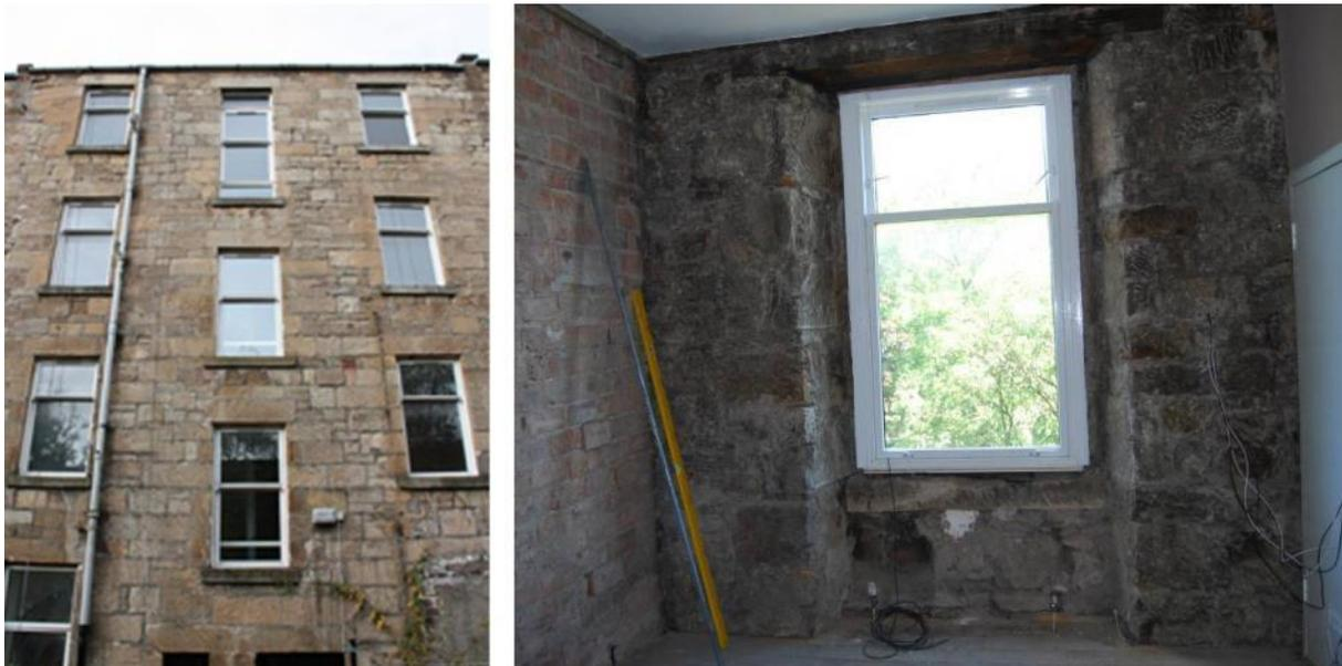
Figure 52 The case study is based on the rear wall of a Glasgow tenement, constructed as randomly coursed masonry with squared sandstones, bedded in lime mortar.
