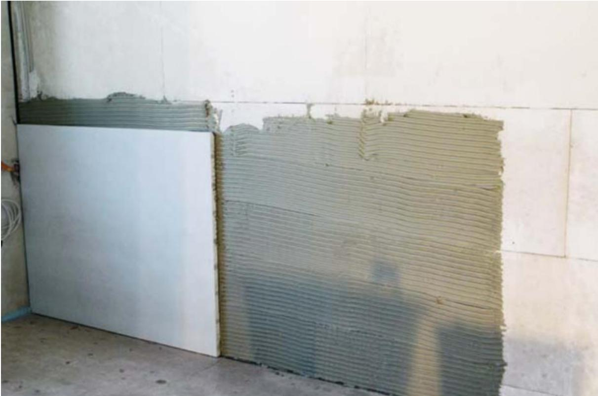
Figure 56 Calcium silicate boards are fixed to the masonry with a mortar-based adhesive. For the case study, a plaster finish and a levelling plaster coat was assumed to provide a level surface.
