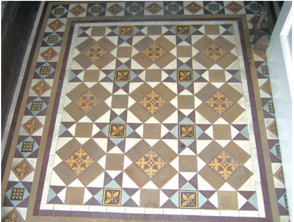
Fig.3 An early 20th century ball floor in Perthshire, with encaustic and geometric tiles.
