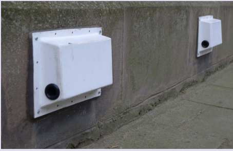
Fig. 5 Temporary air brick covers (© Paul Hendy).
