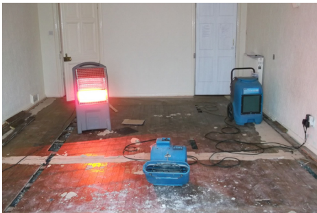
Fig. 8 Conventional heating and dehumidification.
