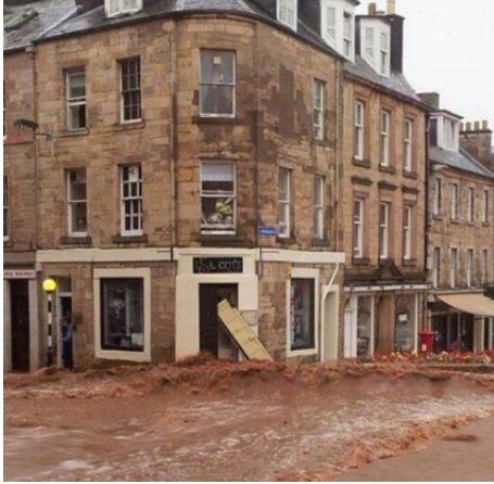
Fig. 2 Flooding caused by blockage in surface water drainage system (© M. Kay).
