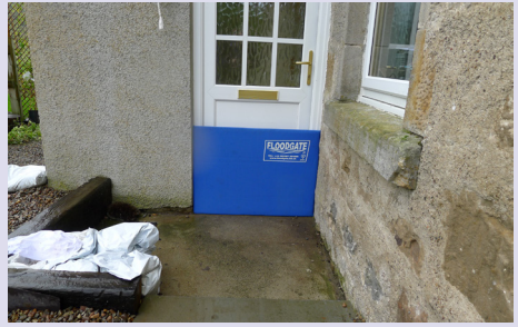
Fig. 6 Temporary flood barriers can be easily fitted into permanently fixed frames when required (© Paul Hendy).
