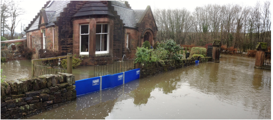
Fig. 7 Perimeter flood barriers can keep water away from a property.
