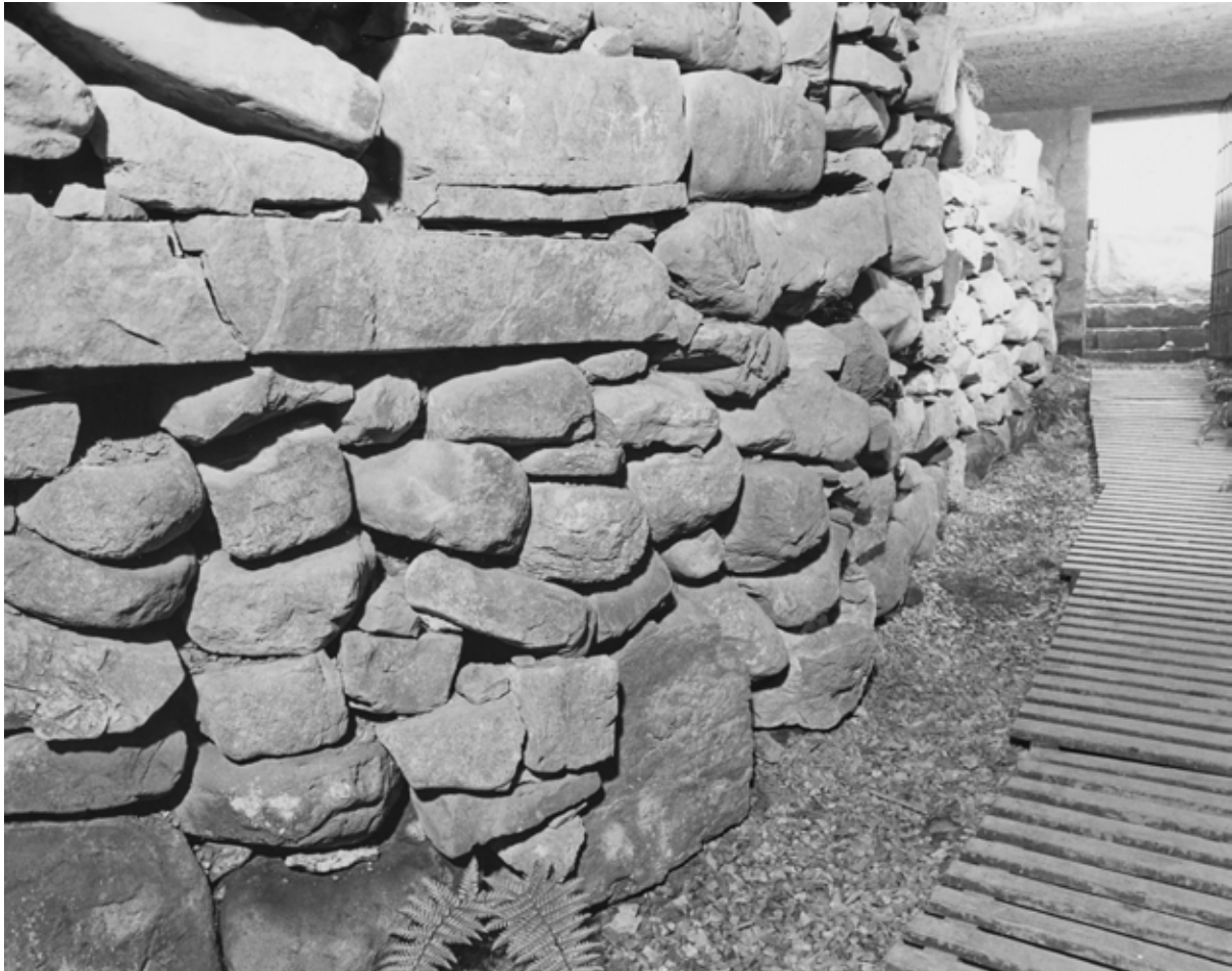
Figure 10: The walls of the souterrain are formed of boulders and quarried stone. Image taken 1975. © Historic Scotland.
