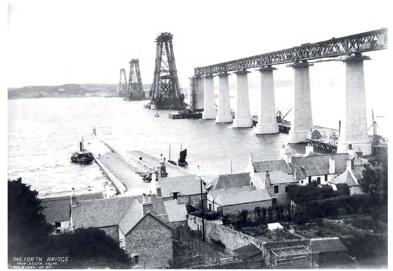
Progress photograph of the Forth Bridge from the south shore showing the south approach viaduct, Hawes Pier and surrounding buildings, 9 Aug 1887. (© Crown Copyright, National Records of Scotland, BR/ FOR/4/34/395, Evelyn Carey, AAA01539)
