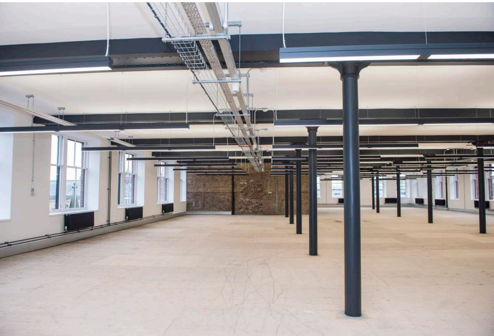
Below: Example of floor of the Garment Factory after refurbishment ©Morgan McDonnell Architecture
