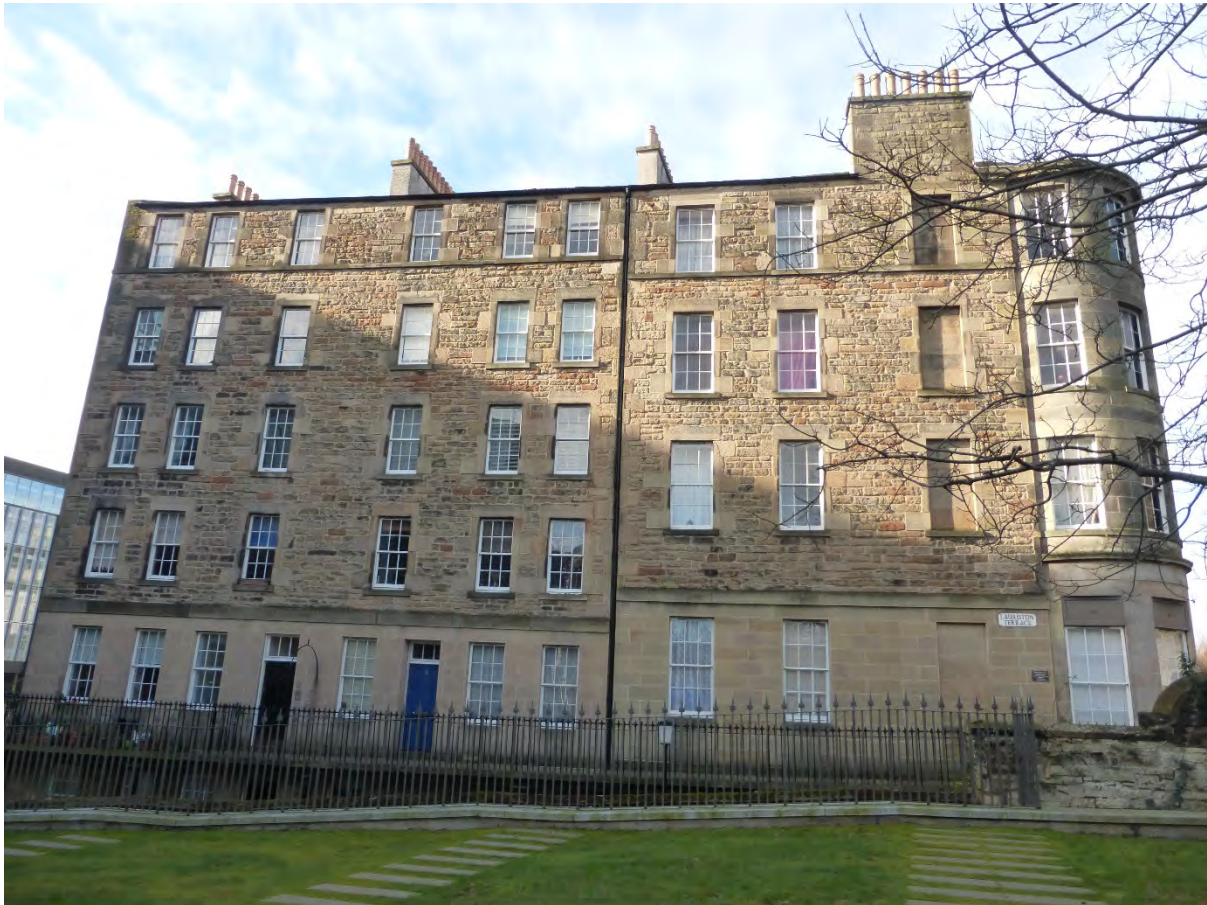
Figure 1: Front elevation of Lauriston Terrace. The flats where work was carried out are the farthest tenements on the left.
