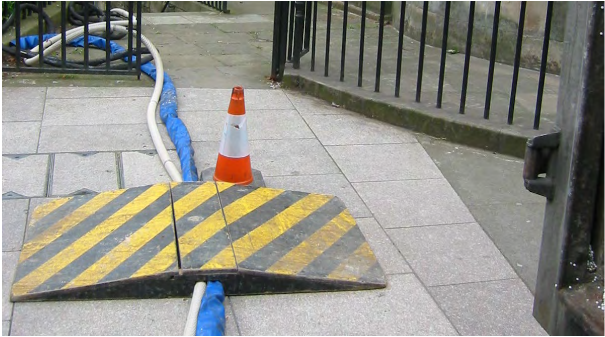
Figure 6. The pipes for the insulation crossing the pavement into Lauriston Terrace.
