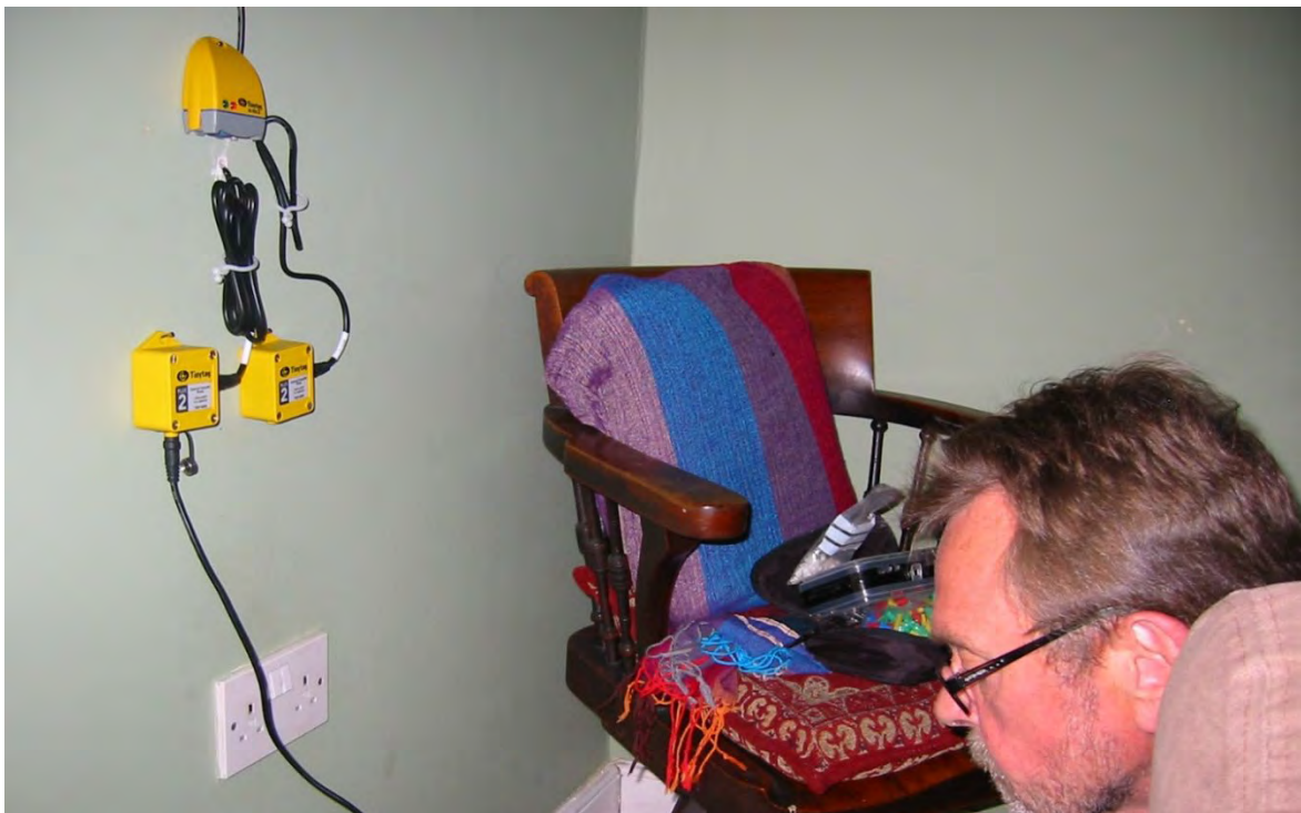
Figure 4. Installation of one of the humidity and temperature sensors.
