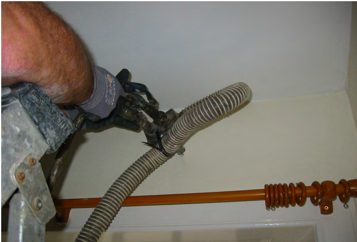
Figure 5. Blowing in the insulation.
