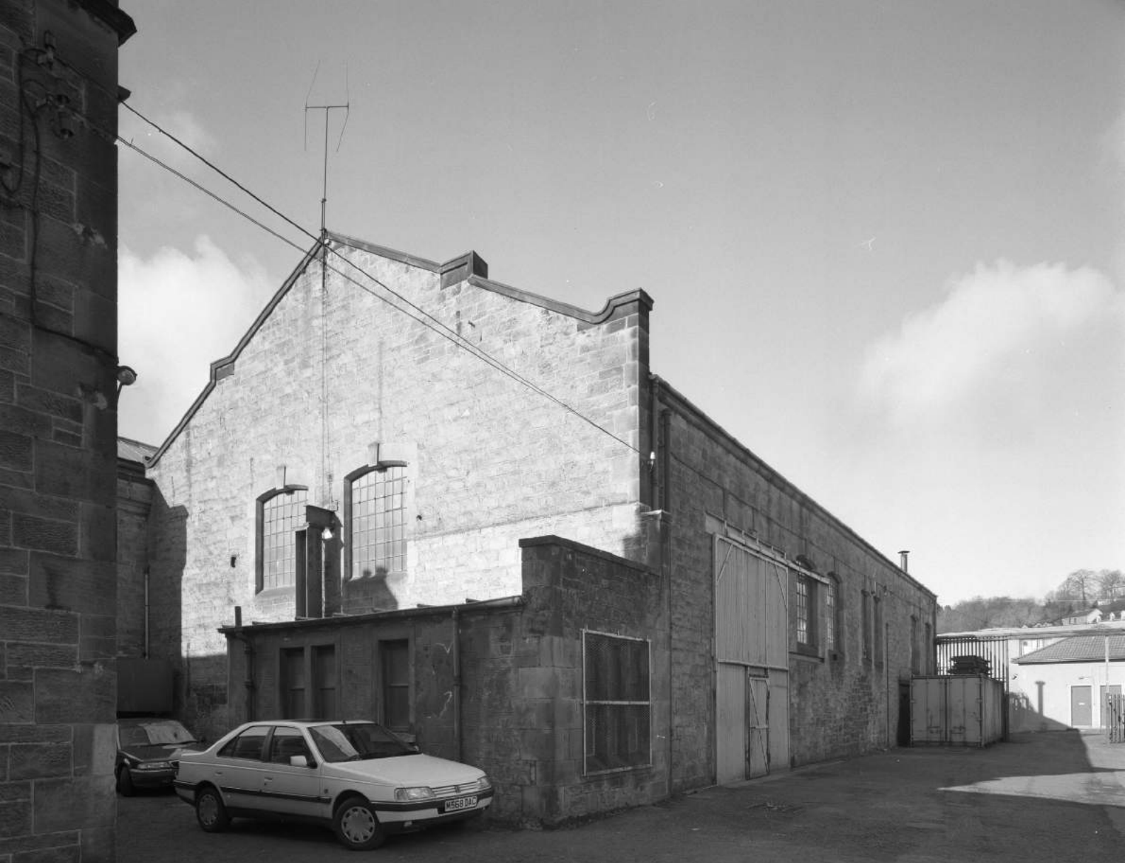
Above: View of the side elevation (North) of the former Hawick Urban Electric Company
